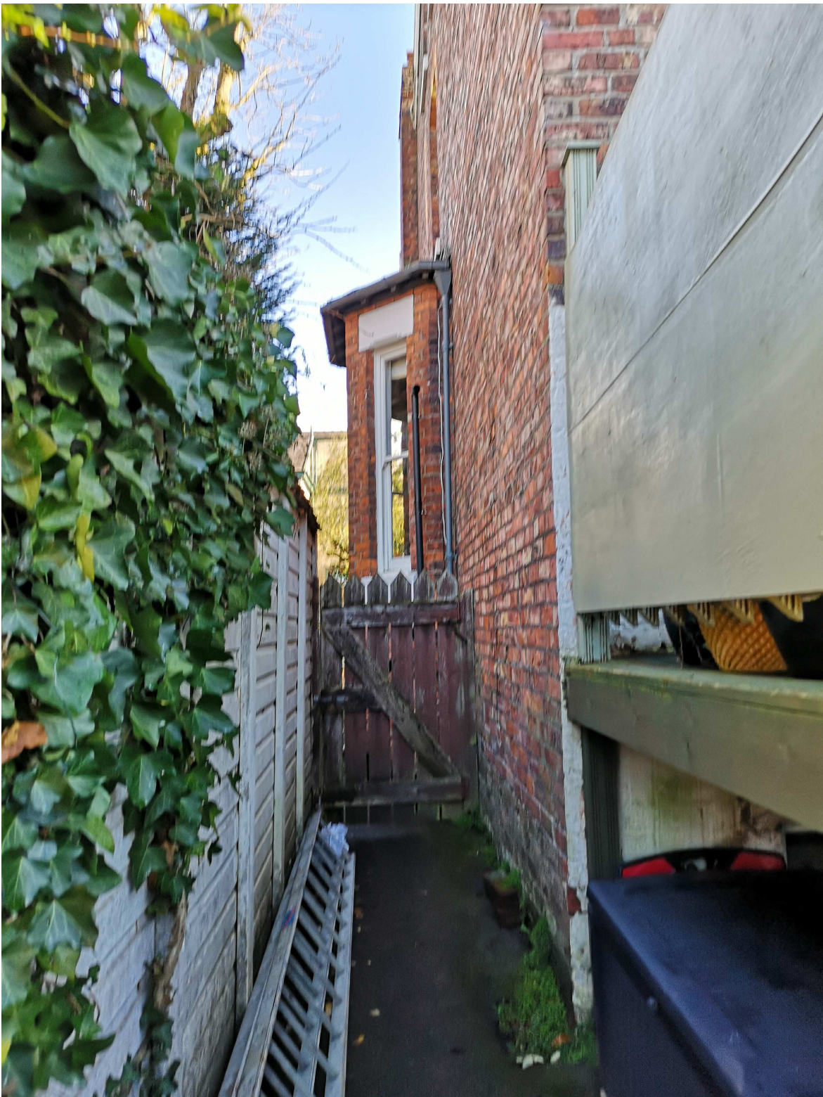
03 EXISTING SIDE ACCESS
