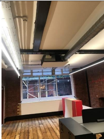
11) Existing interior – reception area – note modern plasterboard ceiling and associated rafts
