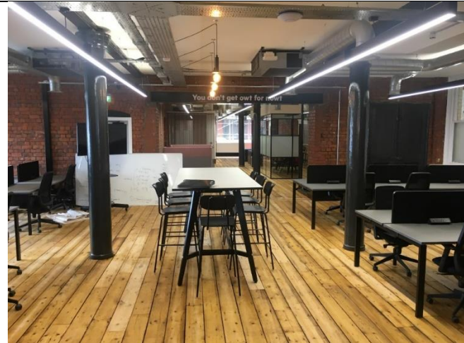
5) Existing interior – note new plasterboard ceiling (white) and hung rafts/ M&E and lighting
