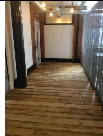
8) Existing interior – note new doors and plasterboard finishes
