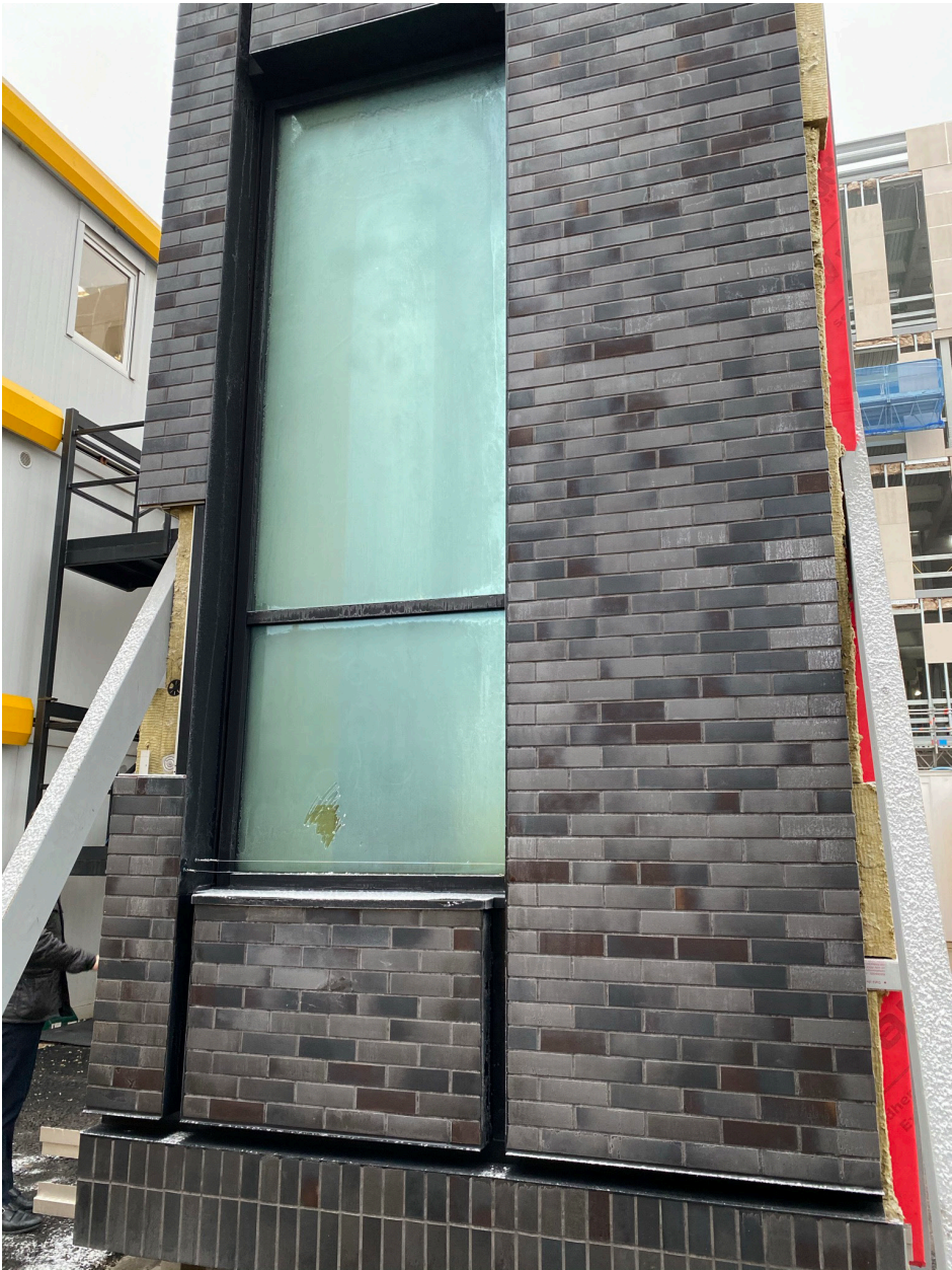
Window cw fritted strip (photo taken on frosty day and frit not clearly apparent)
