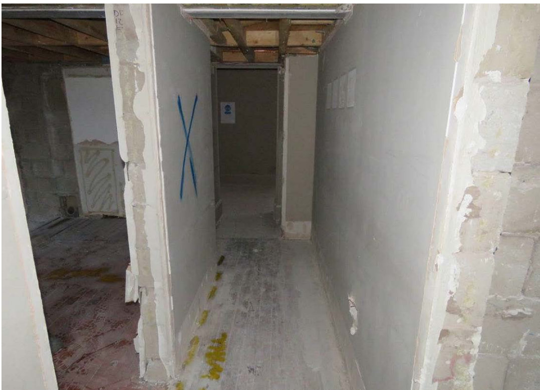
Figure 81: Looking north across F10, which originally formed part of a girls' classroom.
