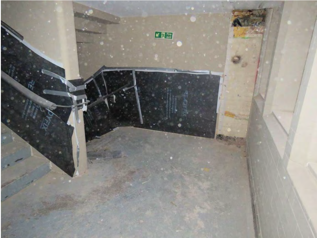
Figure 75: Looking south across the original boys' staircase (GM14). The glazed brick/exposed red brick will have its modern paint layers removed as part of the consented scheme.
