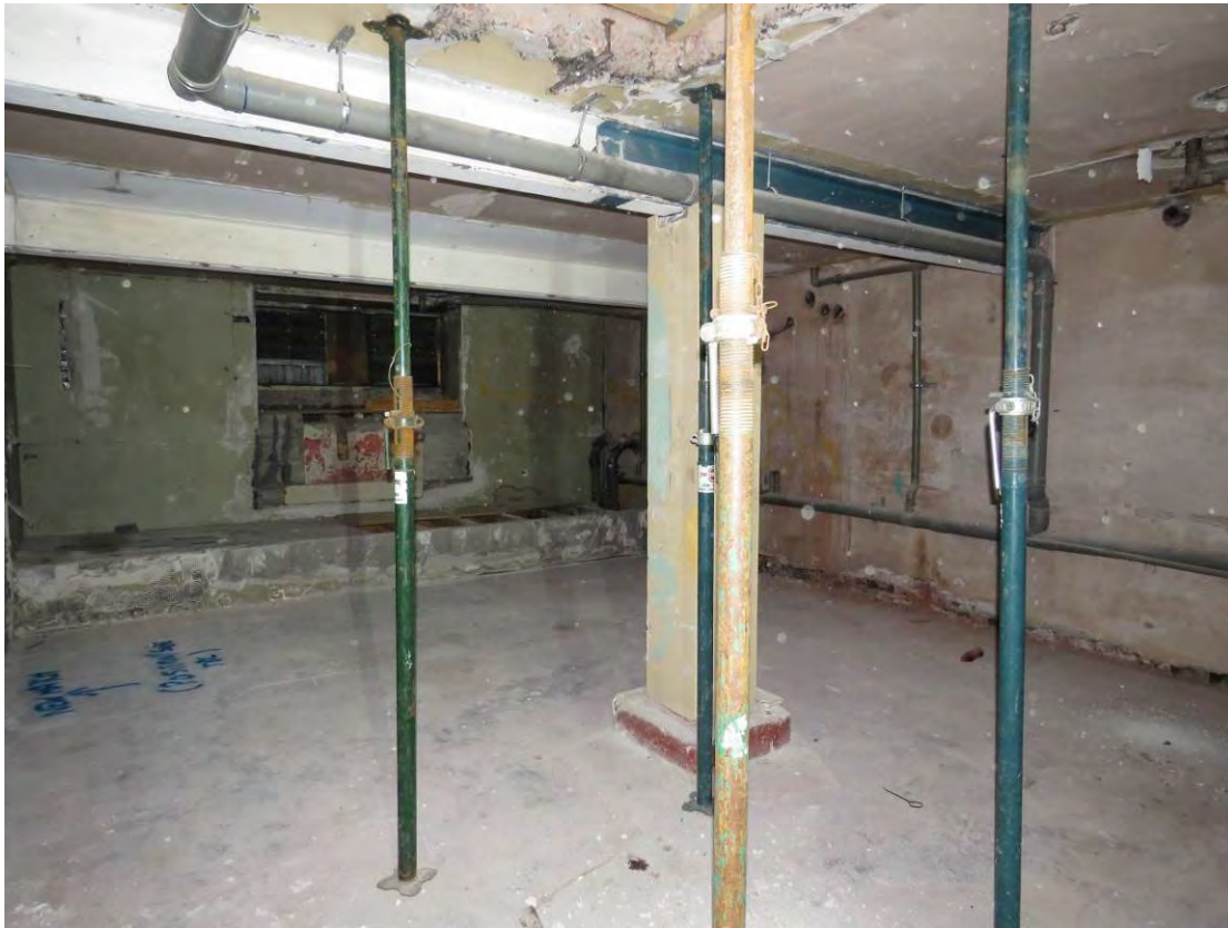
Figure 31: Looking north-east across the original store room (B5) showing a later central column.
