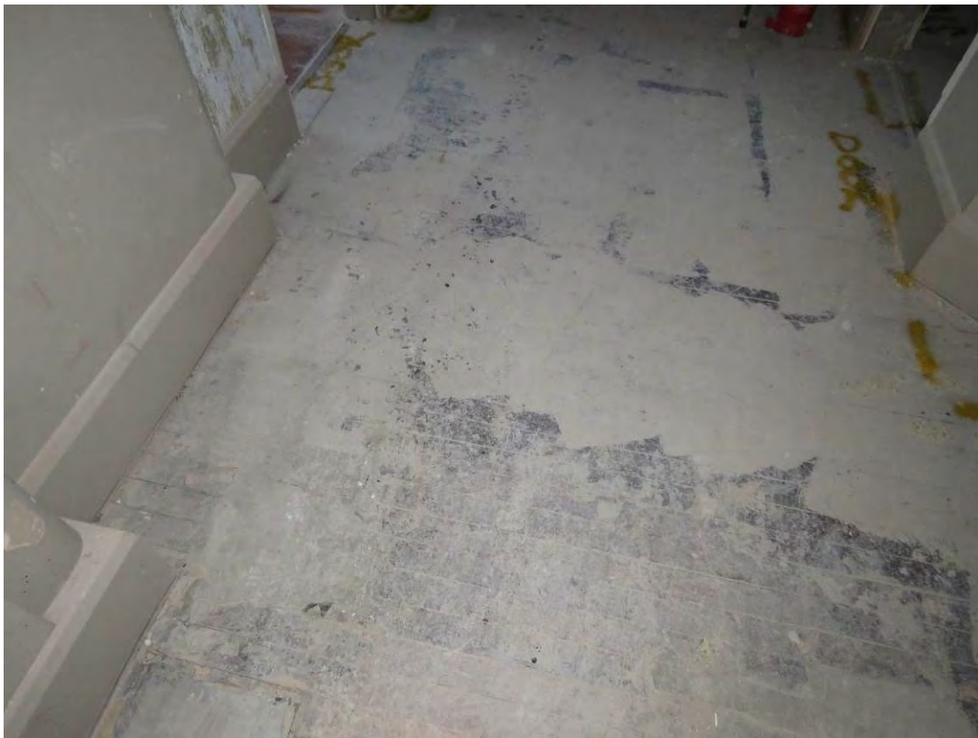
Figure 86: A detailed view of the surviving original timber floorboards to the former girls' school hall (F13), which will be re-covered as part of the consented scheme.
