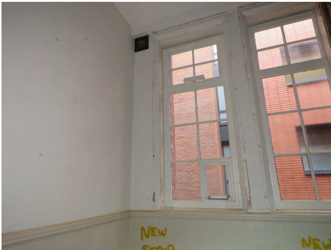
Figure 96: An example of an original/early metal vent to the left of the window in F24, which will be retained and redecorated as part of the consented scheme.
