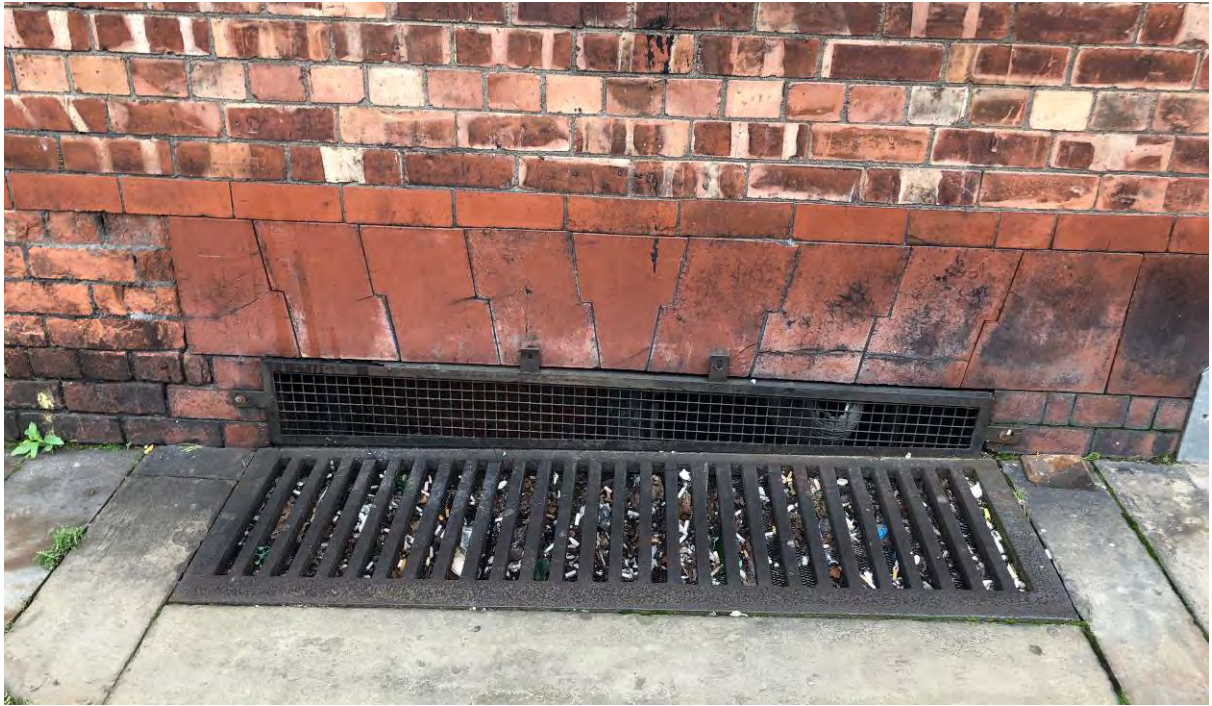
Figure 23: One of the two original basement windows/iron grills to the western corner of the south elevation, designed to light the original basement kitchen. The original grills will be retained and redecorated.
