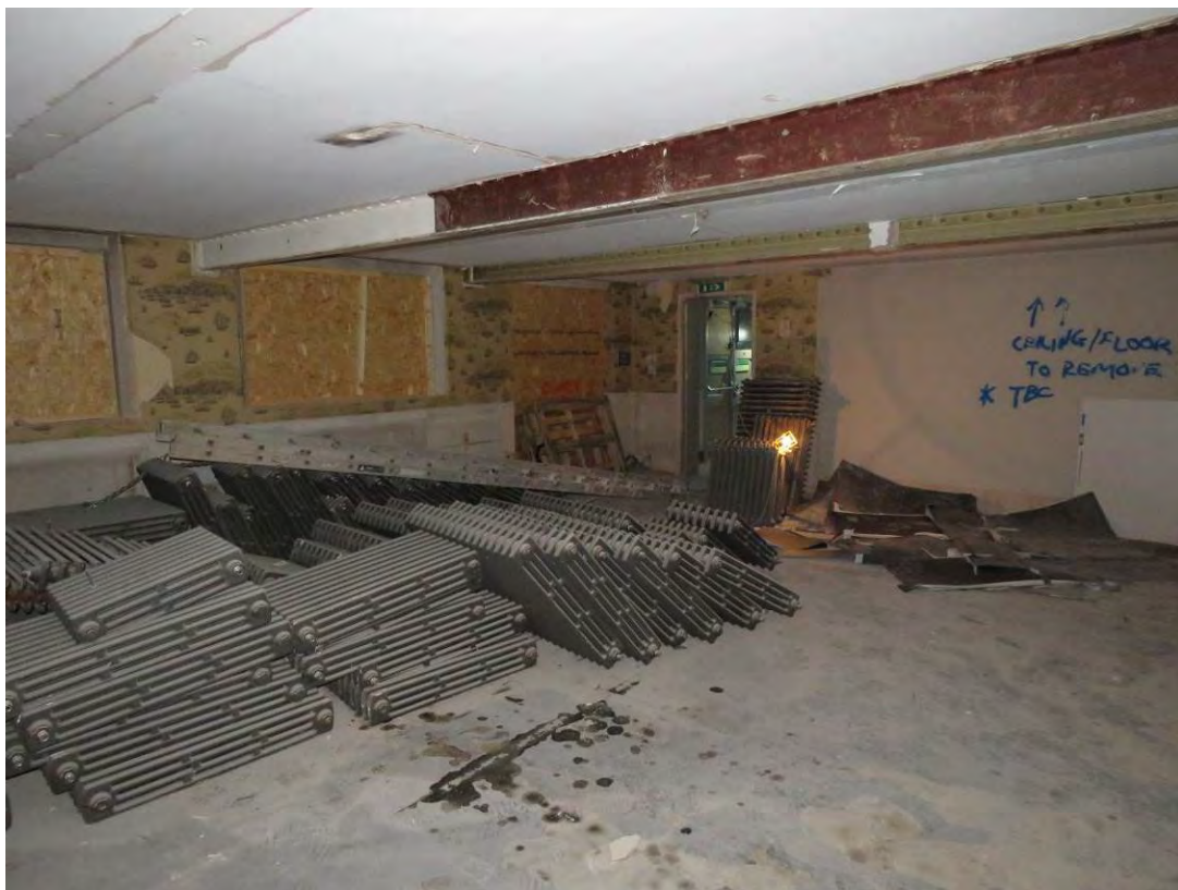
Figure 63: Looking south-east across G23, which formed the original infants' cloakroom, principal teacher's office and toilet, which have all been since removed.
