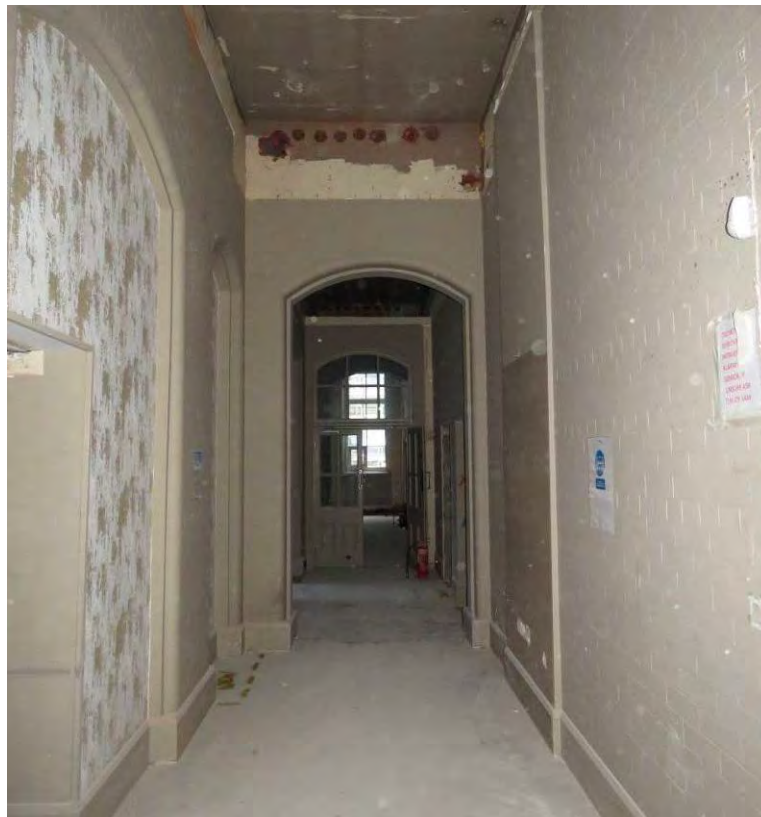
Figure 84: Looking west along F13, which formed the original girls' corridor. The now painted original glazed brick/exposed red brick will have its modern paint layers removed as part of the consented scheme.
