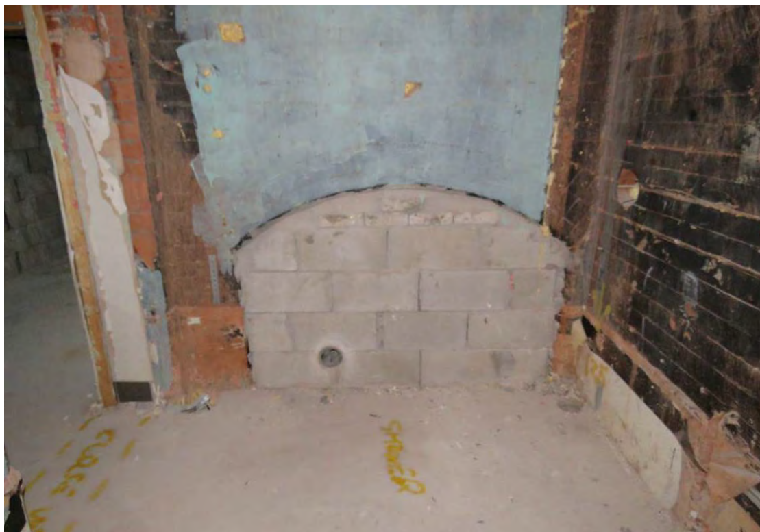
Figure 70: Looking west across the modern 2004 mezzanine level of GM7, which originally formed the upper part of the below infants' corridor (G16). The arched opening led into the infants' hall. The arch will be re-covered as part of the consented scheme.
