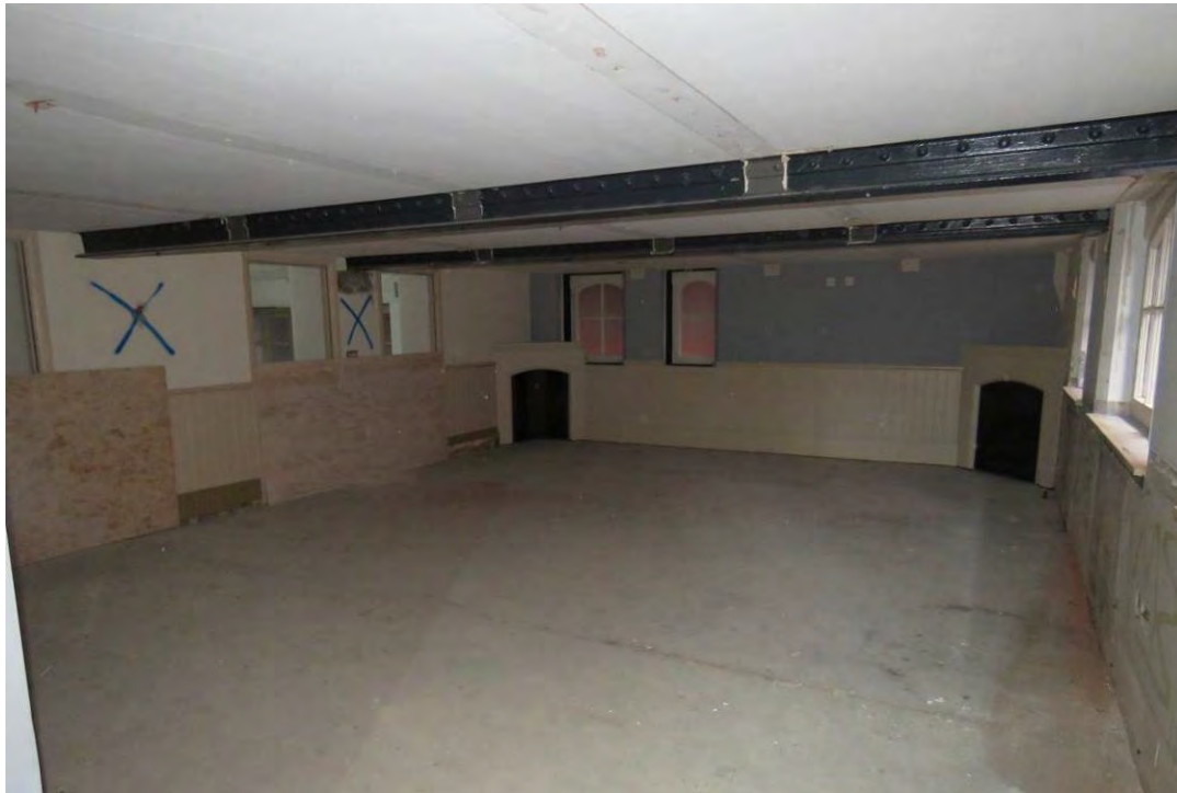
Figure 73: Looking north across the original ground floor mezzanine level (GM13), which originally contained a corridor and two teacher's offices (left and right), divided by glazed timber screens (now removed) and each containing a corner fireplace. The two fireplaces will be retained and redecorated as part of the consented scheme.
