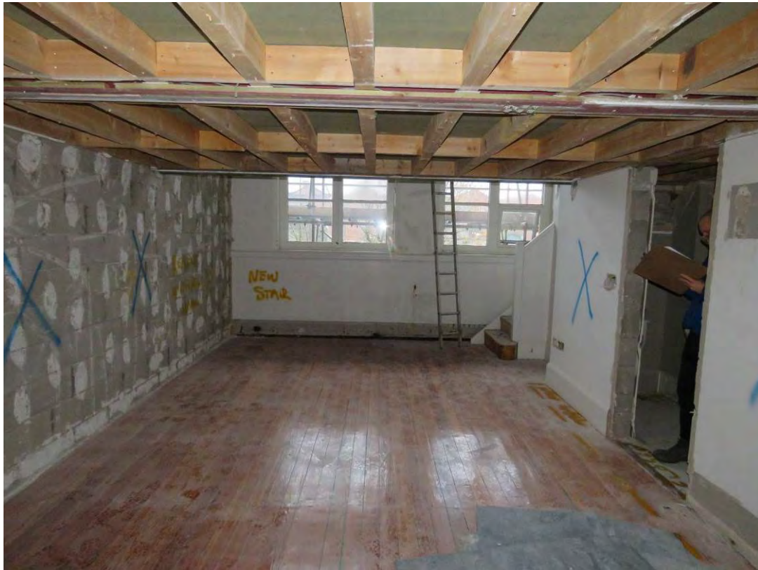
Figure 79: Looking south across F2, showing an example of original timber floorboards, which will be covered with new timber floor as part of the consented scheme.
