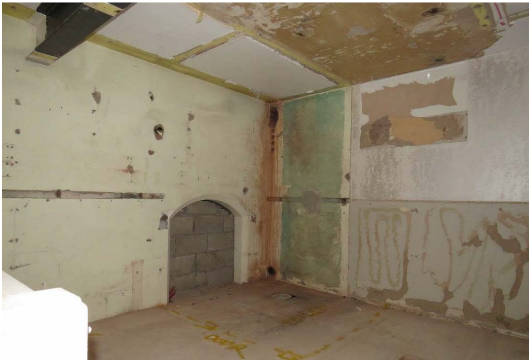
Figure 105: Looking south-east across FM9 which originally formed the upper part of the first floor girls' classroom. The blocked arched opening forms the upper part of the original girls' classroom entrance door. The blocked arch will be re-covered as part of the consented scheme.
