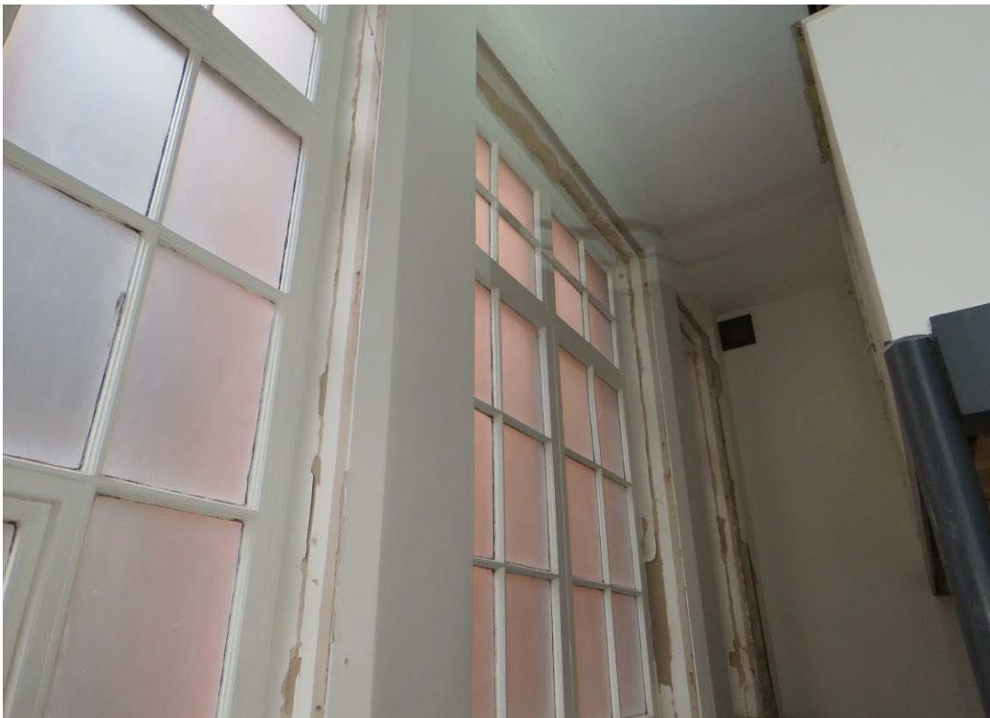
Figure 100: Looking north-east across F25, which originally formed a girls' classroom. An original/early metal ventilation grill can be seen to the right of the right-hand window, which will be retained and redecorated as part of the consented scheme.
