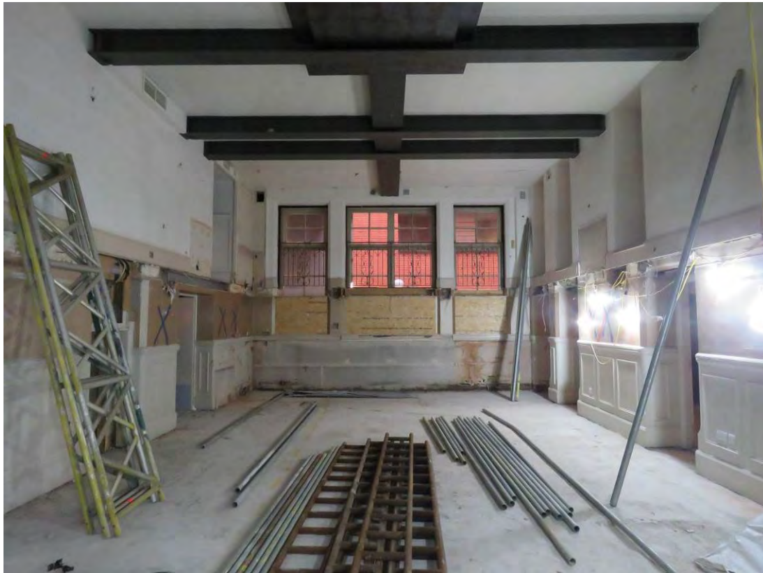
Figure 60: Looking north into the original infants' school hall (G21), showing areas of surviving timber dado rail, which will be retained and concealed from view as part of the consented scheme.
