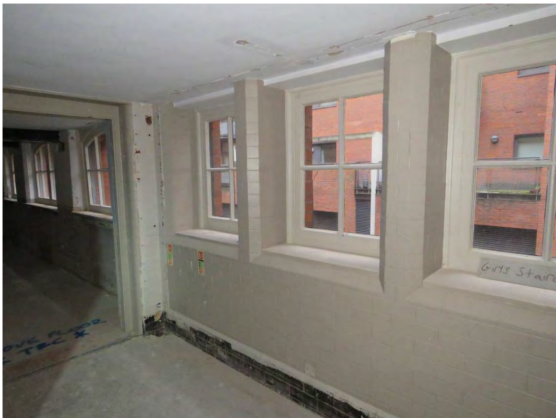
Figure 72: Looking north across the original mezzanine landing of GM12, which formed the original girls' staircase. The glazed brick/ exposed red brick will have its modern paint removed as part of the consented scheme.
