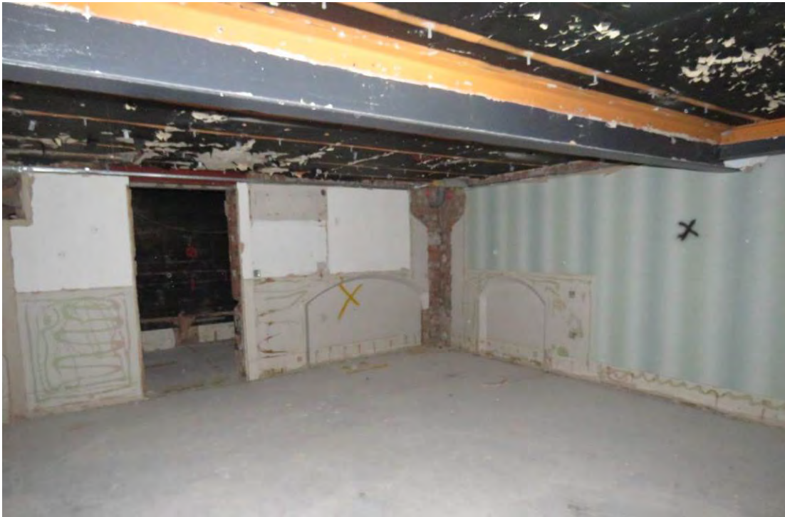
Figure 69: Looking north-east across the modern 2004 mezzanine level of GM6, which originally formed the upper part of the below infants' classroom (G9/10). Although the arched opening to the right does not appear on the original plans, it is original and would have linked two of the classrooms. The arches will be re-covered as part of the consented scheme.
