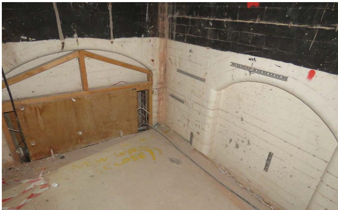
Figure 66: Looking north-west across the modern 2004 mezzanine level of GM2, which originally formed the upper part of the below infants' entrance corridor (G18). The arch to the left forms the original boys' entrance porch doors, whilst the arch to the right forms the upper part of the original boys' staircase entrance. The arches will be re-covered as part of the consented scheme.
