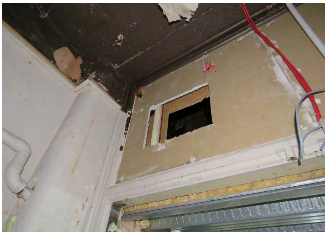
Figure 52: Looking west into the original main infants' corridor (G16) from entrance porch (G15), illustrating the modern 2004 mezzanine floor above.
