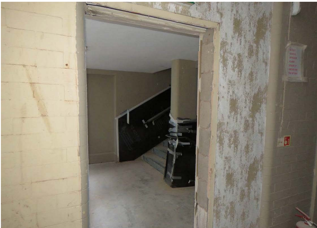
Figure 88: Looking into the former boys' staircase (F18) from F14. The now painted original glazed brick/exposed red brick to the staircase walls will have its modern paint layers removed as part of the consented scheme.
