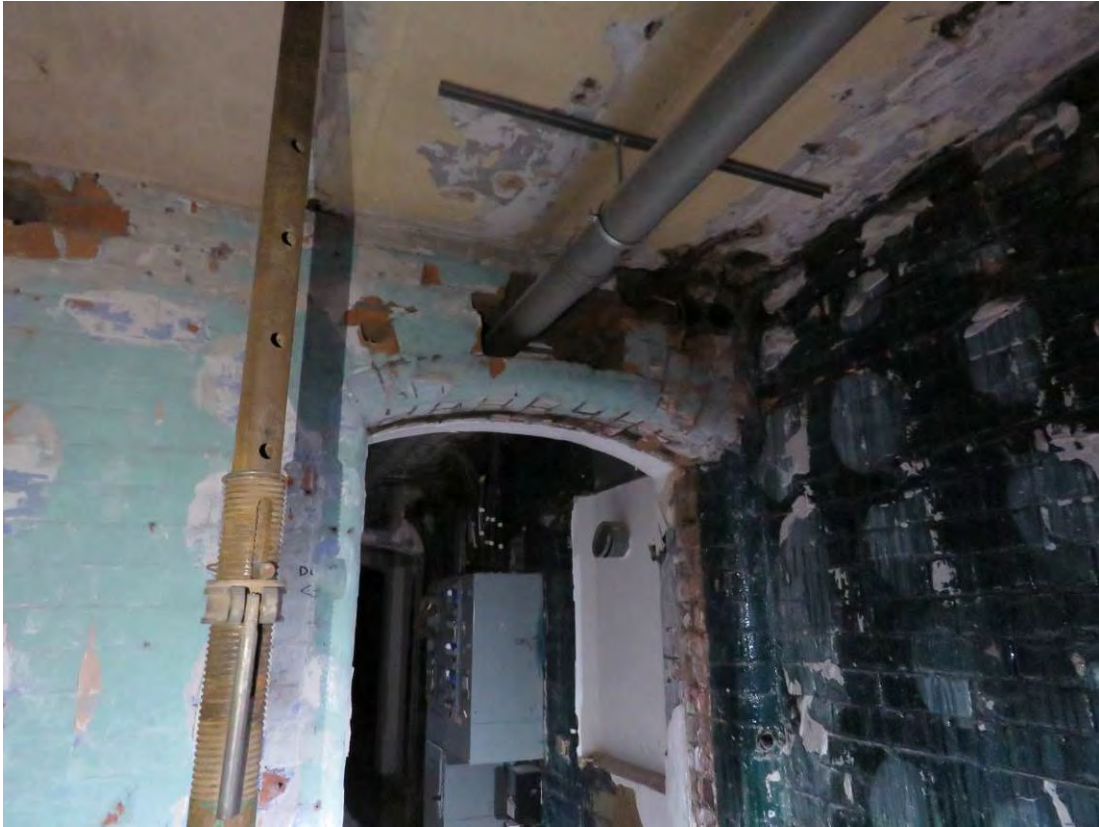
Figure 33: The original segmental arched storeroom door opening (B5).
