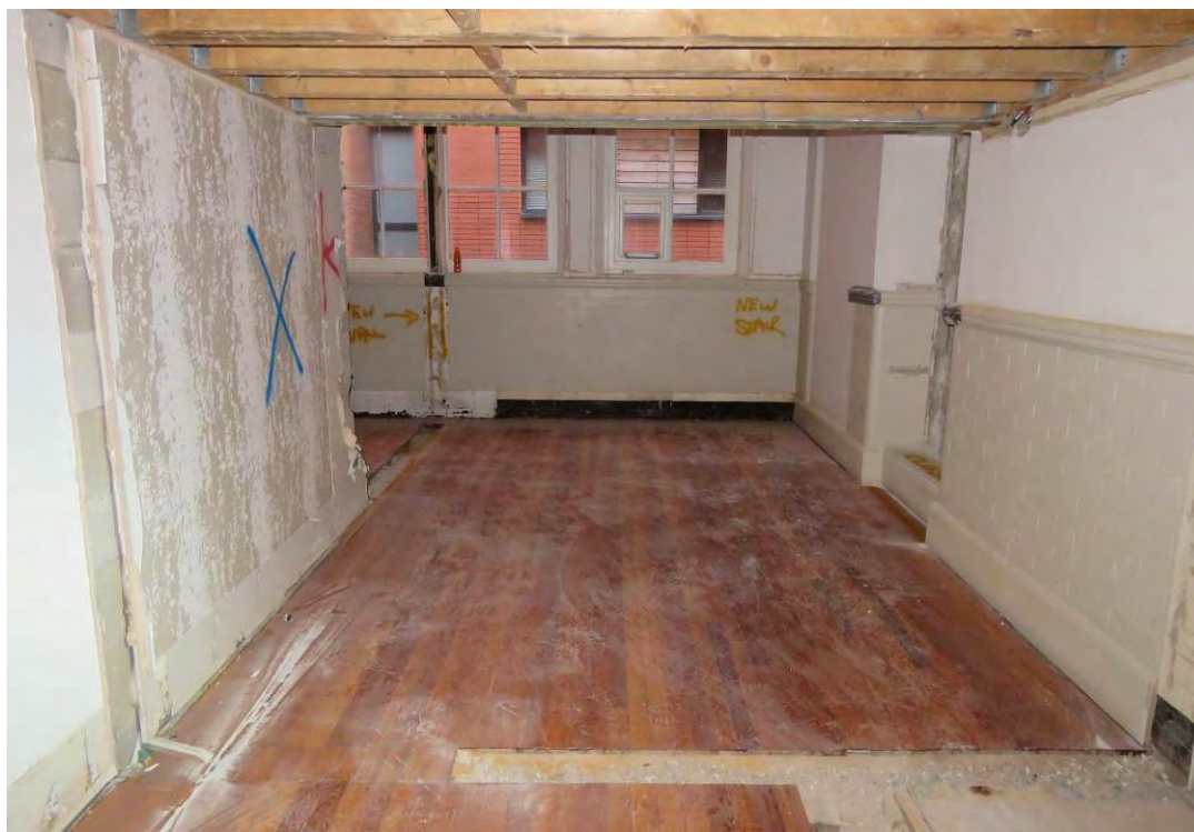
Figure 93: Looking north from F27 into F26, which together with the adjacent rooms originally formed the girls' hall. Beneath the right-hand window can be seen the original brown glazed brick, which acted as a skirting. The timber dado rails are original and will be retained and redecorated. The timber floorboards are original and will be covered with new timber flooring as part of the consented scheme.
