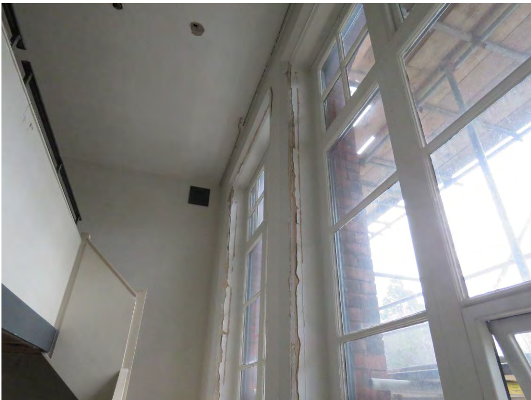
Figure 82a: Looking east across F11 towards an original/early metal ventilation grill, which will be retained and redecorated as part of the consented scheme.
