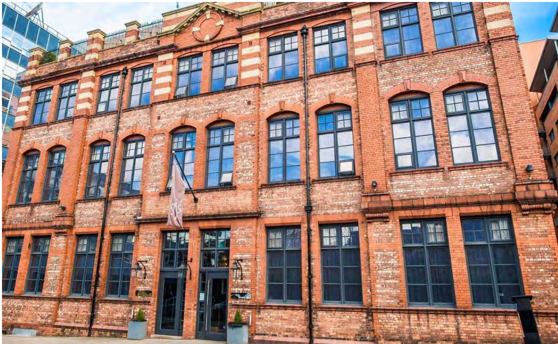
Figure 1: The principal south front of the Great John Street Hotel.
