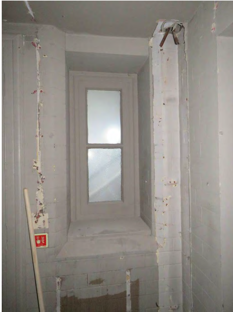
Figure 57: One of the two original boys' entrance windows to the north side of the entrance doors in G20.
