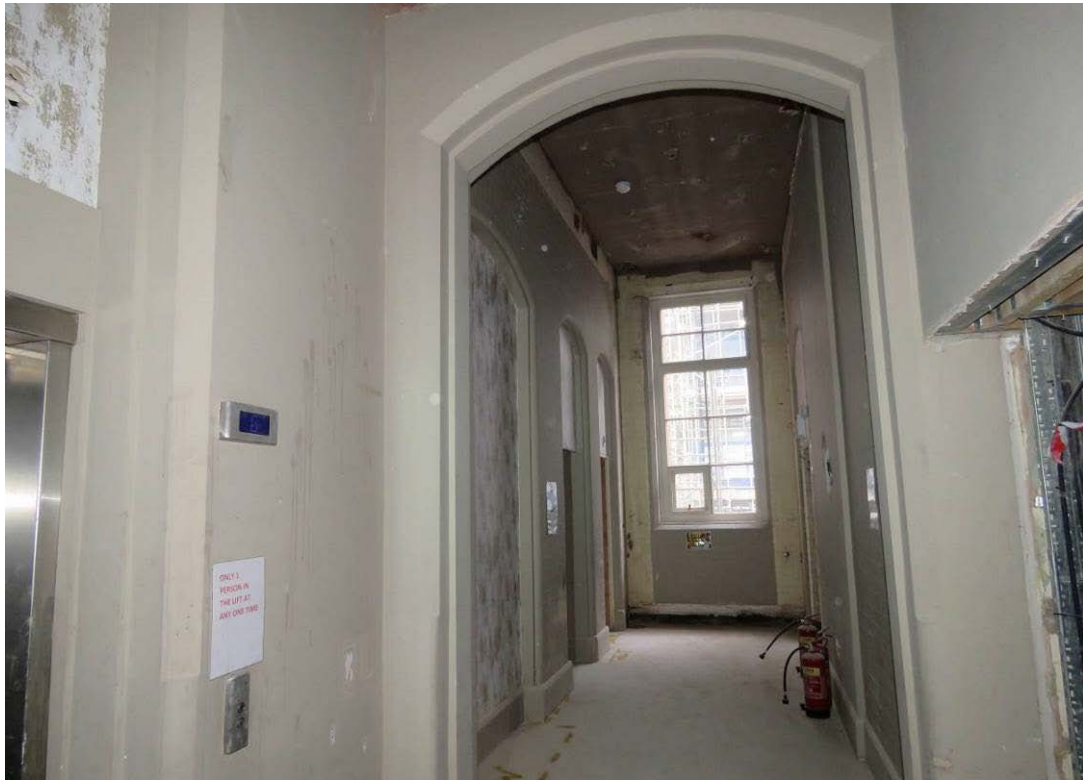
Figure 85: Looking west along F14, which formed the original girls' corridor. The now painted original glazed brick/exposed red brick will have its modern paint layers removed as part of the consented scheme.
