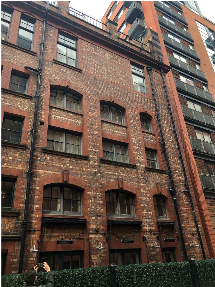
Figure 29: The northern half of the east elevation on Little John Street. The window arrangement denotes the two original mezzanine floor levels to this part of the building.
