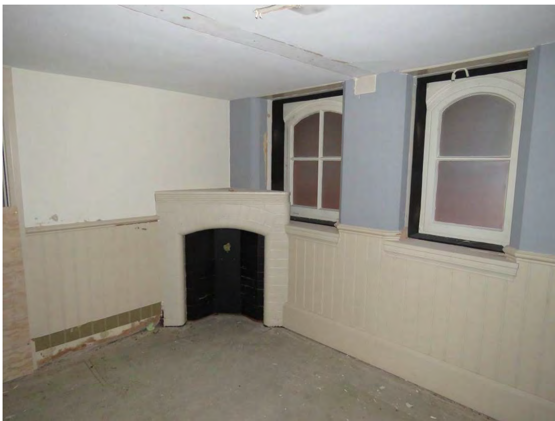
Figure 74: A detailed view of the original glazed brick corner fireplace to the original north-east teacher's office in GM13. This fireplace will be retained as part of the consented scheme.
