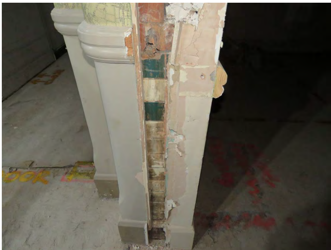
Figure 50: A detailed view of the original door opening between G14 (right) and G16 (left), illustrating the surviving original green and cream glazed brick which originally lined each of the classroom dado levels (now covered). This area of exposed brick will be re-covered with the insertion of a new door.
