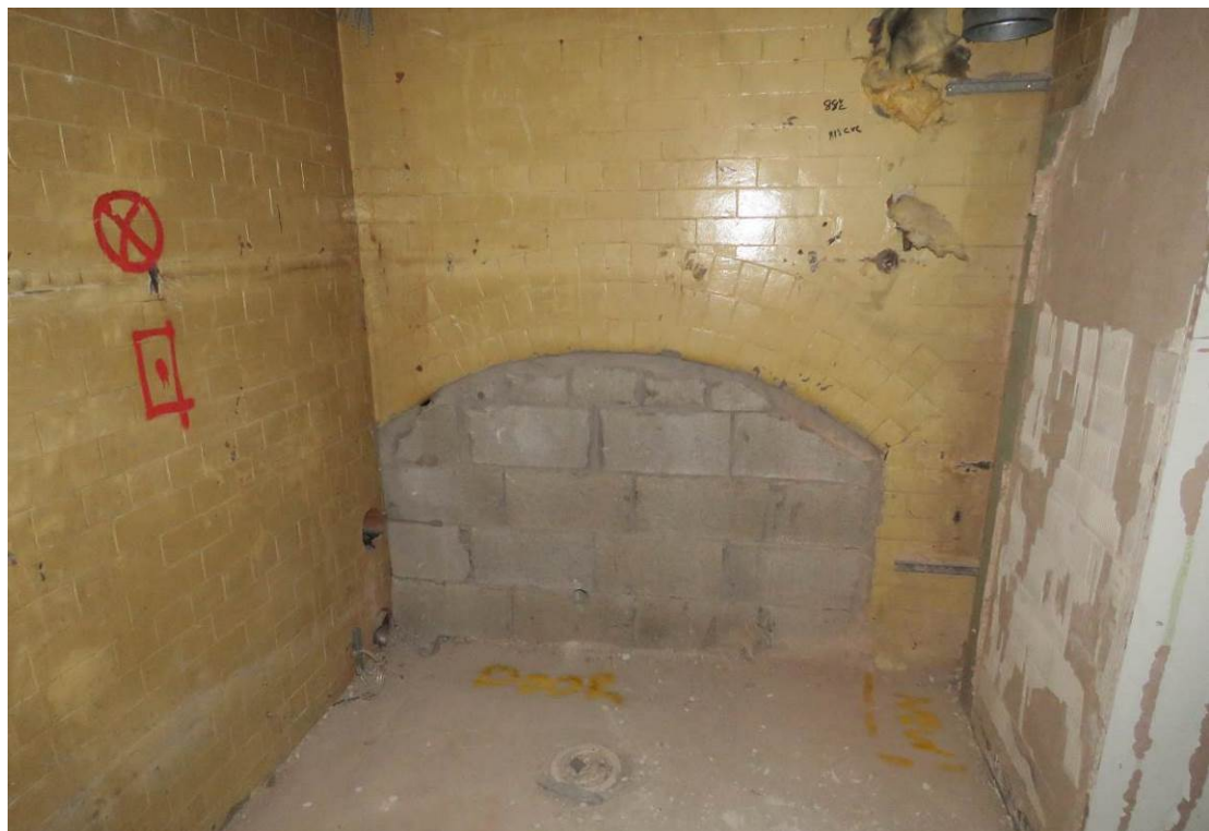
Figure 68: Looking north-east across the modern 2004 mezzanine level of GM3, which originally formed the upper part of the below infants' corridor (G18). The arched opening originally led into the infants' hall (G21). The arch will be re-covered as part of the consented scheme.
