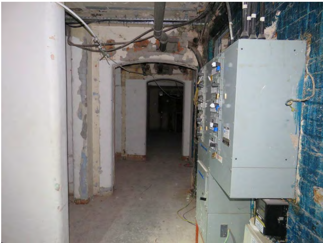
Figure 34: Looking north into the corridor (B4) from the former storeroom (B5) towards the former kitchen (B1). The boys' staircase is concealed to the left.
