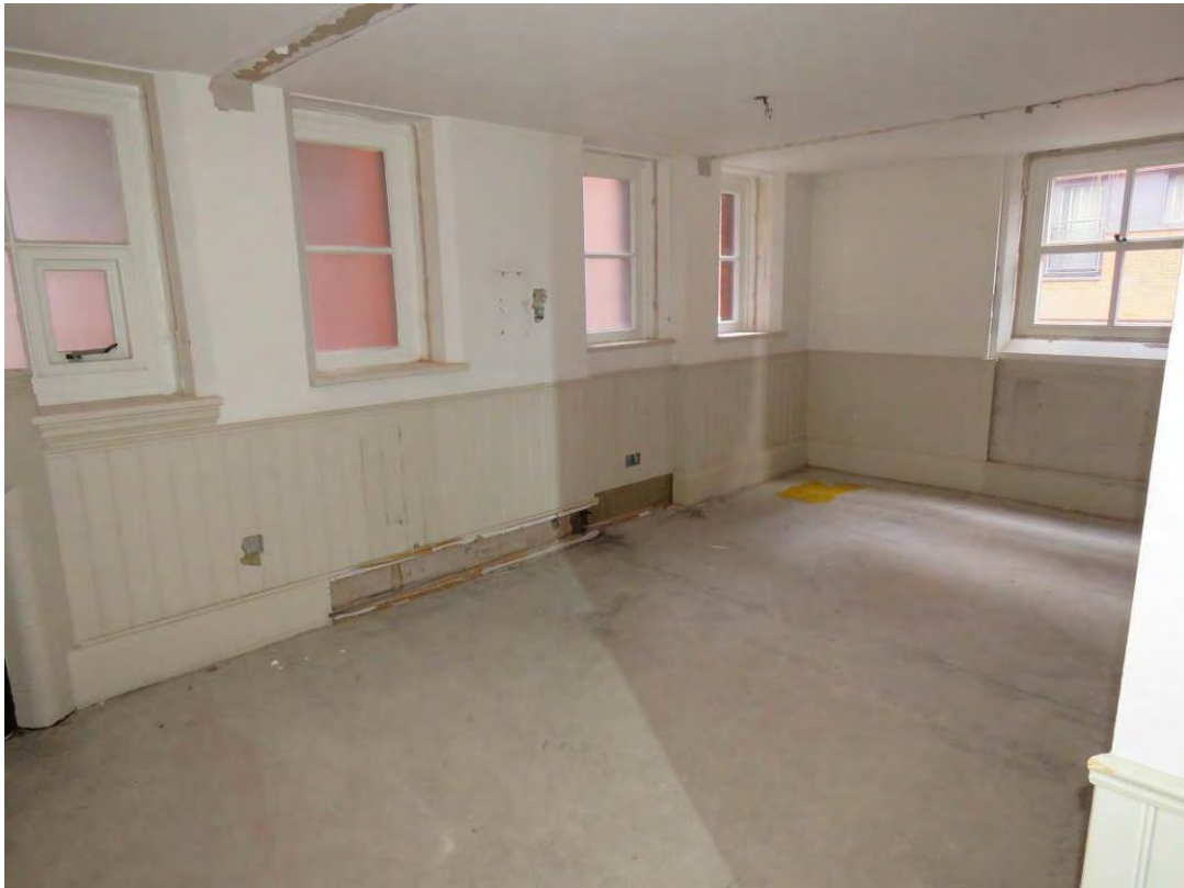
Figure 91: Looking north-east across F27a, which originally formed a teacher's office (left) and girls' toilet (right).
