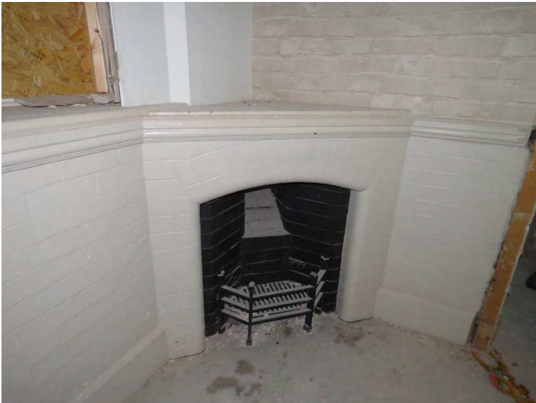
Figure 48: An original corner fireplace as seen in the south-west corner of G13, which originally formed a boys' classroom. This fireplace will be retained and redecorated as part of the consented scheme.
