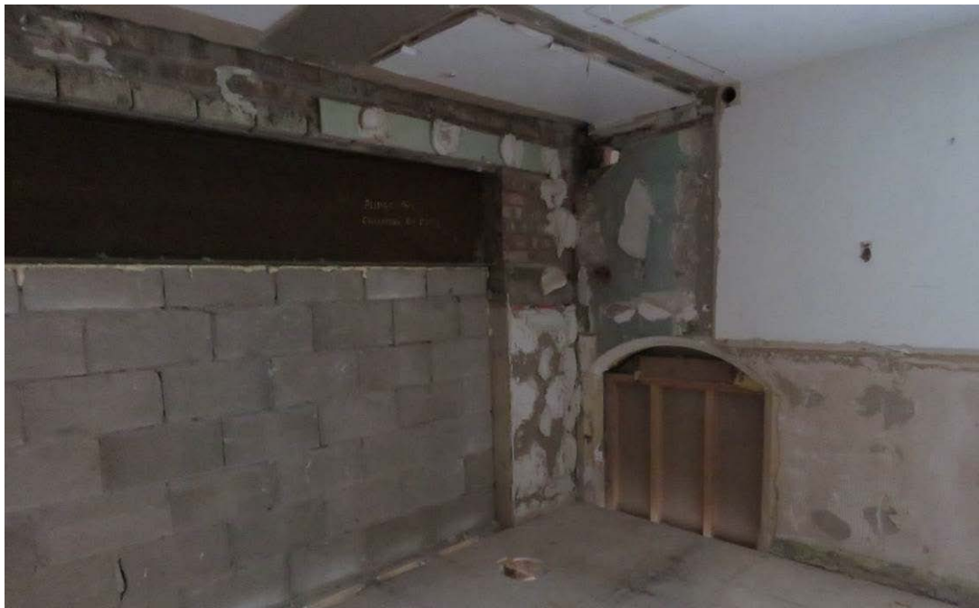
Figure 103: Looking north-west across FM7 which originally formed the upper part of the ground floor infants' classroom. The blocked arched opening forms the upper part of the original first floor girls' classroom entrance door. The blocked arch will be re-covered as part of the consented scheme.
