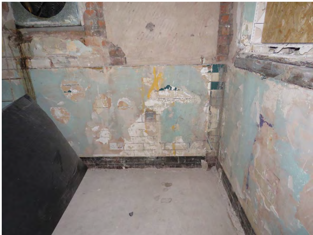
Figure 59: A detailed view of the partially plastered/ partially exposed original glazed brick to the north-west corner of the former hotel kitchen (G22). The plastered glazed brick walls will be re-covered as part of the consented scheme.
