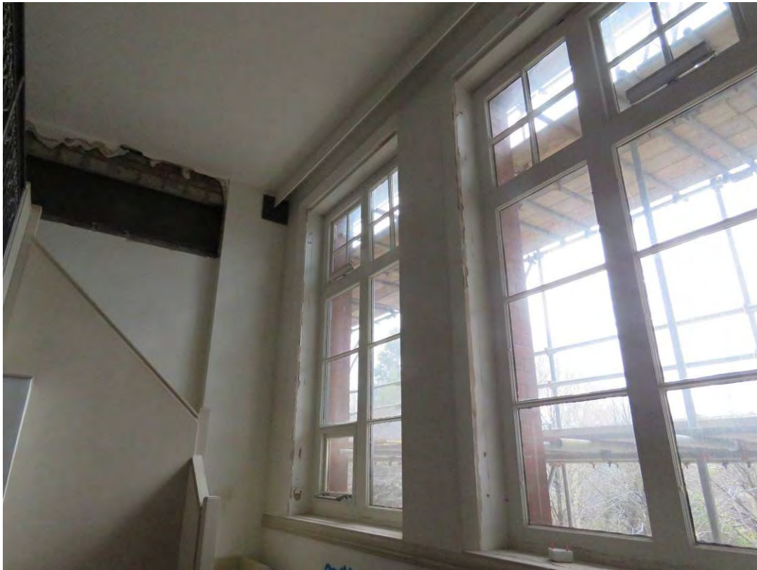
Figure 80: Looking east across F8 towards an original/early metal ventilation grill, which will be retained and redecorated as part of the consented scheme.
