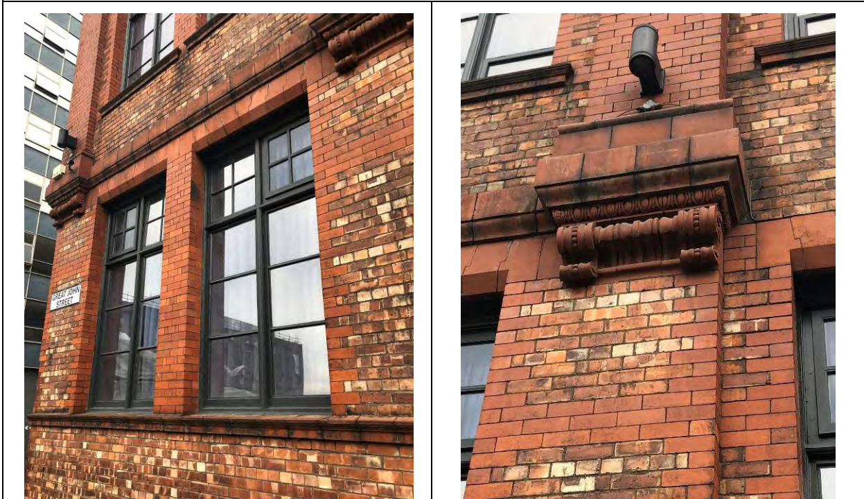
Figure 21: An example of the remaining original casement windows to the ground floor, Great John Street.
