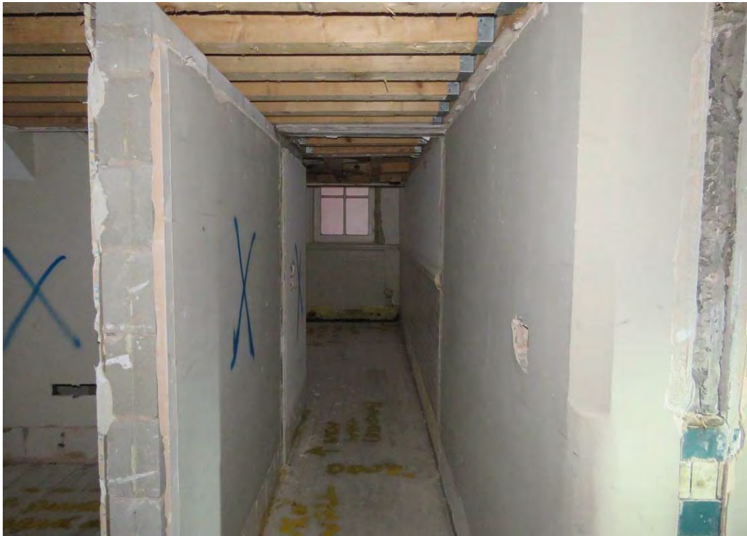
Figure 97: Looking north through F22 into F25, which together were originally a girls' classroom. Note the original plaster wall with splayed corner forming the original entrance door (right) and an area of exposed original green and cream glazed brick, which will be re-covered with the insertion of a new doorway.
