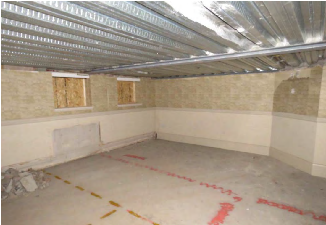
Figure 49: Looking south-east into G14, illustrating the modern 2004 mezzanine floor above and 2004 window openings onto Little John Street to the left. This room originally formed part of G13.
