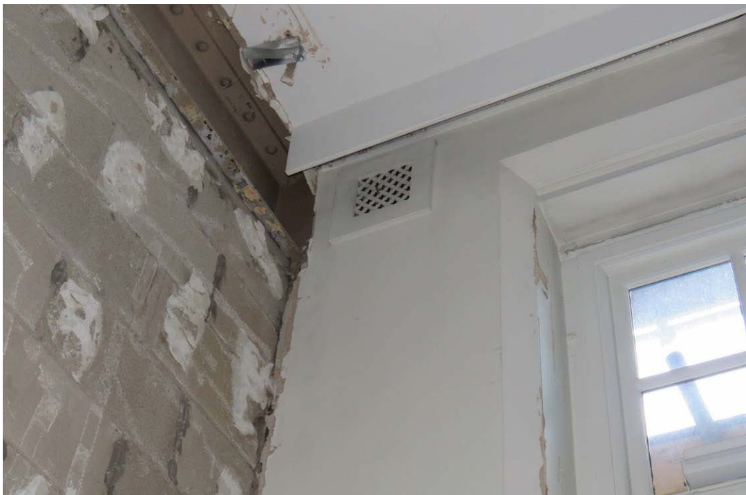
Figure 79a: An example of an original/early ventilation grill in the south-east corner of F2, which will be retained and redecorated as part of the consented scheme.
