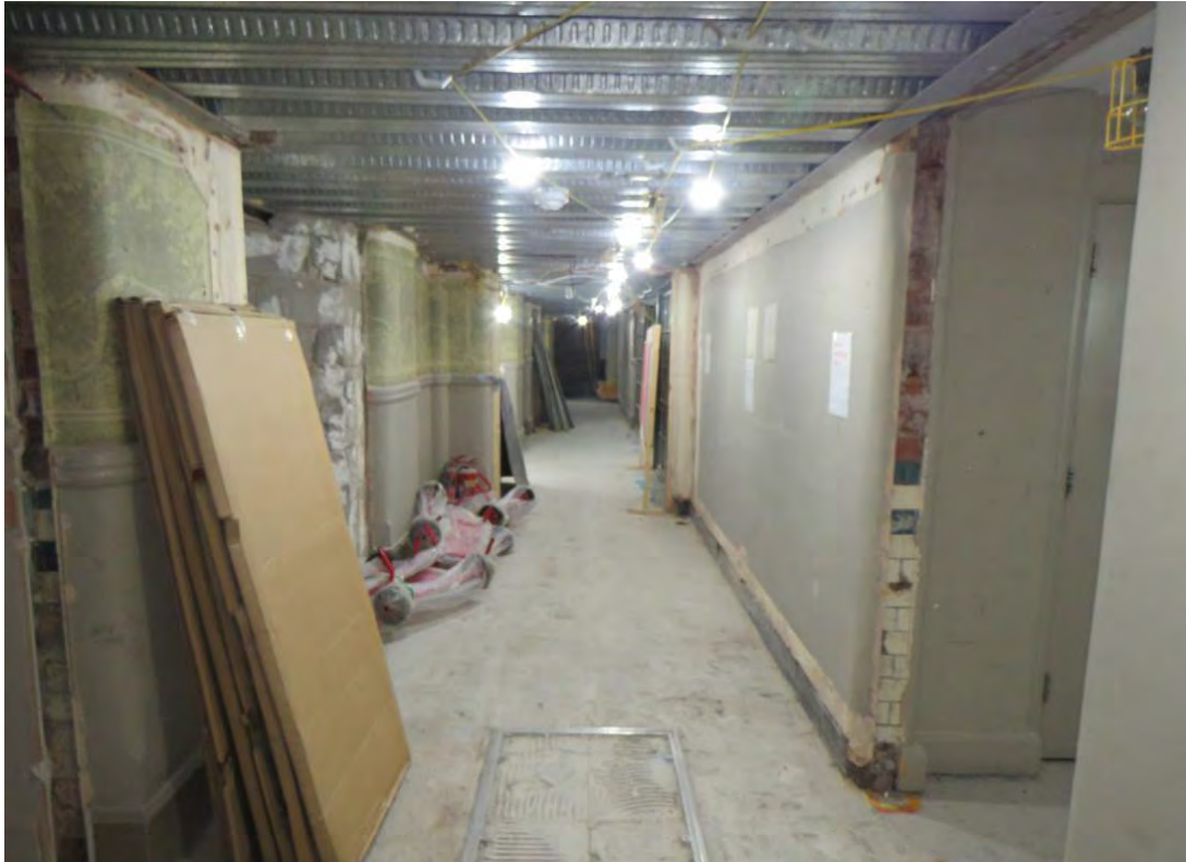
Figure 53: Looking west along the original infants' corridor (G16), showing the modern 2004 mezzanine ceiling. The exposed door jamb to the right shows an area of surviving glazed brickwork which will be re-covered with the insertion of new doors as part of the consented scheme. To the left can be seen remaining examples of original timber dado rail which will be retained and redecorated as part of the consented scheme.
