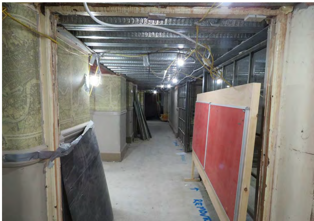
Figure 54: Looking further east along corridor G16, showing the modern glazed screen and doors which formed part of the 2004 hotel bar (right).
