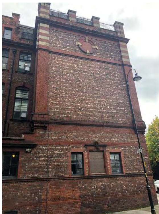
Figure 26: The southern end of the west elevation, showing the modern, inserted 2004 windows either side of the original plaque.
