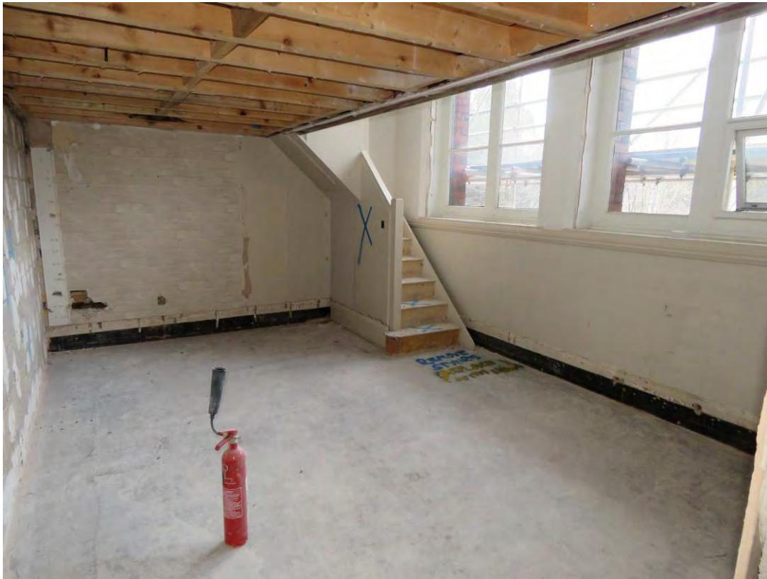
Figure 82: Looking south-east across F11, illustrating an example of a modern 2004 hotel mezzanine and stairs.
