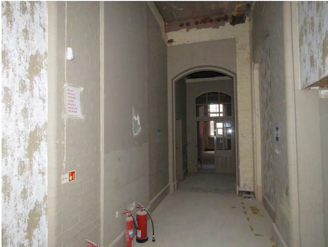
Figure 87: Looking east along the former girls' corridor (F14). The now painted original glazed brick/exposed red brick will have its modern paint layers removed as part of the consented scheme.
