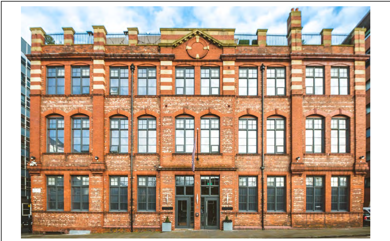
Figure 20: The principal south elevation fronting Great John Street.
