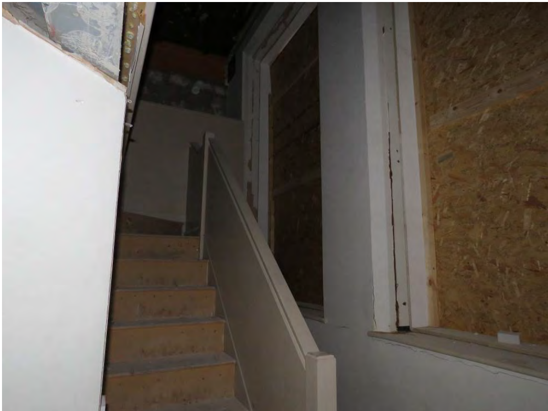
Figure 46: Looking east into G4, which originally formed part of a boys' classroom. The stairs and mezzanine were added in 2004.
