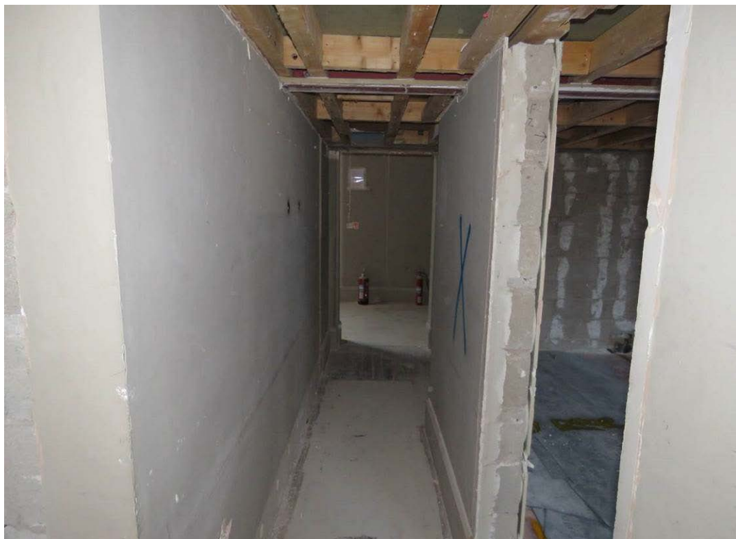
Figure 78: Looking north along F3 showing the modern 2004 walls (left) and mezzanine floor above.
