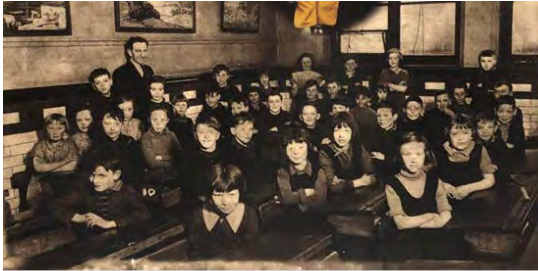
Figure 8: One of the classrooms during the 1930s, showing the original glazed brick to the dado level. Source: Great John Street Hotel archive. Source: Great John Street Hotel archive.
