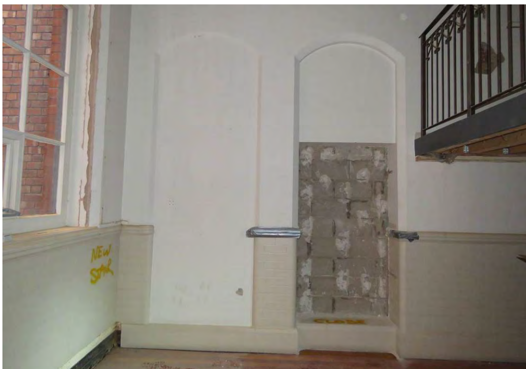
Figure 94: Looking east across the northern end of the former girls' hall (F26), showing the original surviving doorway into the teacher's office (left) and girls' cloakroom (right). Note the original glazed brick, which has since been overpainted and will remain painted. The original timber dado rail and plastered walls will be redecorated, whilst the two blocked archways will remain blocked and redecorated as part of the consented scheme.
