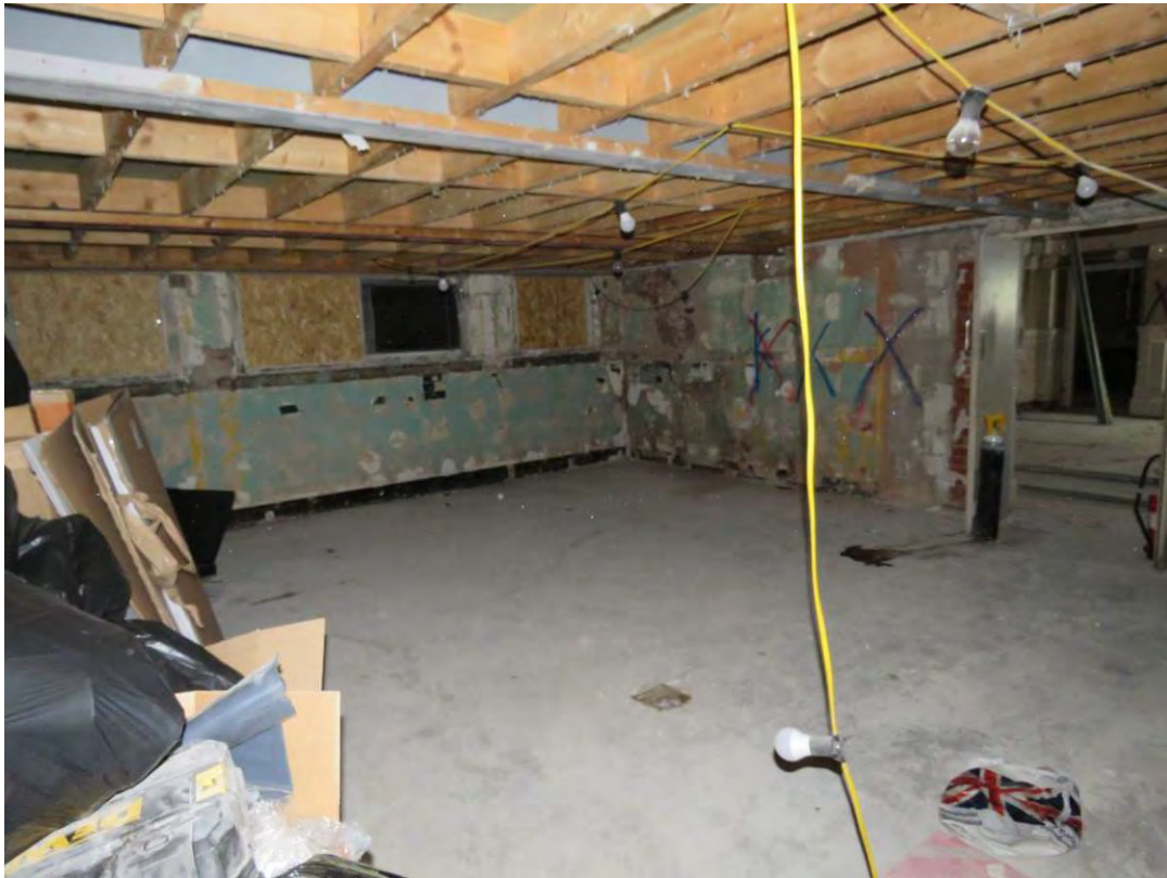
Figure 58: Looking north-east across a former boys' classroom (G22), which was converted to the hotel kitchen in 2004, including the insertion of a modern mezzanine floor above.
