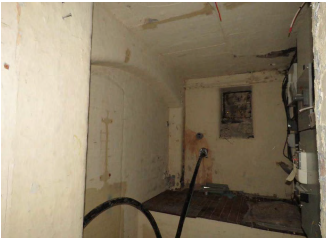
Figure 36: Looking into the original coal store (B2), showing the original surviving coal hatch, which leads up to Atherton Street. The blocked arched opening to the left appears to be original, and may have been a slight change to the original design of the basement. This doorway linked the coal store with the kitchen.
