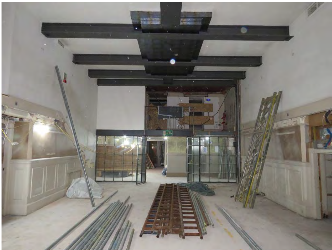
Figure 61: Looking south across G21 towards the modern 2004 hotel glazed screen.
