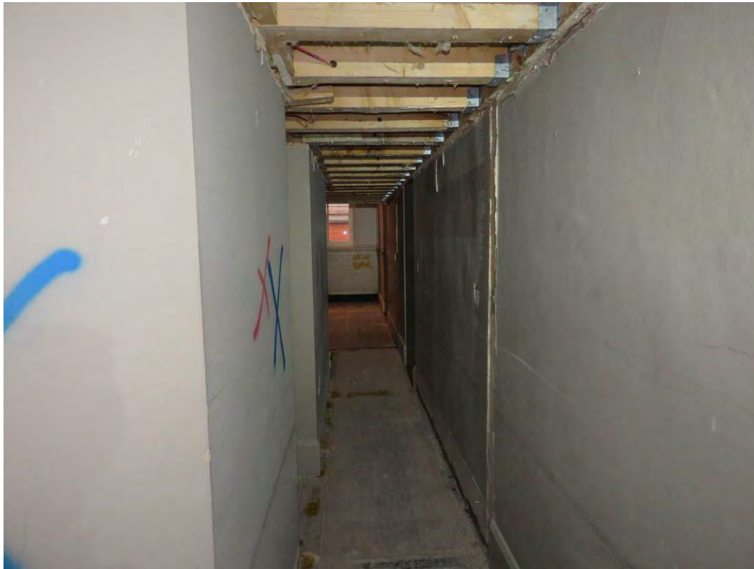
Figure 89: Looking north into F18, which originally formed part of the girls' school hall.
