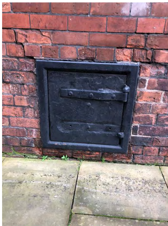
Figure 28: The original cast iron coal hatch below the boys' entrance window (Fig 27), which would have originally allowed coal to be delivered into the coal store at basement level. This hatch will be retained and redecorated.
