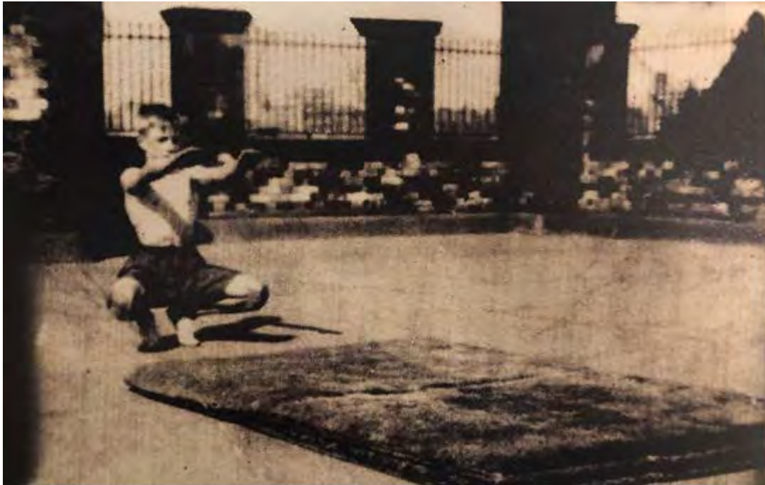
Figure 6: A school boy using the original roof top playground for exercise during the c1930s. Source: Great John Street Hotel archive.
