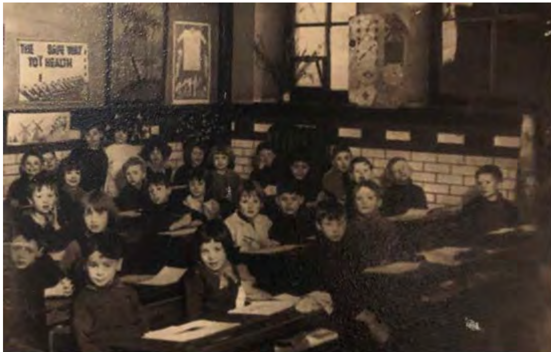
Figure 7: One of the classrooms during the 1930s, showing the original glazed brick to the dado level. Source: Great John Street Hotel archive.
