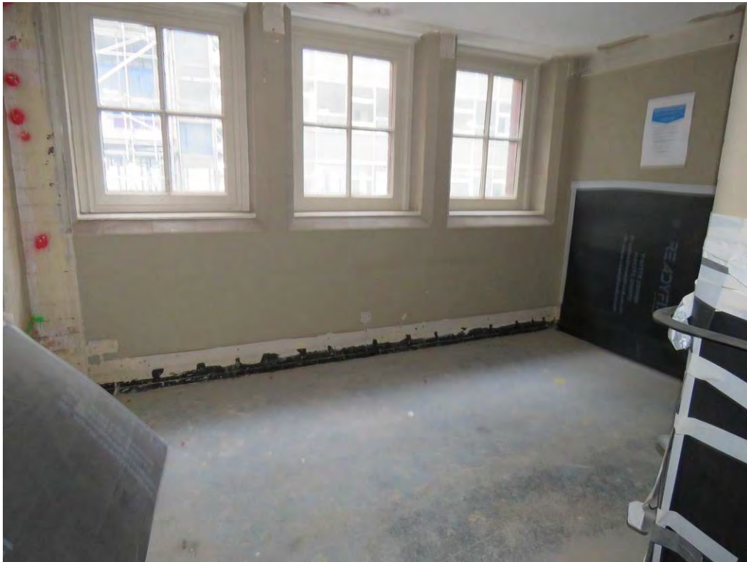
Figure 104: Looking across north-west across the former boys' staircase landing (FM8). The original glazed brick/exposed red brick will have its modern paint layers removed as part of the consented scheme.
