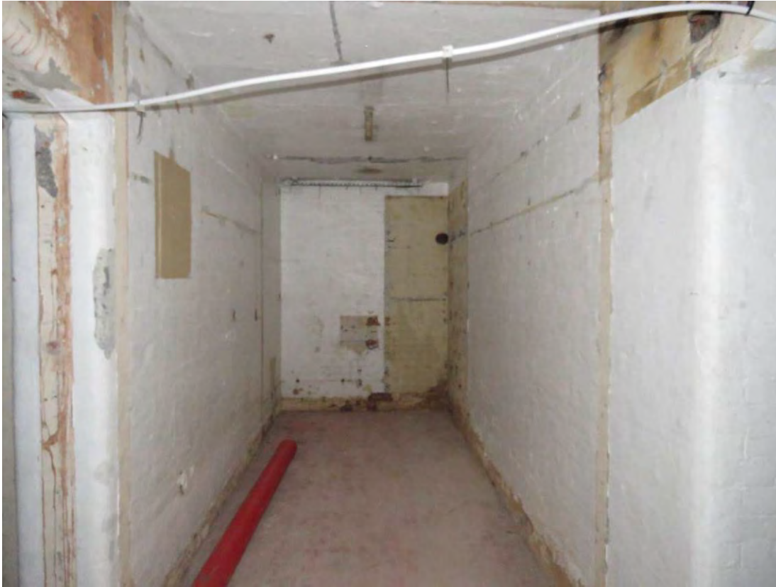
Figure 37: Looking east into B3 which forms a continuation of corridor B4.
