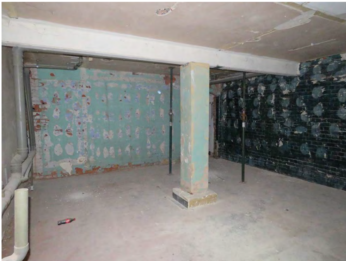
Figure 32: Looking south-west across the former store room (B5).
