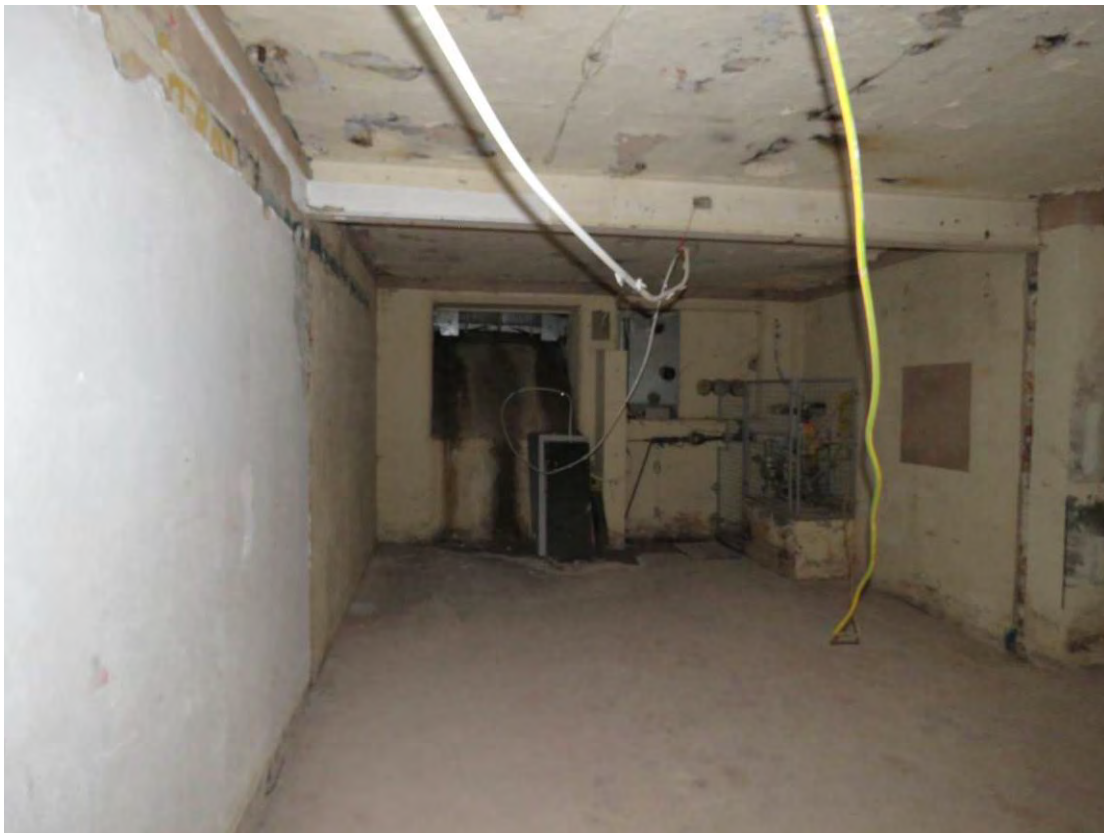
Figure 38: Looking south into the original kitchen (B1), showing the two original window openings which terminate at pavement level.
