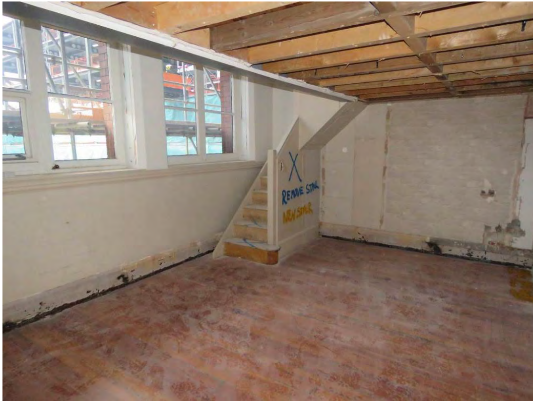
Figure 77: Looking south-west across F1, showing an example of a modern 2004 hotel mezzanine and stairs and area of original timber floorboards, which will be covered with modern flooring as part of the consented scheme.
