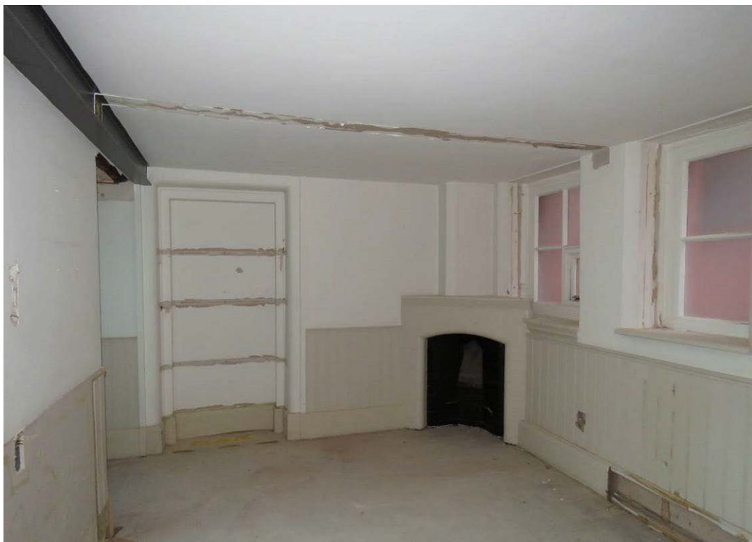
Figure 92: Looking north-west across F27a, which originally formed a teacher's office. To the right is the original office fireplace which will be retained and redecorated as part of the consented scheme. The blocked doorway formed the sole original entrance into the office from the girls' school hall.
