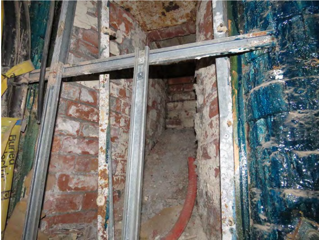
Figure 39: Looking into one of two now blocked air vents which terminated either side of the boys' entrance.
