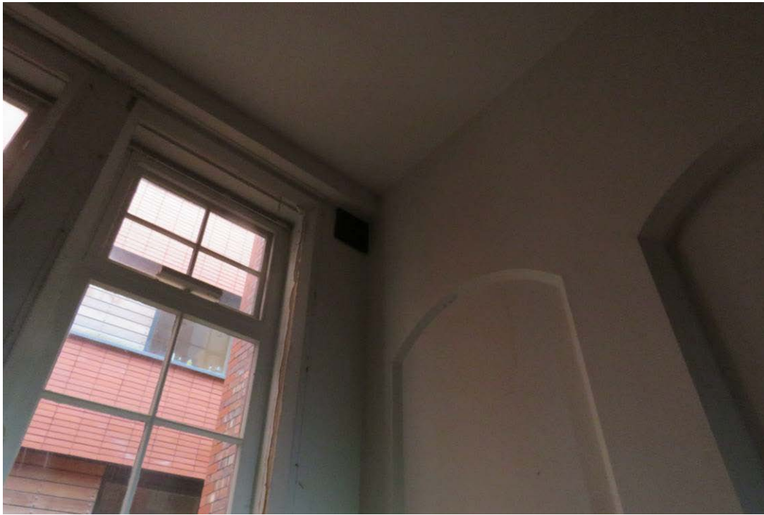
Figure 95: Looking north-east across F25, which originally formed a girls' classroom. An original/early metal ventilation grill can be seen to the right of the right-hand window, which will be retained and redecorated as part of the consented scheme.
