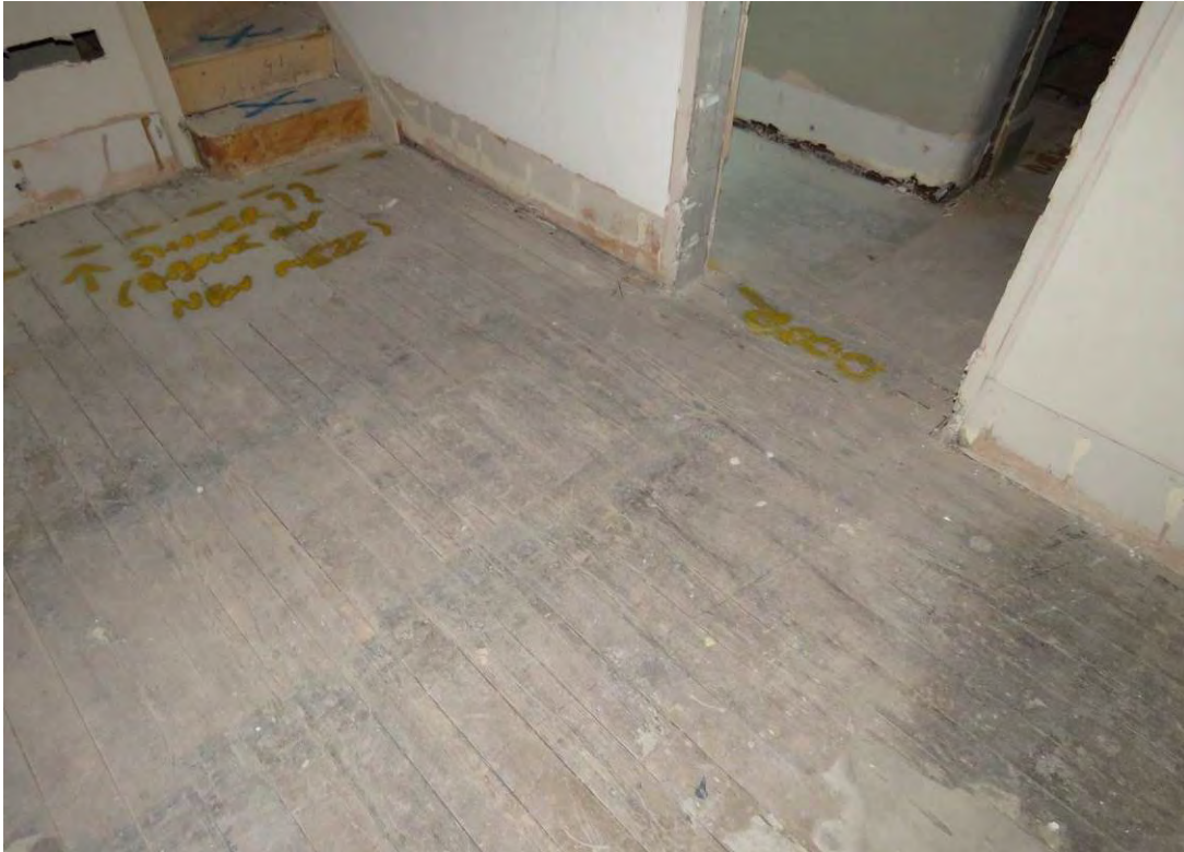
Figure 99: Detail of an area of original timber floorboards in F23, which will be re-covered with new timber flooring as part of the consented scheme.
