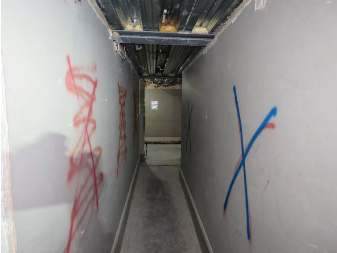
Figure 45: Looking north through G2 towards the original boys' corridor (G18). This space originally formed part of a larger classroom.
