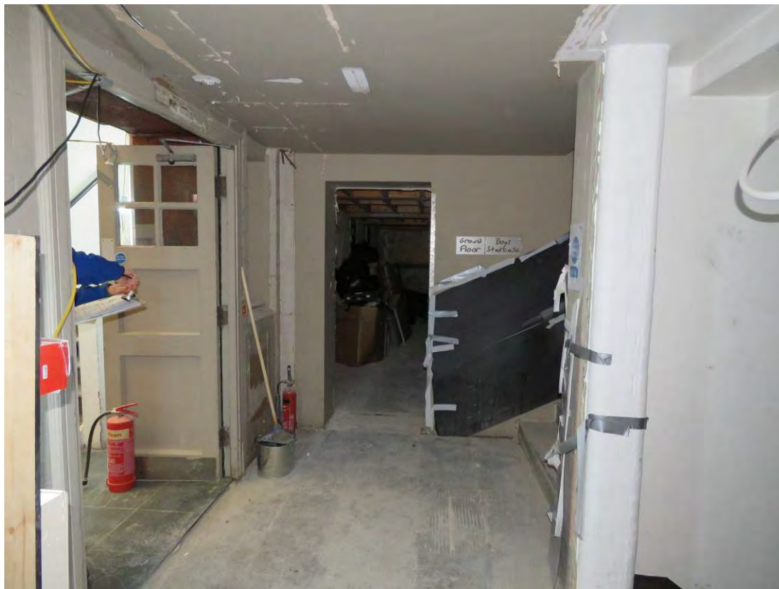
Figure 55: Looking north into the former boys' staircase (G20). The double doors to the left will be retained and redecorated, and the original glazed brick/exposed red brick walls will have their modern paint layers removed as part of the consented scheme.
