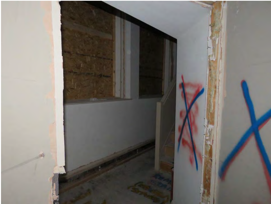
Figure 43: Looking south-west into G1, which formed one of the original infant's classrooms.
