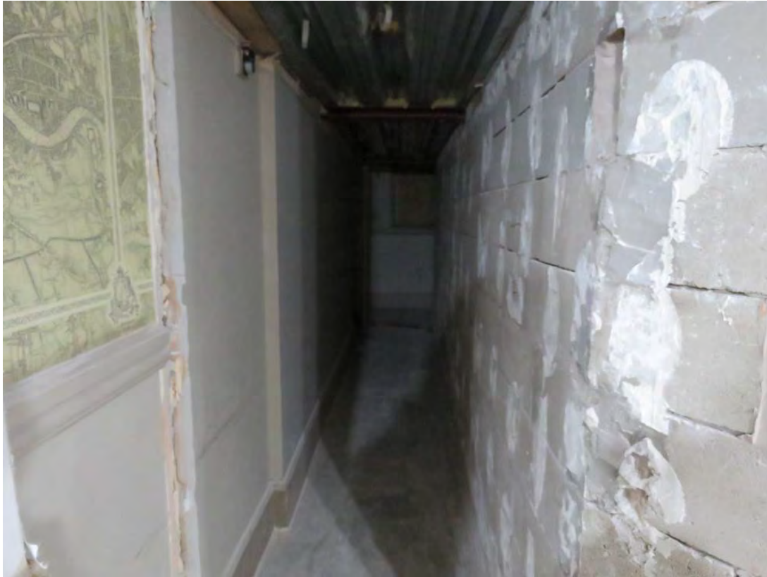
Figure 47: Looking south into G12, which originally formed part of a boys' classroom.
