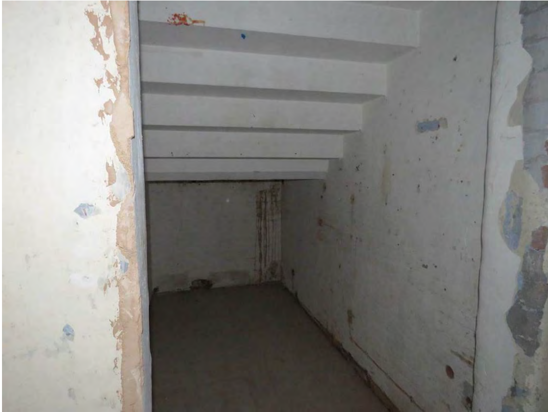
Figure 35: A view looking beneath the boys' staircase (B4).
