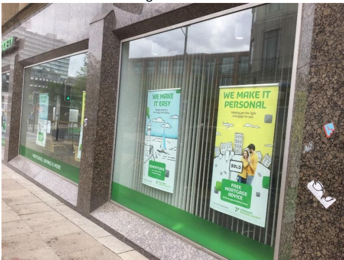
View of existing shopfront finish
