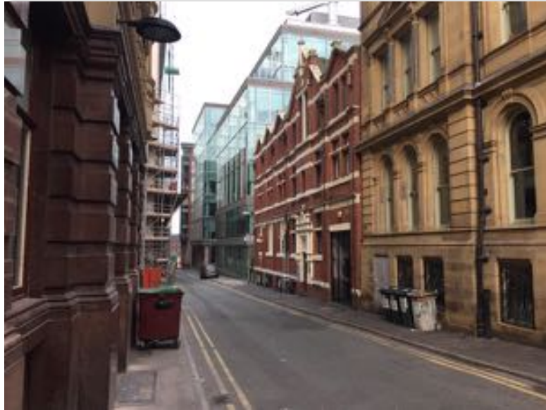
Photograph 3.1 – Existing Invicta House Entrance on Atkinson Street
