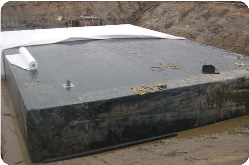
2mts deep tank with 3mts cover
