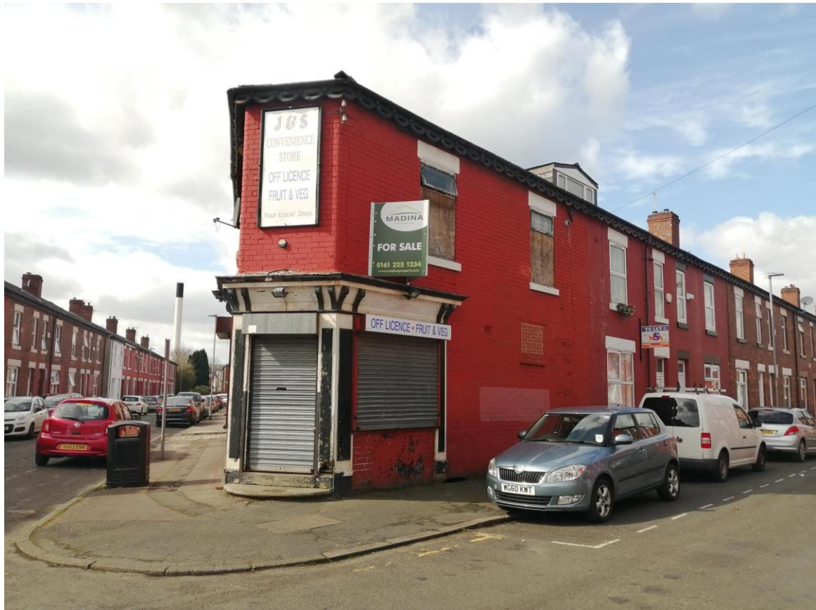
Figure 4: 20 South Grove (South Grove elevation).
