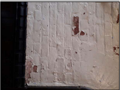
P52 - View of Tenant Hall / Suite A0/36. To remove flaking paint finish to section of brick wall to left hand side of doorway. To prepare surface prime / seal and repaint all brickwork to the hall.
