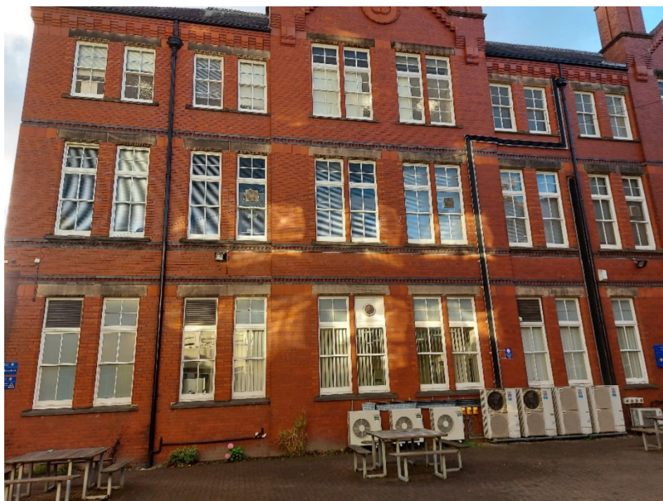
1920s red-brick extension
