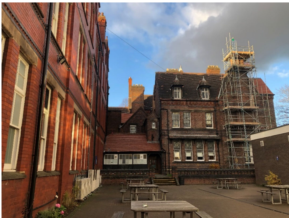
1920s extension to left of the original listed Firwood Building
