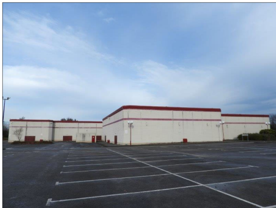
Plate 5. Showcase Cinema (southern elevation)
