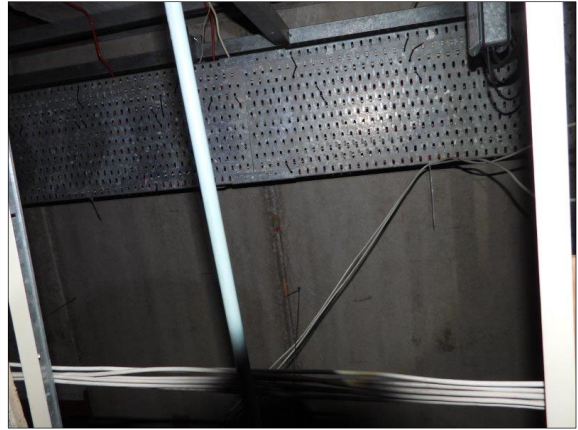
Plate 18. Showcase Cinema (Roof)
