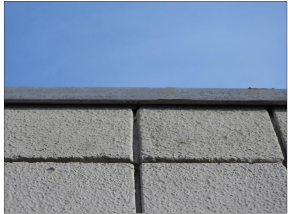
Plate 20. Showcase Cinema (Roof)
