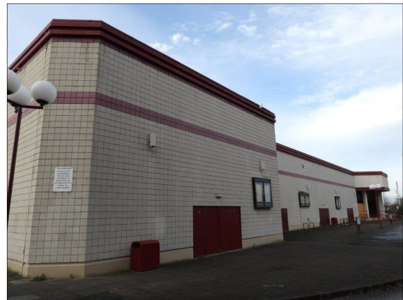
Plate 6. Showcase Cinema (north-east elevation)
