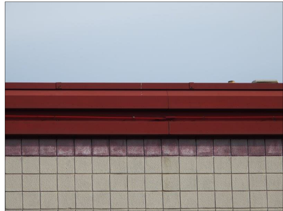
Plate 10. Showcase Cinema (metal gutter-boxing)
