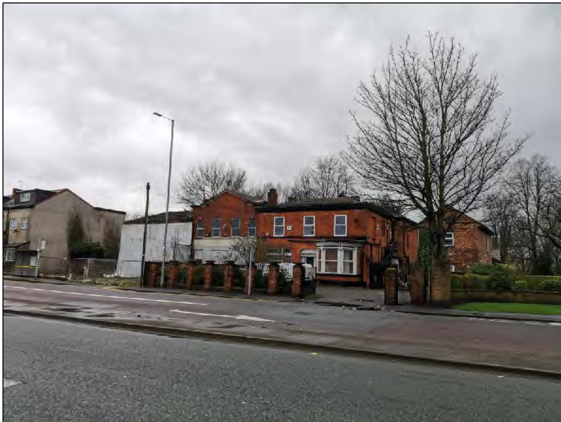
Plate 18: Looking west towards 691-695 Rochdale Road
