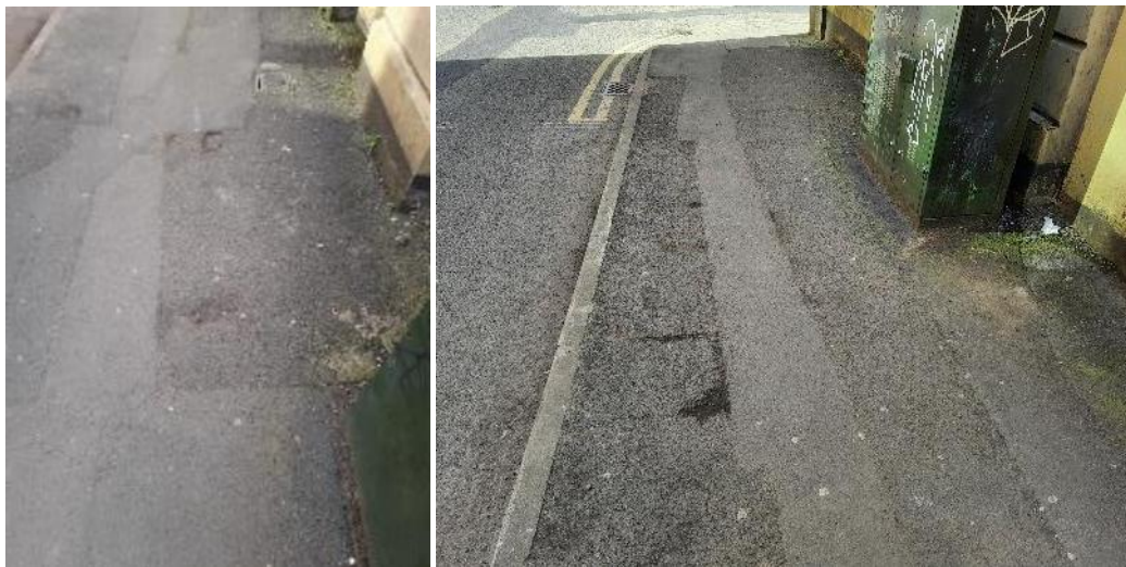
Figures 3.1 and 3.2 – Illustration of reinstated strip of footway surface
