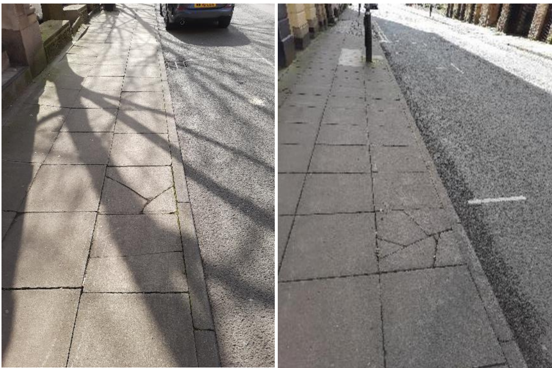
Figure 3.8 – Raised edge of paving stones alongside 11 Bloom Street
