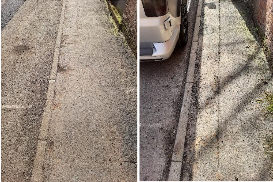
Figure 3.11 – Missing kerbstone on Mindel House side of gated alleyway and surface gouging
