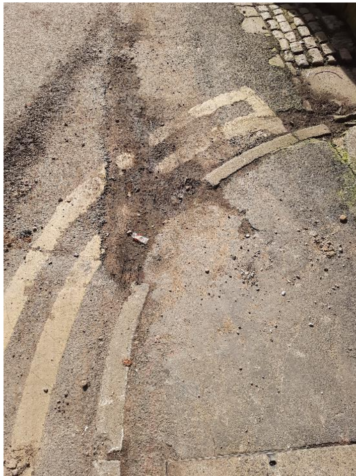
Figure 3.11 – Missing kerbstone on Mindel House side of gated alleyway and surface gouging
