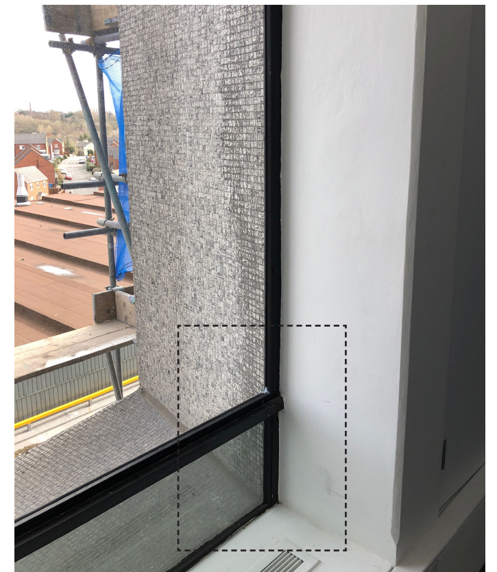
Existing Crittal windows with low level transom
