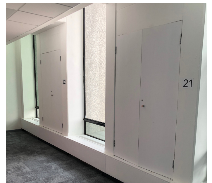
Replacement service void doors and stall riser: painted white finish.
