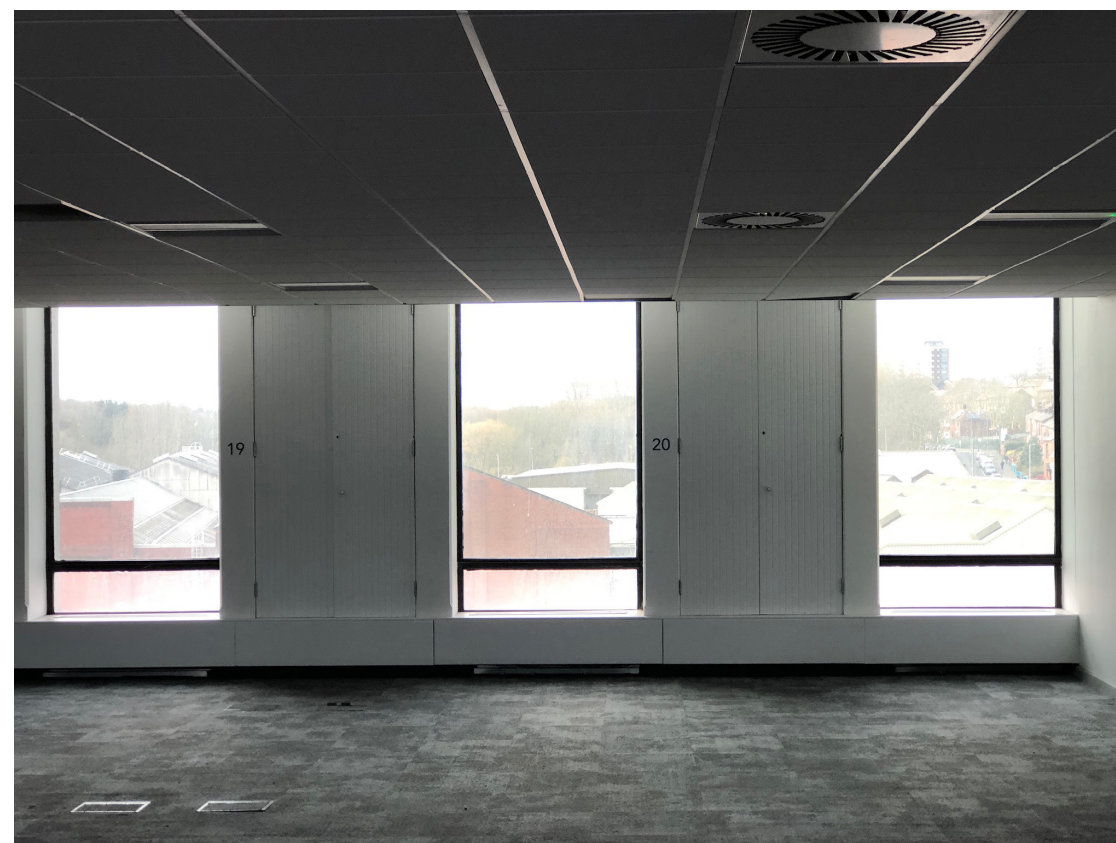
View of internal finish and suspended ceiling
