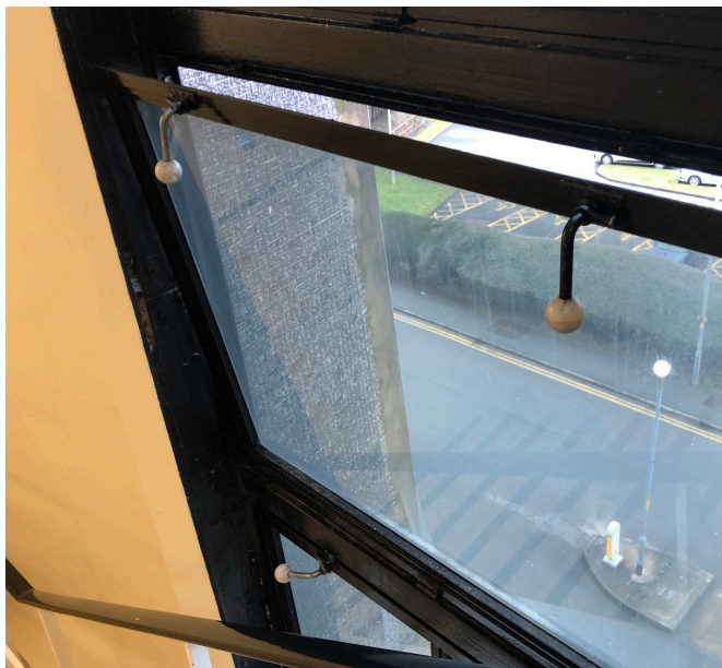
Existing winding gear to stairwell windows
