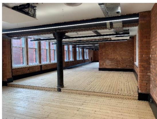
Figure 3: Looking south along the east side of the first floor. Note the changes in level and directions of timber floorboards which denotes the historic subdivision of the space.
