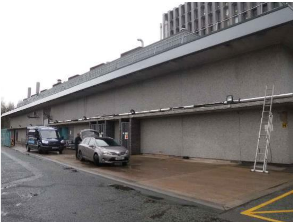
Photo B.86: General view of the east elevation of the East Machine Hall
