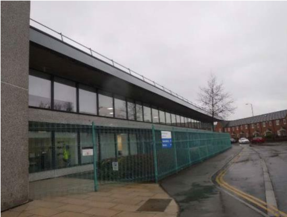
Photo B.77: General view of the East Machine Hall, south elevation
