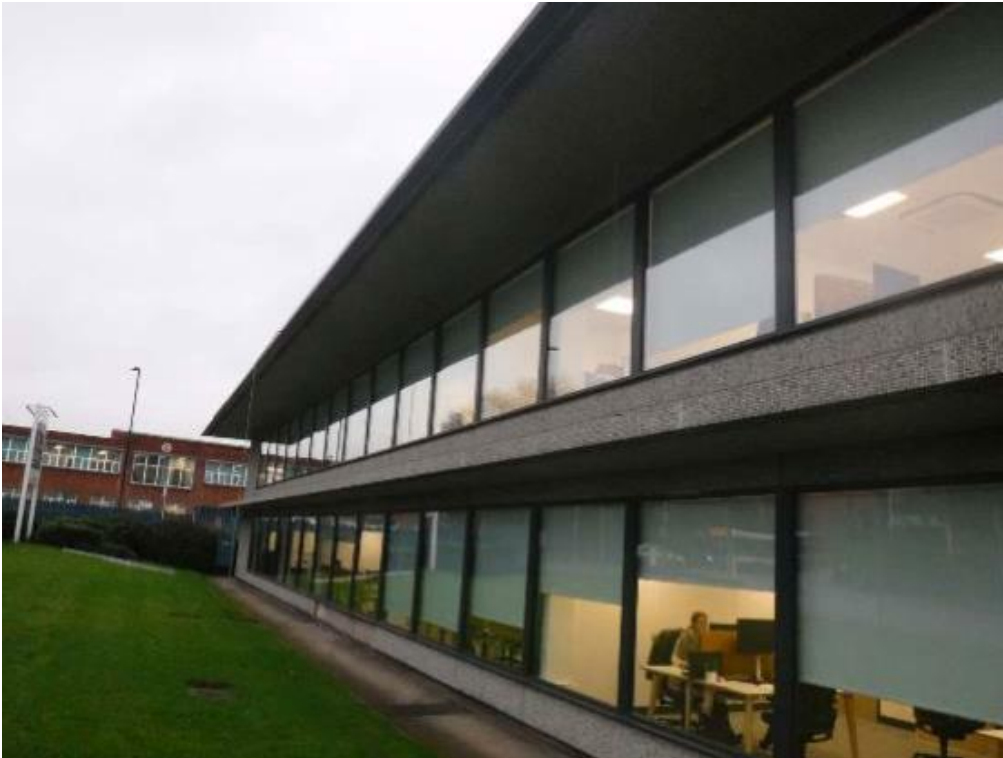
Photo B.53: General view of the south elevation of the west machine hall
