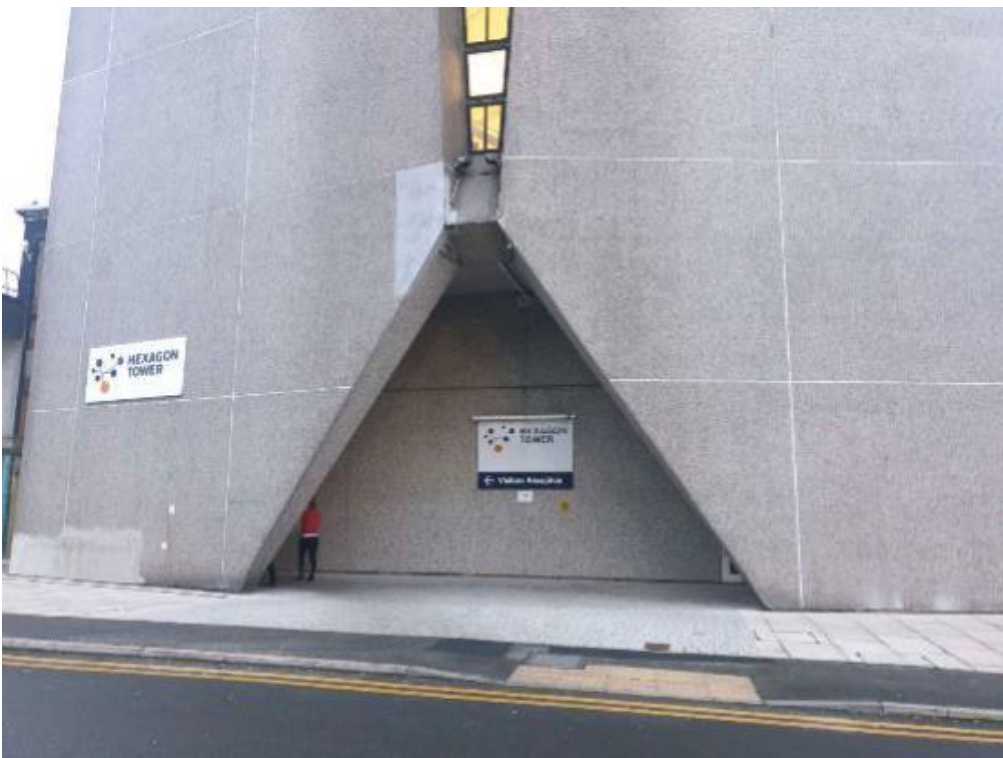
Photo B.92: General view of the south entrance to Hexagon Tower
