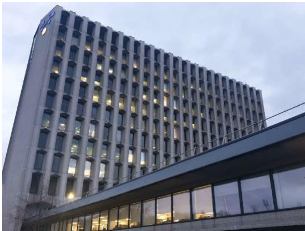
Photo B.3: General view of the east elevation of Hexagon Tower
