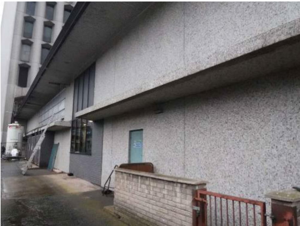
Photo B.44: General view of the north elevation of the west machine hall
