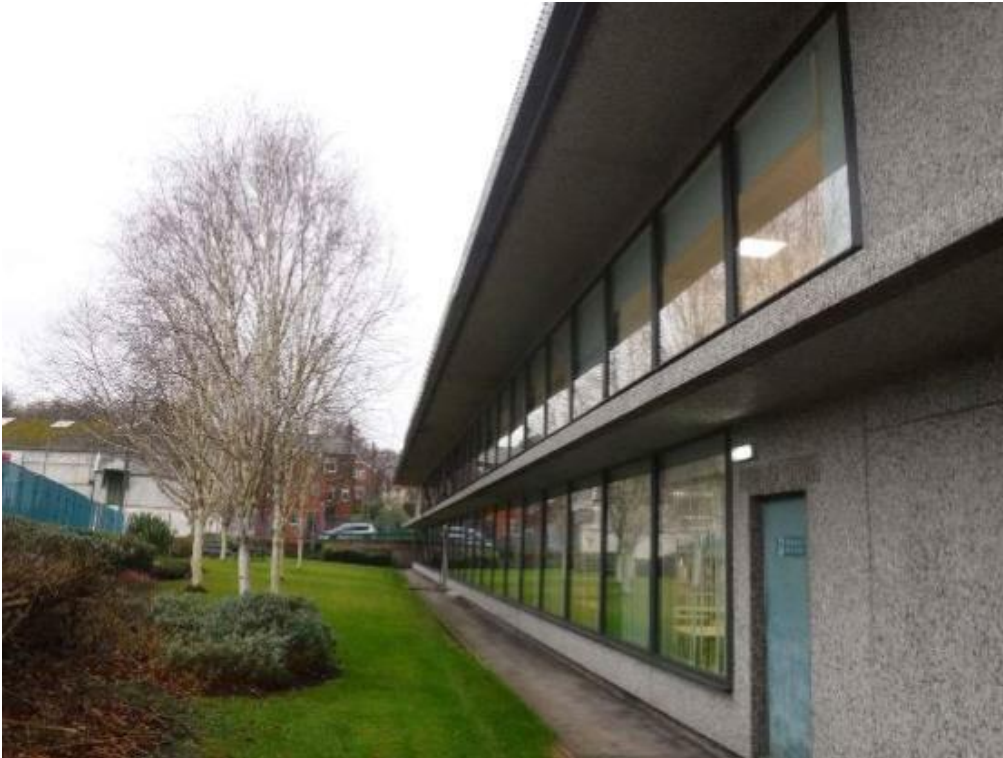
Photo B.65: General view of the west elevation of the west machine hall
