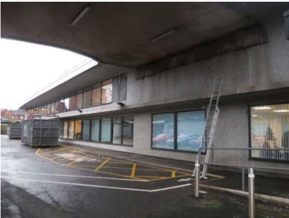
Photo B.72: General view of the north elevation of the East Machine Hall
