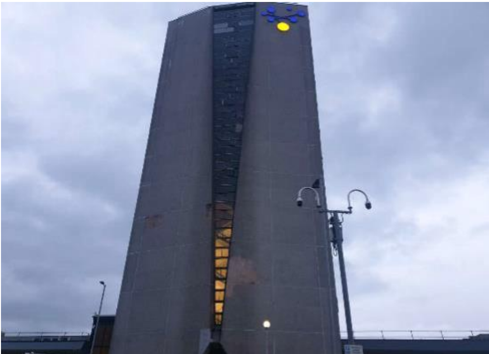
Photo B.2: General view of the south elevation of Hexagon Tower
