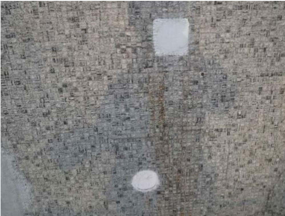
Photo B.19: A view showing two repaired core holes in the south elevation at ground level
