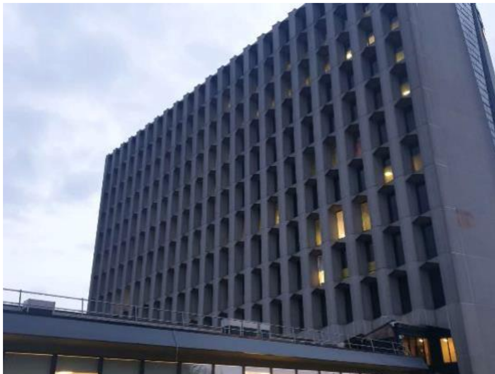
Photo B.4: General view of the west elevation of Hexagon Tower
