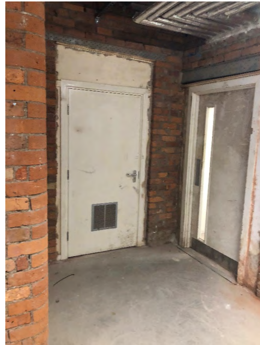
Figure 3.52 Photo of Room B1.06/B1 CORR.02 (Source : Photograph taken by author 21/03/21)
