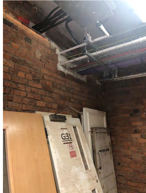
Figure 3.48 Photo of Room B1.05 (Source : Photograph taken by author 21/03/21)
