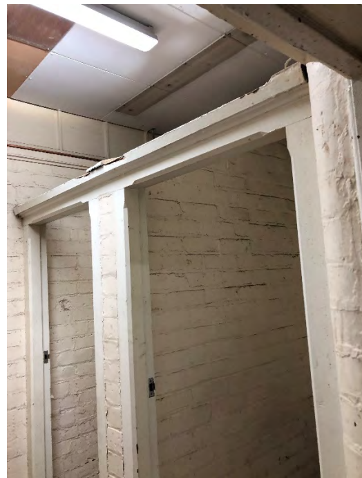
Figure 3.60 Photo of Room B1.25 (Source : Photograph taken by author 21/03/21)
