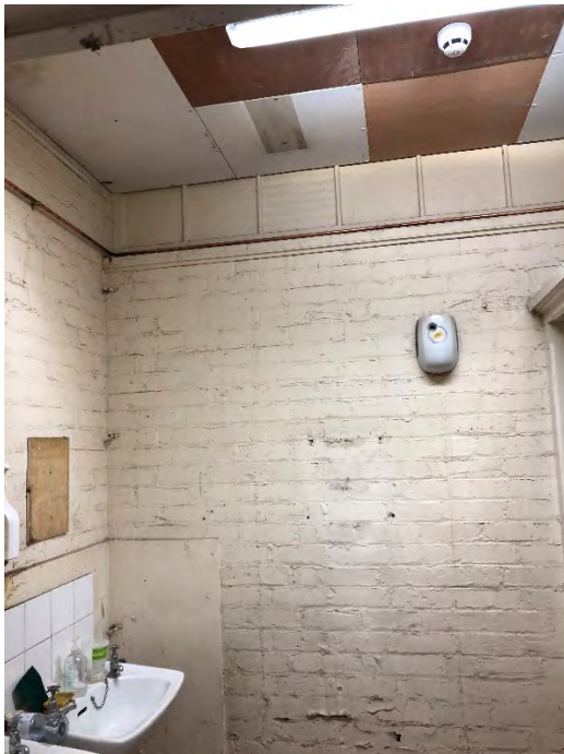
Figure 3.59 Photo of Room B1.25 (Source : Photograph taken by author 21/03/21)
