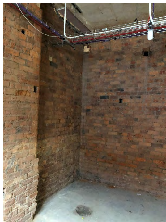
Figure 3.54 Photo of Room B1.06/B1 CORR.02 (Source : Photograph taken by author 21/03/21)
