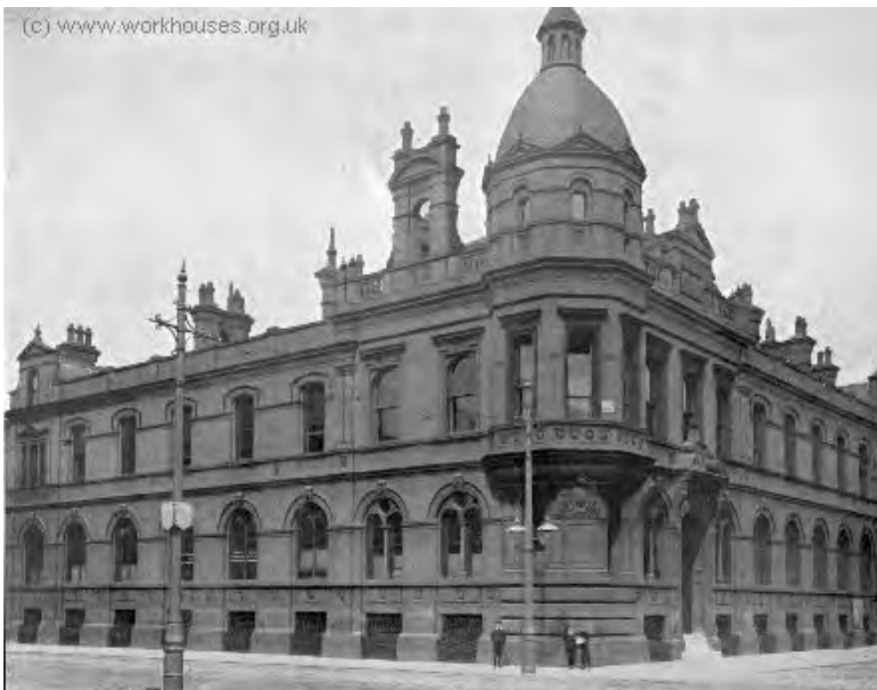
Figure 3.14 Photograph dating from the early 1900's looking towards the corner of Lower Ormond Street and Cavendish Street (Source : www.workhouses.org accessed 12/03/2021)
