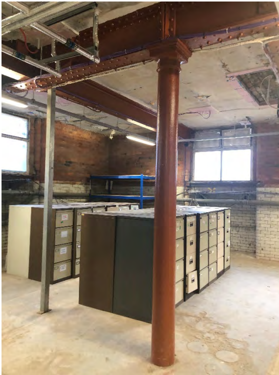
Figure 3.40 Photo of Room B1.03 currently used as Archive Storage (Source : Photograph taken by author 21/03/21)
