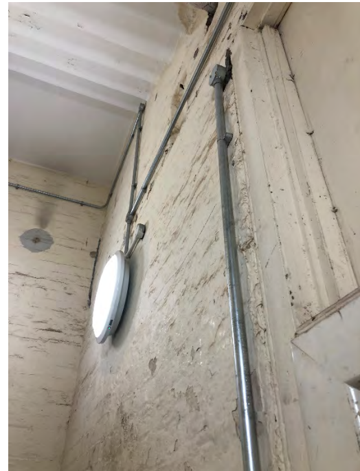
Figure 3.66 Photo of B1 Stair 5 (Source : Photograph taken by author 21/03/21)
