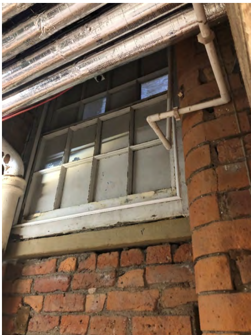
Figure 3.69 Photo of B1 Stair 3 (Source : Photograph taken by author 21/03/21)
