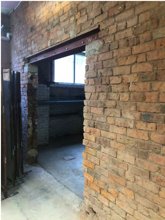
Figure 3.51 Photo of Room B1.06/B1 CORR.02 (Source : Photograph taken by author 21/03/21)
