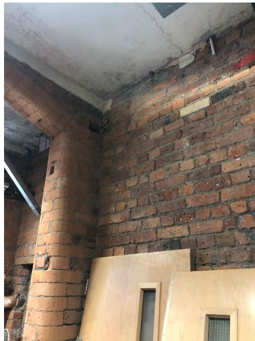
Figure 3.50 Photo of Room B1.05 (Source : Photograph taken by author 21/03/21)
