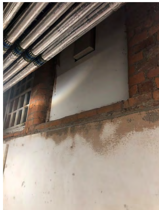
Figure 3.70 Photo of B1 Stair 3 (Source : Photograph taken by author 21/03/21)
