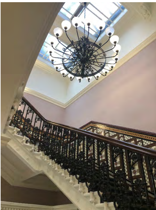
Figure 3.27 Photograph of the restored main stair and rooflight over (Source : photograph taken by author 21/03/2021)
