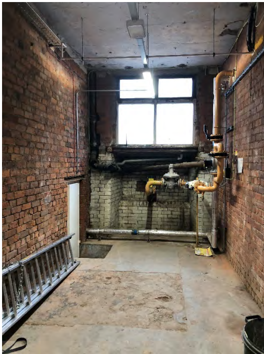
Figure 3.55 Photo of Room B1.18 (Source : Photograph taken by author 21/03/21)
