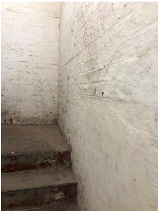
Figure 3.65 Photo of B1 Stair 5 (Source : Photograph taken by author 21/03/21)
