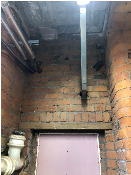
Figure 3.49 Photo of Room B1.05 (Source : Photograph taken by author 21/03/21)
