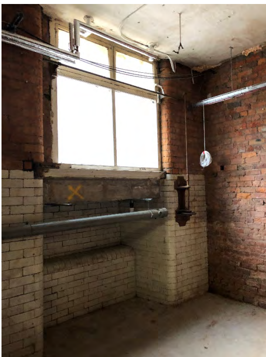
Figure 3.53 Photo of Room B1.06/B1 CORR.02 (Source : Photograph taken by author 21/03/21)
