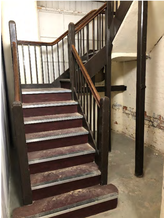
Figure 3.63 Photo of B1 Stair 2 (Source : Photograph taken by author 21/03/21)
