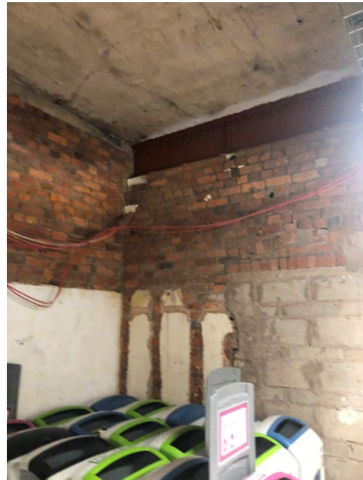
Figure 3.68 Photo of B1 Stair 3 (Source : Photograph taken by author 21/03/21)
