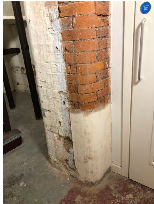
Figure 3.64 Photo of B1 Stair 2 (Source : Photograph taken by author 21/03/21)
