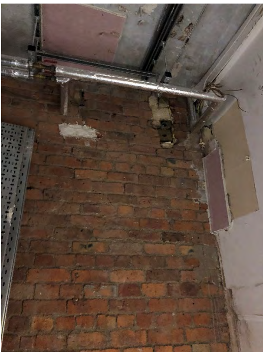
Figure 3.45 Photo of Room B1.04 currently used as a Store Room (Source : Photograph taken by author 21/03/21)
