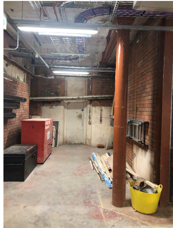
Figure 3.37 Photo of Room B1.01 Basement Storage area (Source : Photograph taken by author, 21/03/21)
