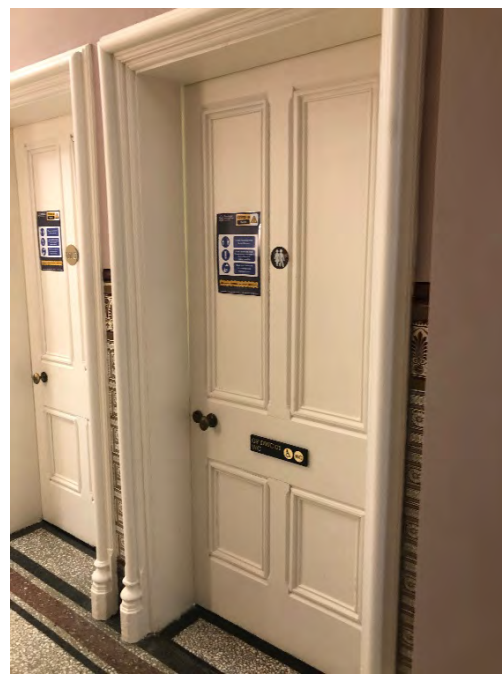
Figure 3.28 Photograph of the restored historic doors and architraves (Source : photograph taken by author 21/03/2021)
