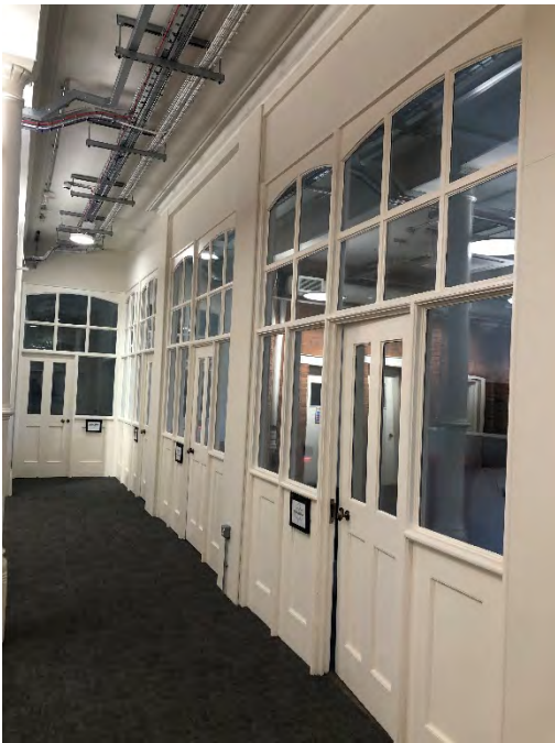
Figure 3.25 Photograph of the replacement glazed screens to the Ground Floor level offices fronting Lower Ormond Street (Source : photograph taken by author 21/03/2021)
