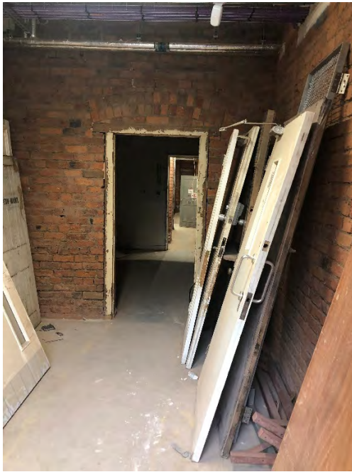
Figure 3.47 Photo of Room B1.05 (Source : Photograph taken by author 21/03/21)
