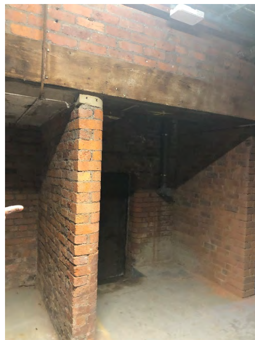
Figure 3.58 Photo of Room B1.19 (Source : Photograph taken by author 21/03/21)
