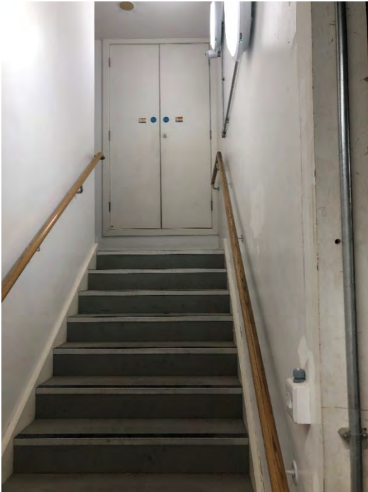
Figure 3.67 Photo of B1 Stair 3 (Source : Photograph taken by author 21/03/21)
