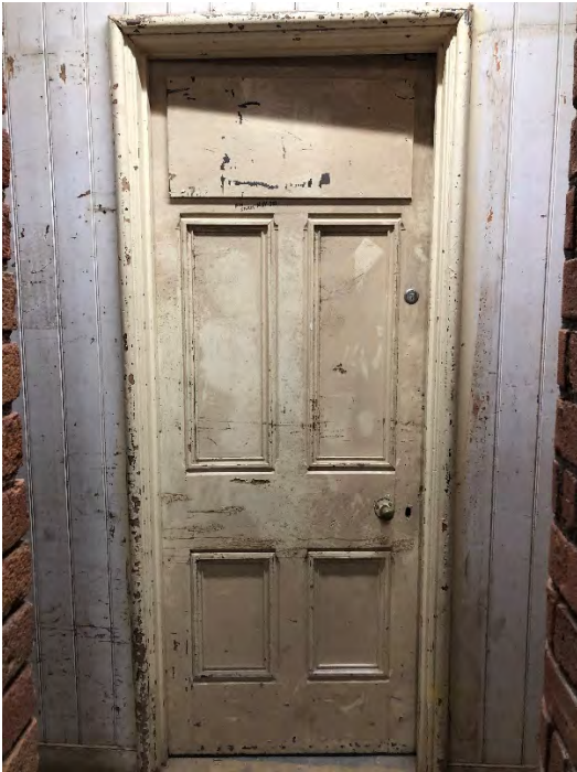
Figure 3.43 Photo of the door to Room B1.04 currently used as a Store (Source : Photograph taken by author 21/03/21)
