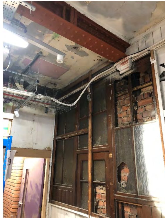
Figure 3.41 Photo of Room B1.03 currently used as Archive Storage (Source : Photograph taken by author 21/03/21)
