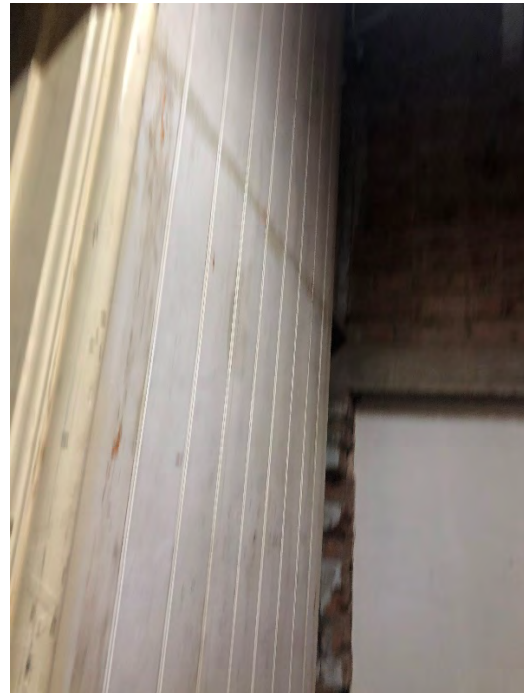
Figure 3.44 Photo of the partition wall to Room B1.04 (Source : Photograph taken by author 21/03/21)
