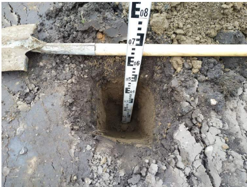
Photograph 13 150mm to topsoil and 450mm of subsoil emplaced in VP03.
