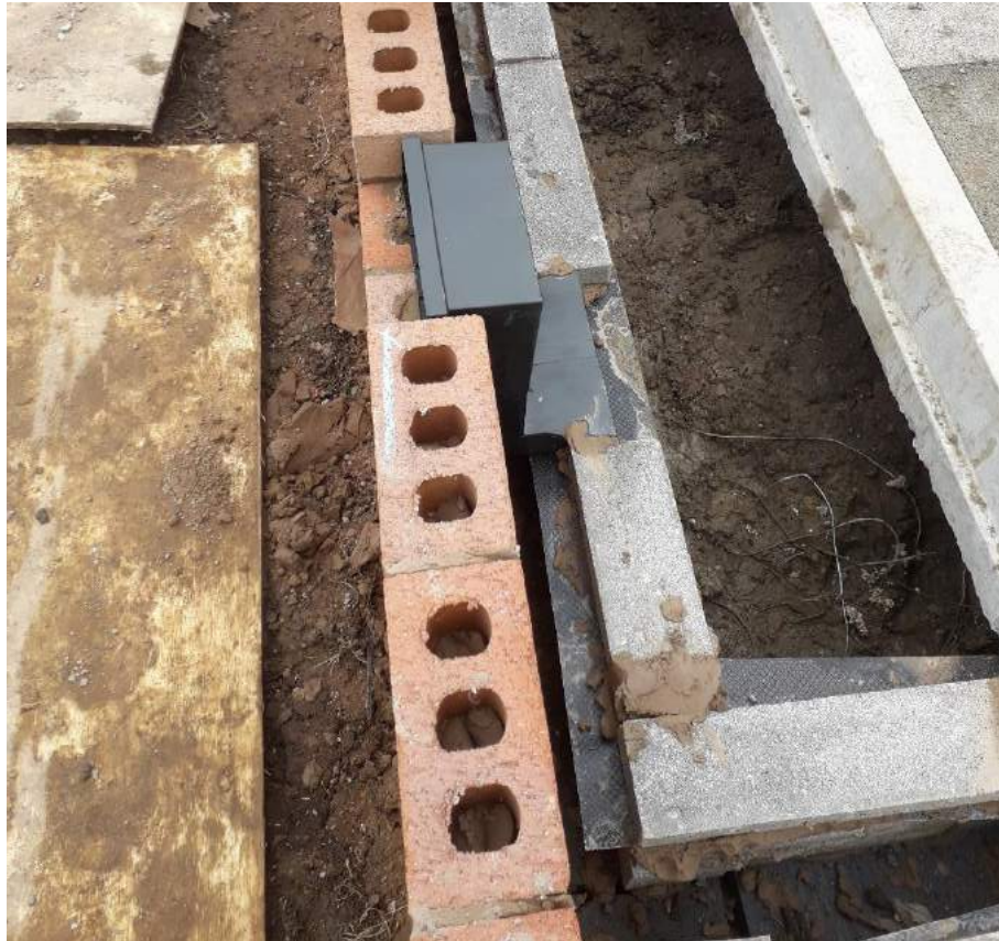
Photograph 1 Swan neck vent being installed into Plot 1 & 2.
