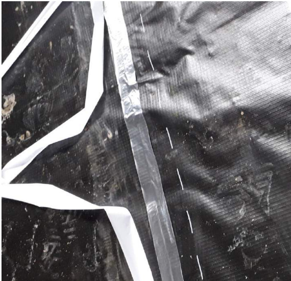
Photograph 7 Close up of surface taping to edge joints.
