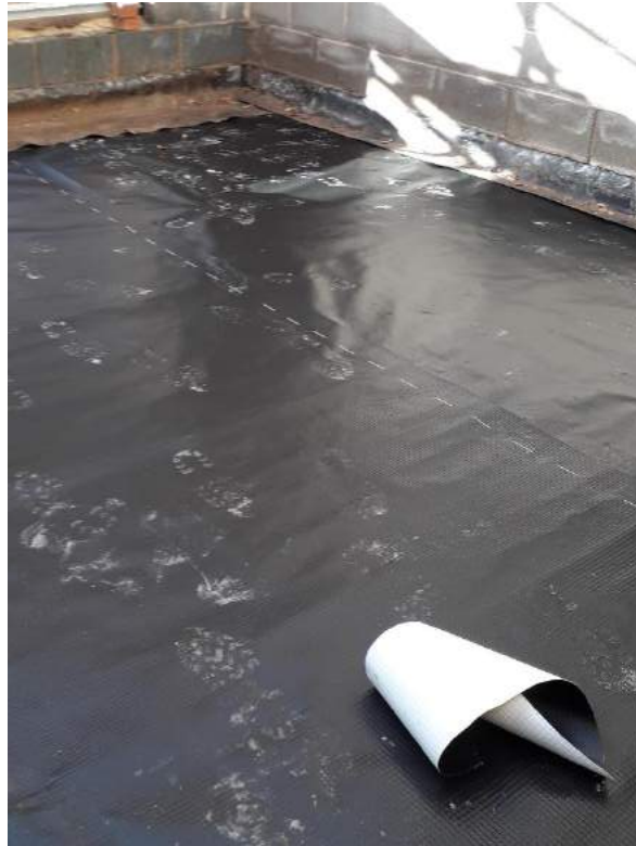
Photograph 8 Plot 3 indicating width of membrane to minimise internal lapping.
