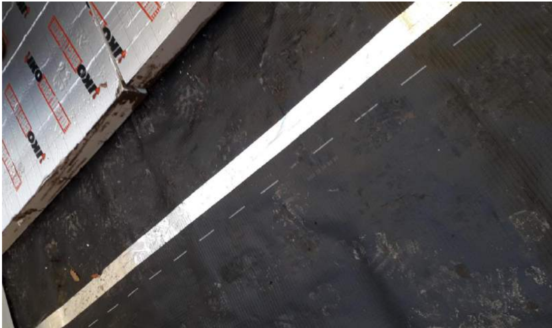
Photograph 6 Lapped and taped Radbar hydrocarbon membrane within Plot 1, with insulation to the surface.
