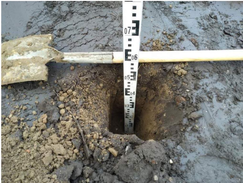
Photograph 9 150mm to topsoil and 450mm of subsoil emplaced in VP01.
