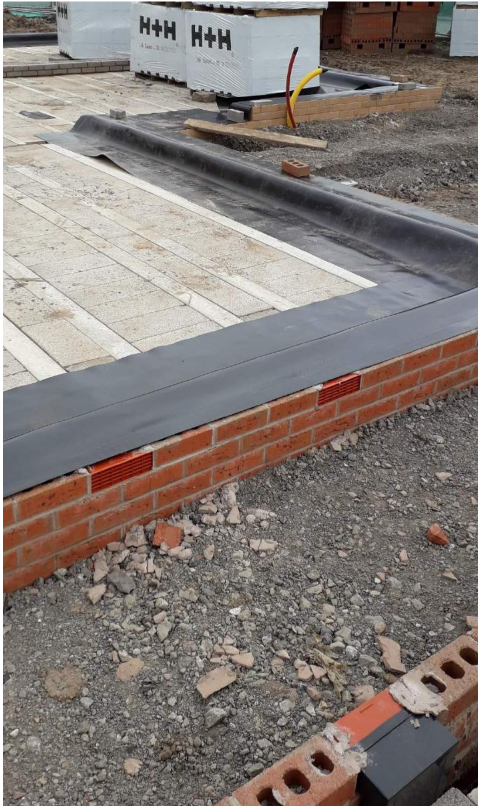
Photograph 3 Vents and edge details to Plots 3 and 4 with vent of Plot 2 to right.
