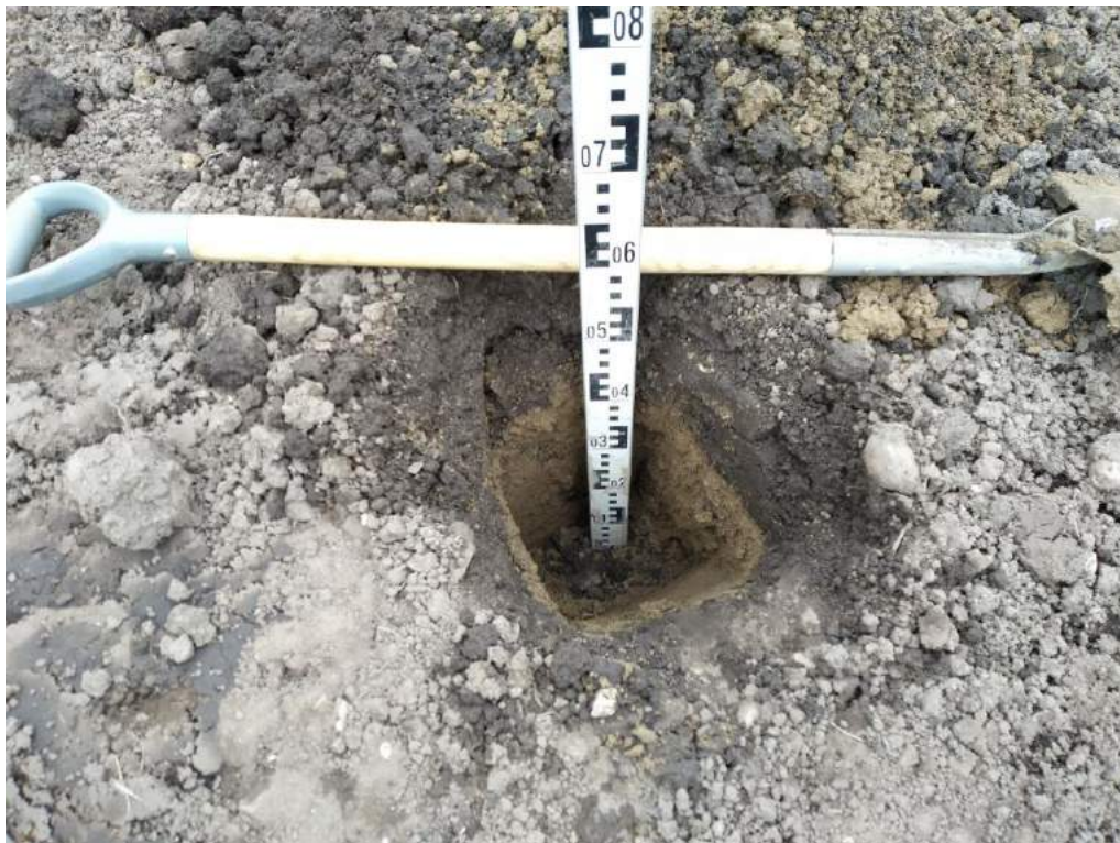
Photograph 15 150mm to topsoil and 450mm of subsoil emplaced in VP04.
