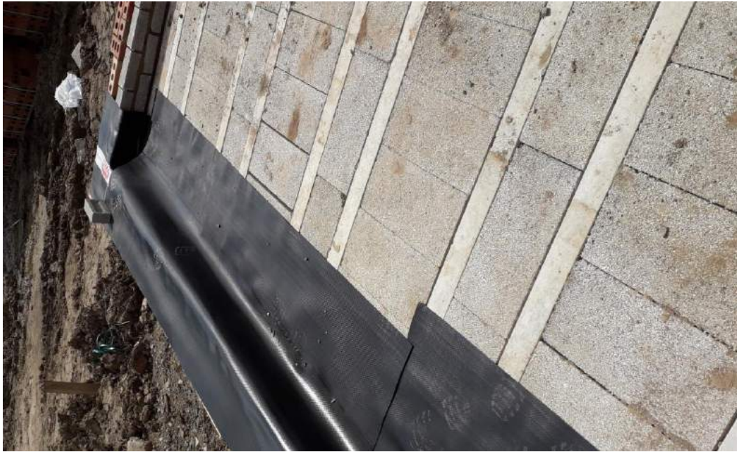
Photograph 4 Beam and Block floor with edge details to Plots 3 and 4
