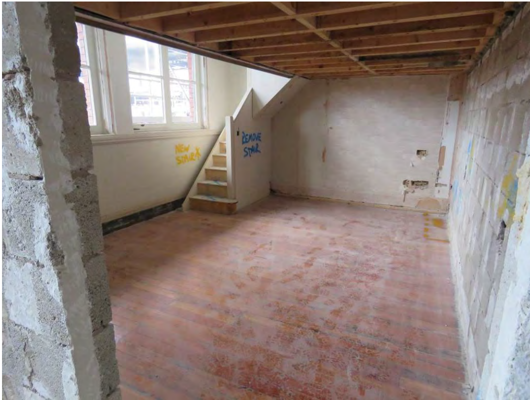
Figure 112: Looking south-west across S1, which formed an original boys' classroom. The original timber flooring will be covered as part of the consented scheme.
