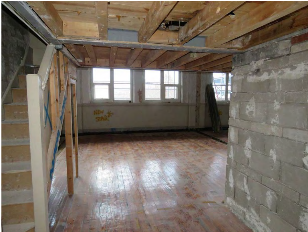
Figure 115: Looking south across S5 showing an original example of timber floorboards, which will be covered with new timber floor as part of the consented scheme.
