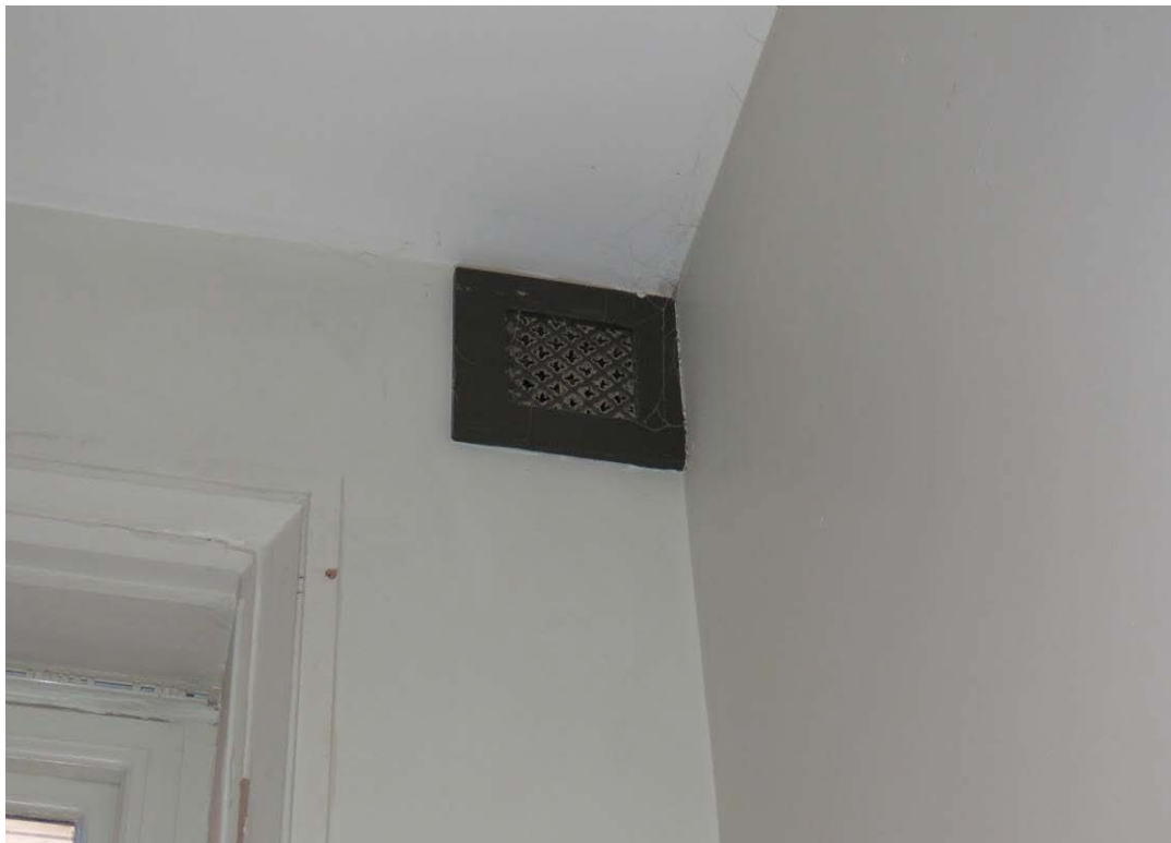
Figure 122: An example of an original/early metal ventilation grill to the north-east of S21, which formed the original boys' school hall. The vent will be retained and redecorated as part of the consented scheme.
