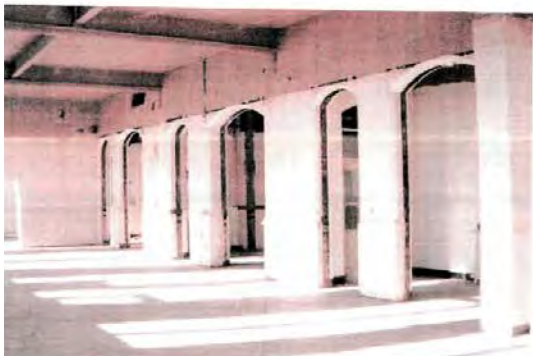
Figure 181: 2004 photographic survey – Internal third floor classroom views.
