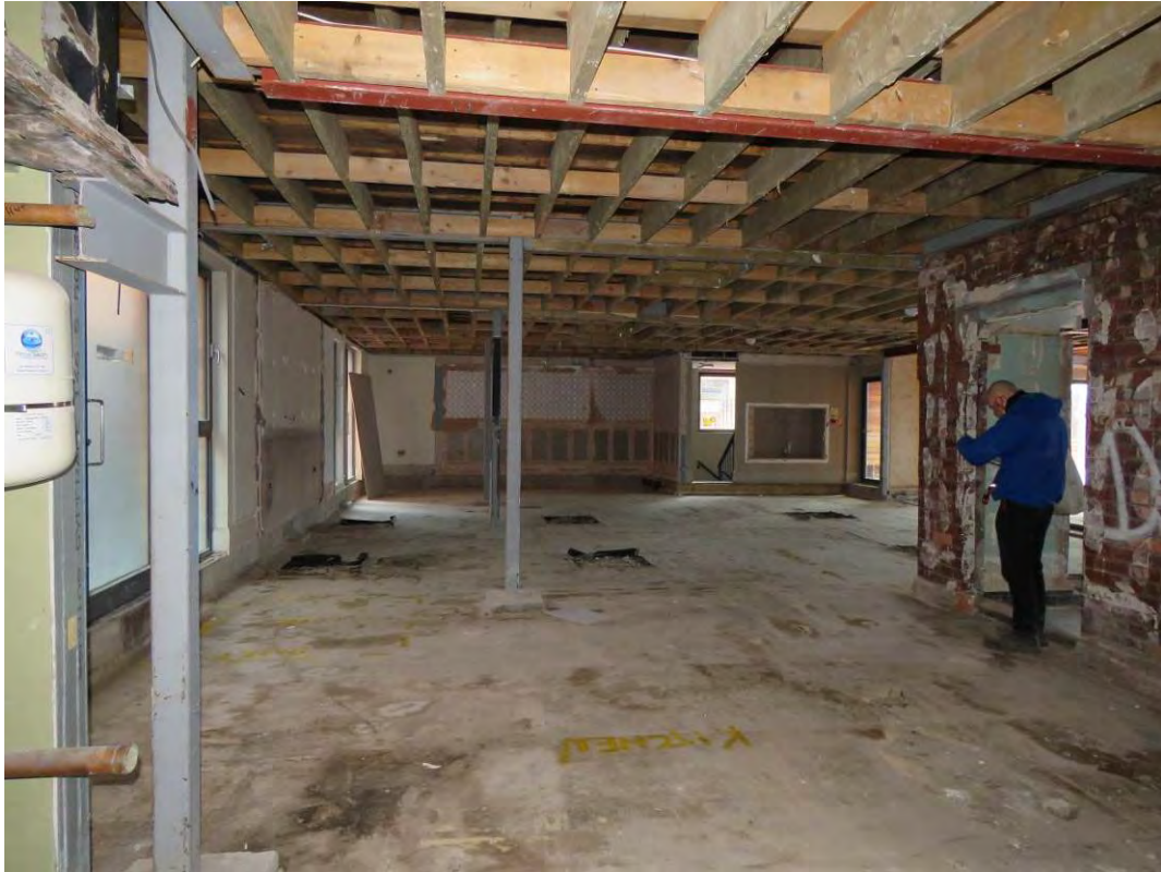
Figure 138: Looking east across T3 from the location of the now removed modern toilets (T7), showing the 2004 roof extension.
