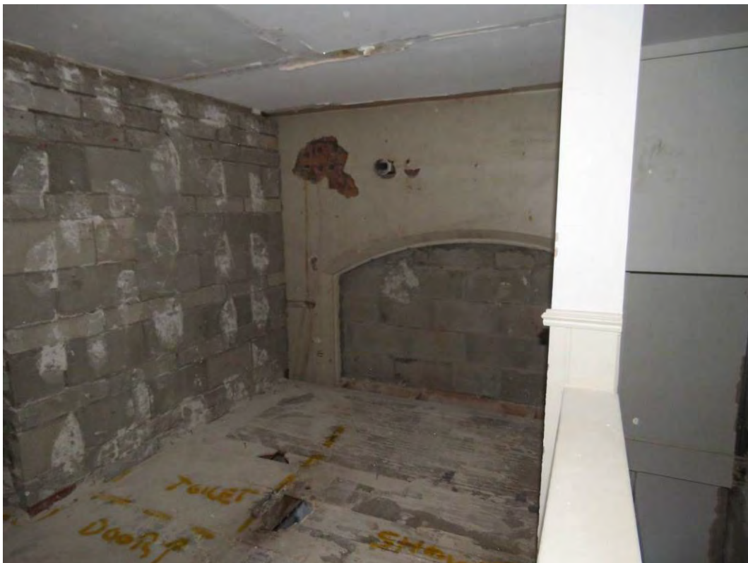
Figure 131: Looking north towards the now blocked original internal window opening of SM4. The arch will be re-covered as part of the consented scheme.
