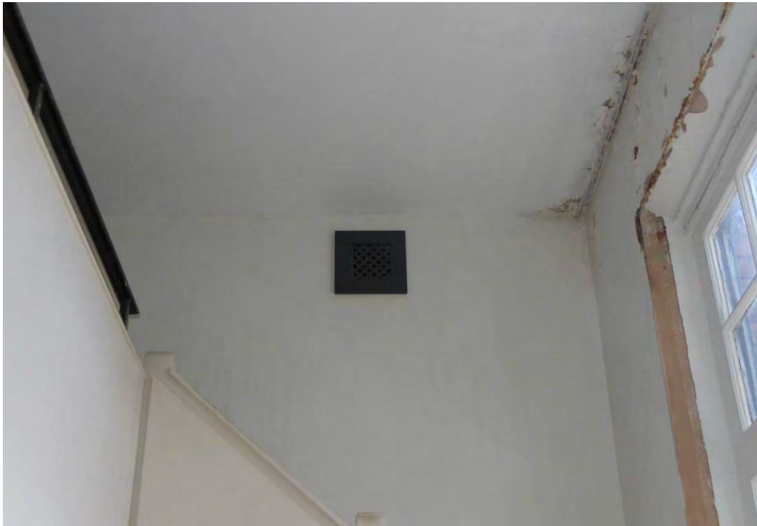
Figure 116: An example of a surviving original/early ventilation grill in the south-east corner of S9, which originally formed a boys' classroom, which will be retained and redecorated as part of the consented scheme.
