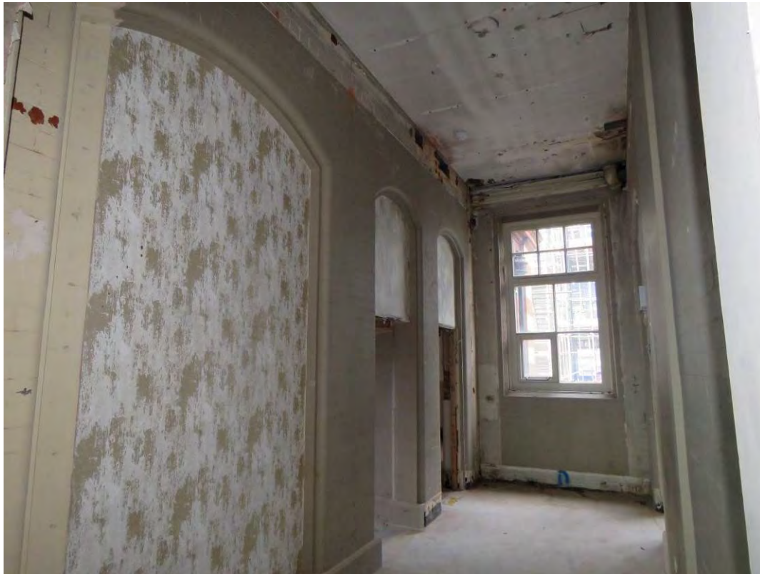
Figure 121: Looking west along S12 which formed the original boys' corridor, showing the original arched window and door openings to the former boys' classrooms (left). The original glazed brick/exposed red brick will have its modern paint layers removed as part of the consented scheme.
