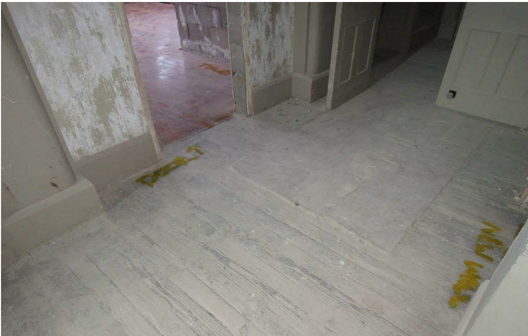
Figure 119: A view of the surviving original floorboards to the southern side of the original boys' school hall floor, which will be covered as part of the consented scheme.
