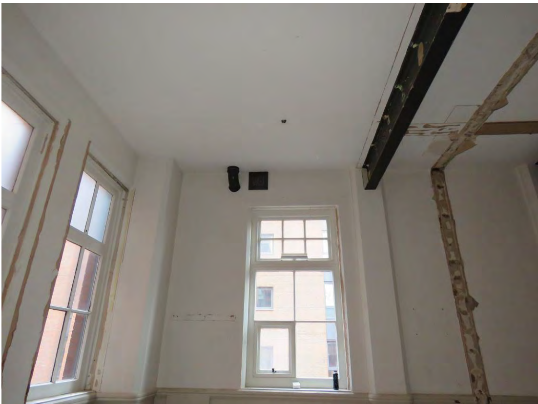
Figure 126: An example of a surviving original/early metal ventilation grill to the east elevation of S20, which will be retained and redecorated as part of the consented scheme.
