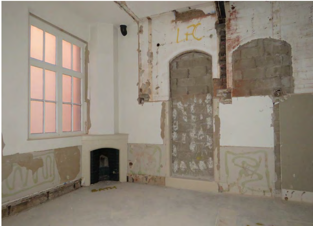
Figure 123: Looking north-east across S23, which originally formed the boys' principal teacher's office to the left, accessed from the boys' school hall (left blocked opening), whilst the blocked opening to the right formed the entrance to the original boys' cloakroom, accessed from the boys school hall. The original glazed brick fireplace to the former office will be retained and redecorated as part of the consented scheme.
