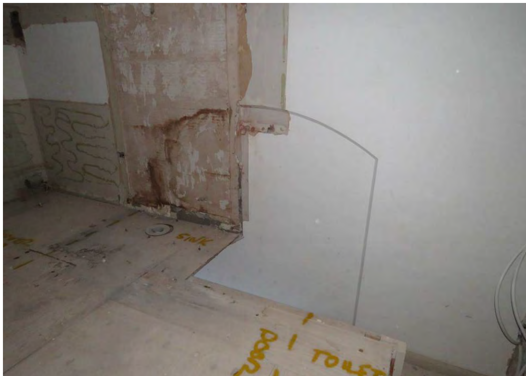
Figure 129: Looking north-west towards the north wall of SM3, illustrating an original internal window opening (now blocked). The arch will be partially re-covered as part of the consented scheme.
