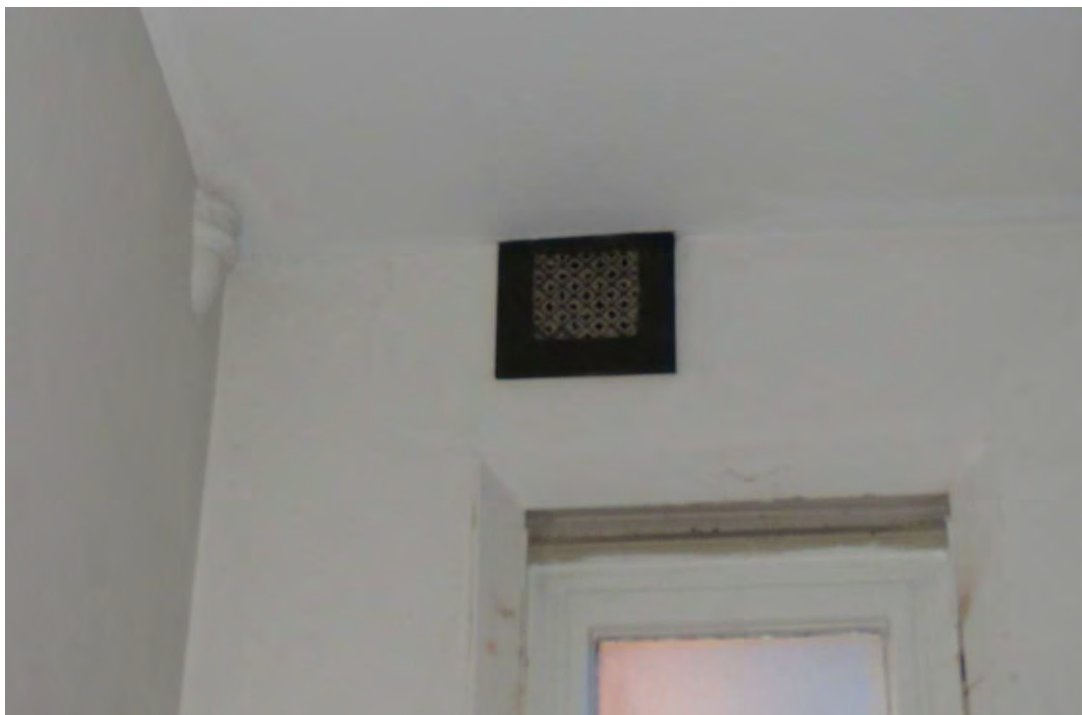
Figure 124: A surviving original/early metal ventilation grill to the former boys' toilet in S23, which will be retained and redecorated as part of the consented scheme.
