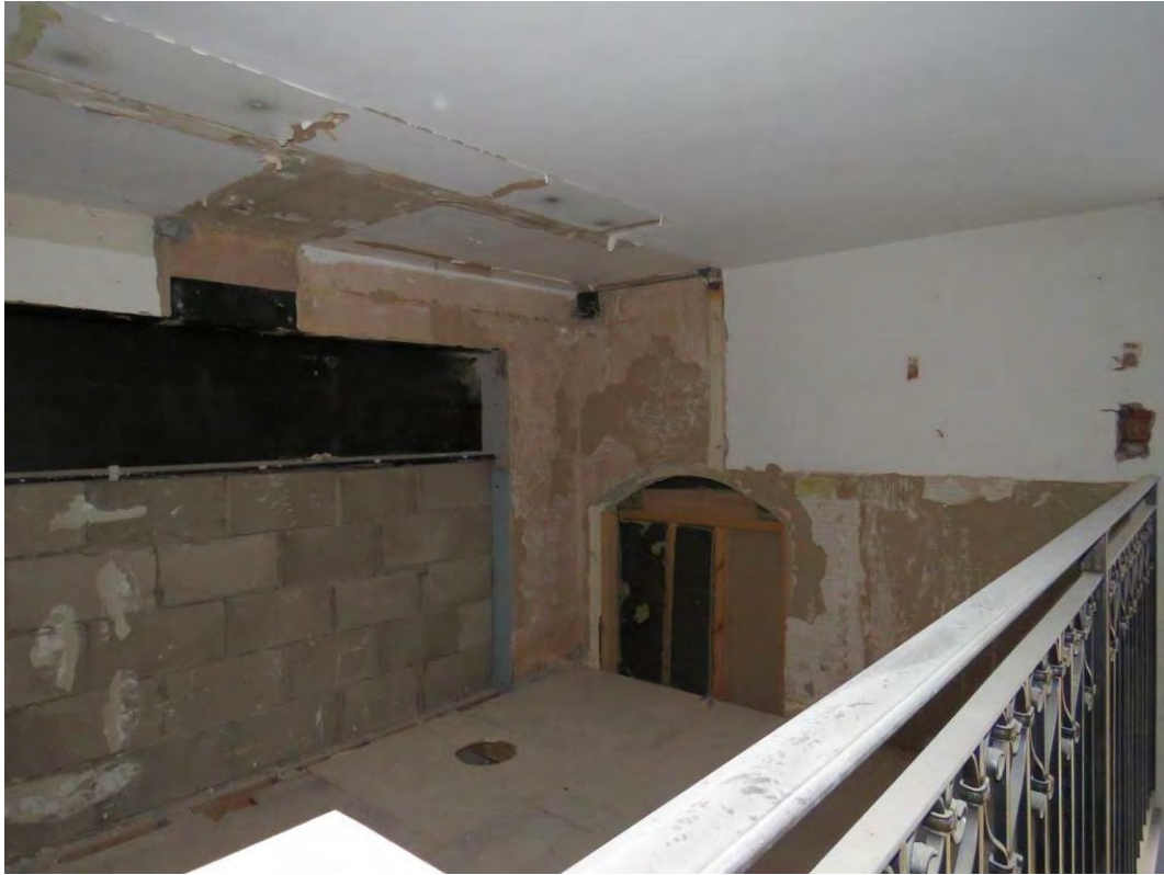
Figure 134: Looking north-west across SM6 towards the now blocked original door opening to the former second floor boys' classroom below. The arch will be re-covered as part of the consented scheme.
