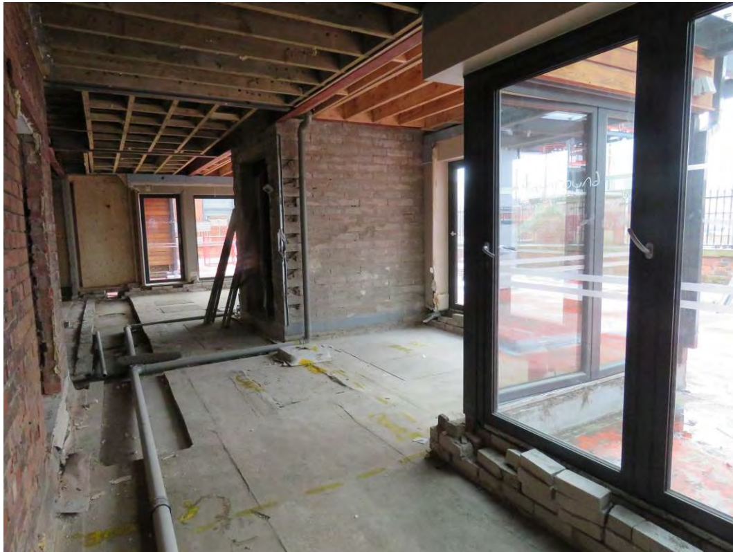
Figure 136: Looking south-west across towards the modern 2004 passenger lift enclosure (centre). The wall to the left forms the original external boys' staircase wall.
