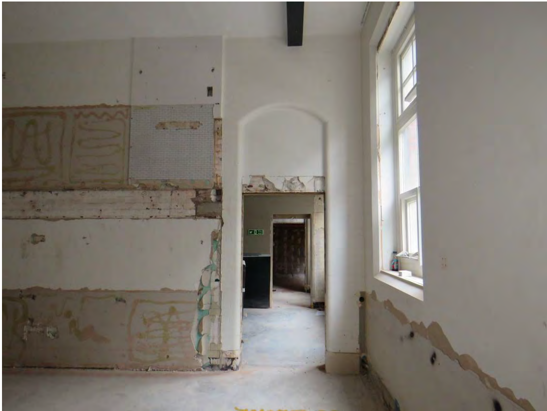
Figure 125: Looking south across a former boys' classroom (S17) into the original boys' staircase (S13).
