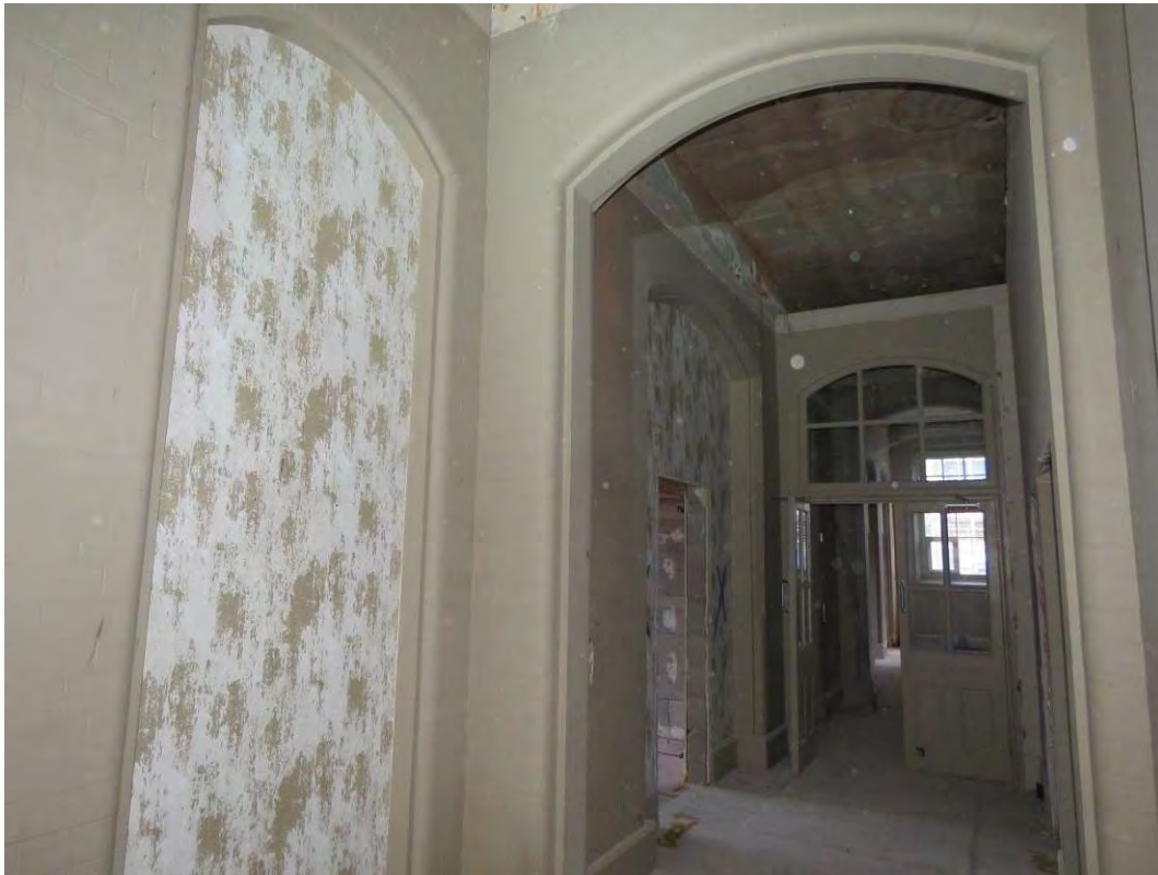
Figure 118: Looking west across S11, which formed the original boys' corridor. The arched openings to the left originally formed door and window openings into the adjacent classrooms. To the right can be seen an original pair of glazed timber corridor doors and fanlight which have been removed from their original location and repositioned. The doors and fanlight will be retained and redecorated as part of the consented scheme. The original glazed brick/exposed red brick will have its modern paint layers removed as part of the consented scheme.
