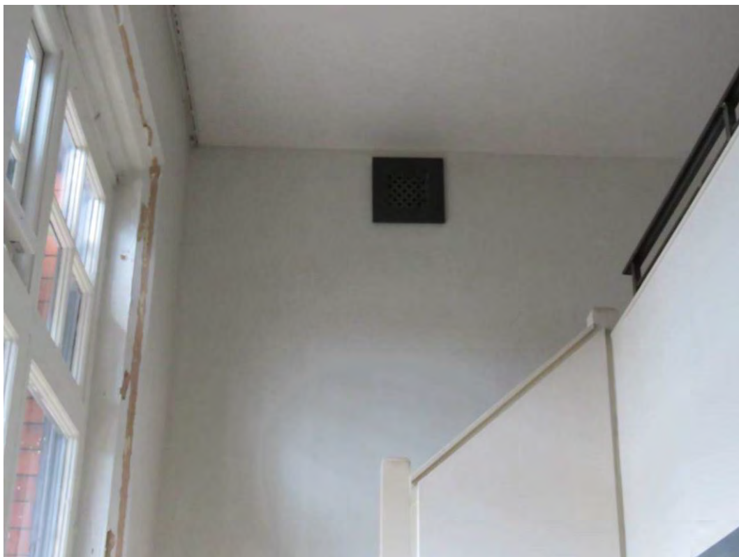
Figure 113: An example of an original/early metal ventilation grill to the south-west corner of S1, which will be retained and redecorated as part of the consented scheme
