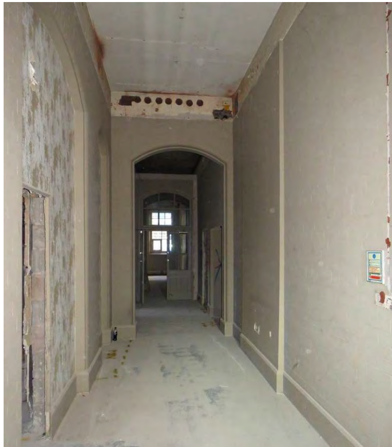
Figure 117: Looking west along S11, which formed the original boys' corridor. The original glazed brick/exposed red brick will have its modern paint layers removed as part of the consented scheme.
