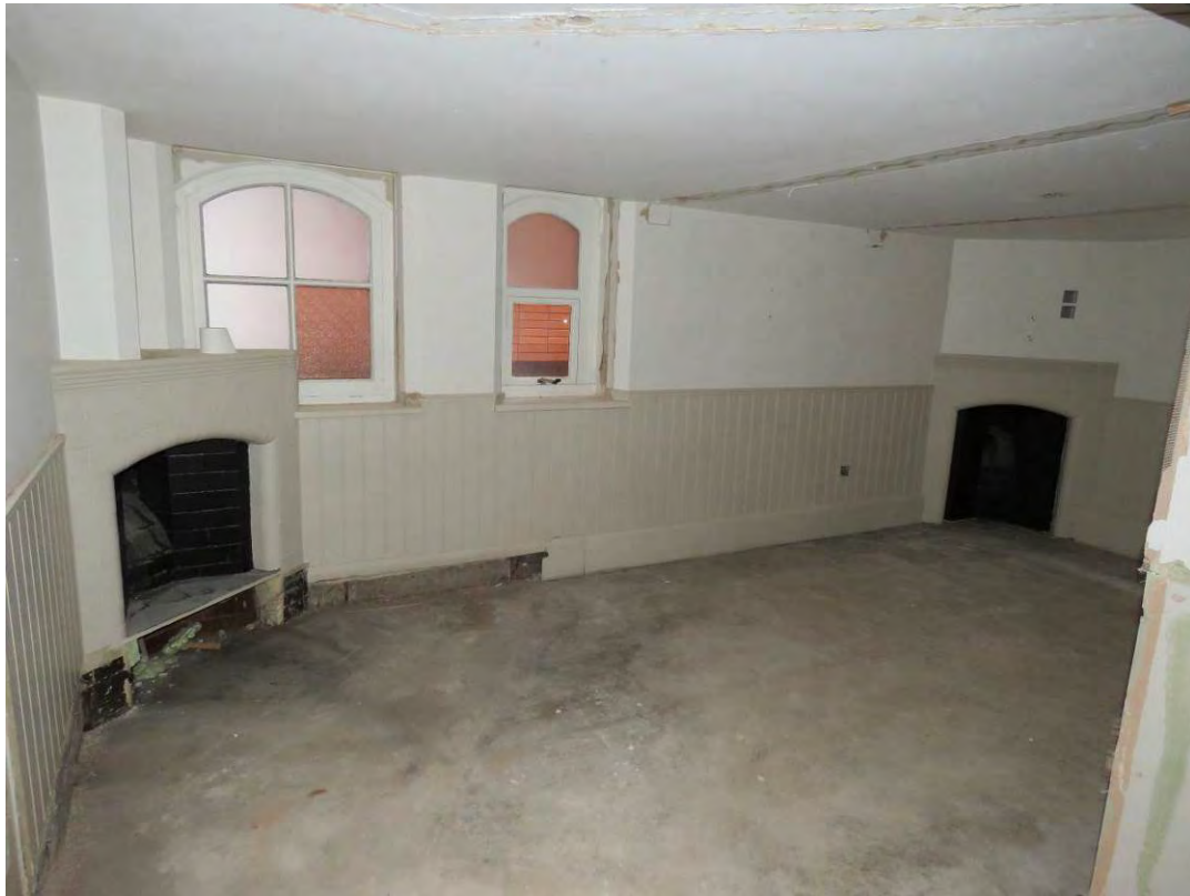
Figure 108: Looking north-east into FM15, which originally formed two teacher's offices. The original glazed brick fireplaces will be retained and redecorated as part of the consented scheme.
