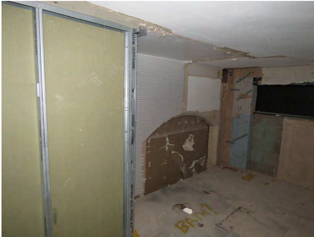
Figure 132: Looking north-east across SM5 towards the blocked upper part of an original internal window. The arch will be re-covered as part of the consented scheme.
