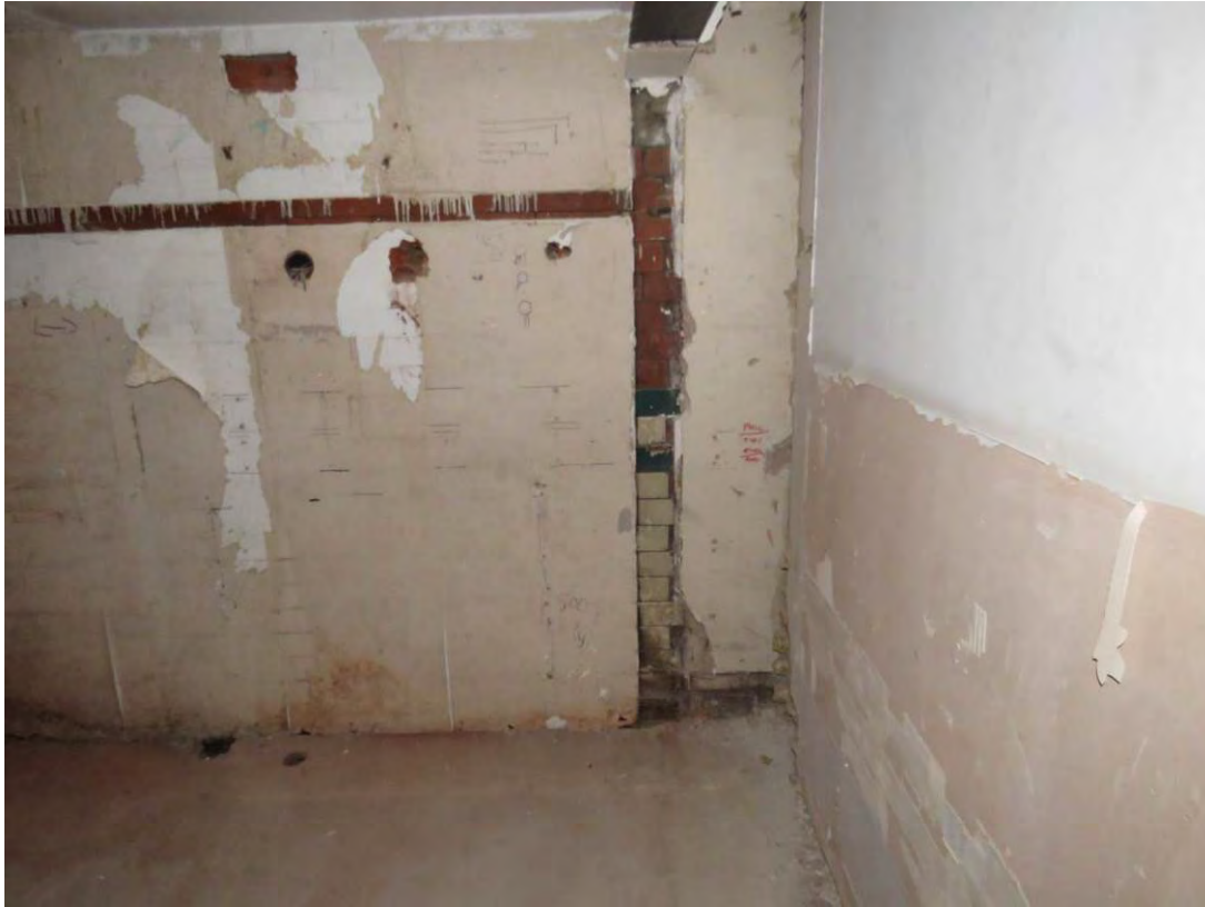
Figure 110: Looking west into the former en-suite from room FM14, showing the location of the original glazed partition dividing the teacher's office (right) and access corridor (left). This photo illustrates that originally the upper parts of the walls were exposed brick, whilst the lower part was glazed brick. The horizontal area of exposed brick (left) is likely to have originally been a timber coat rail at the end of the access corridor. The walls will be re-covered as part of the consented scheme.
