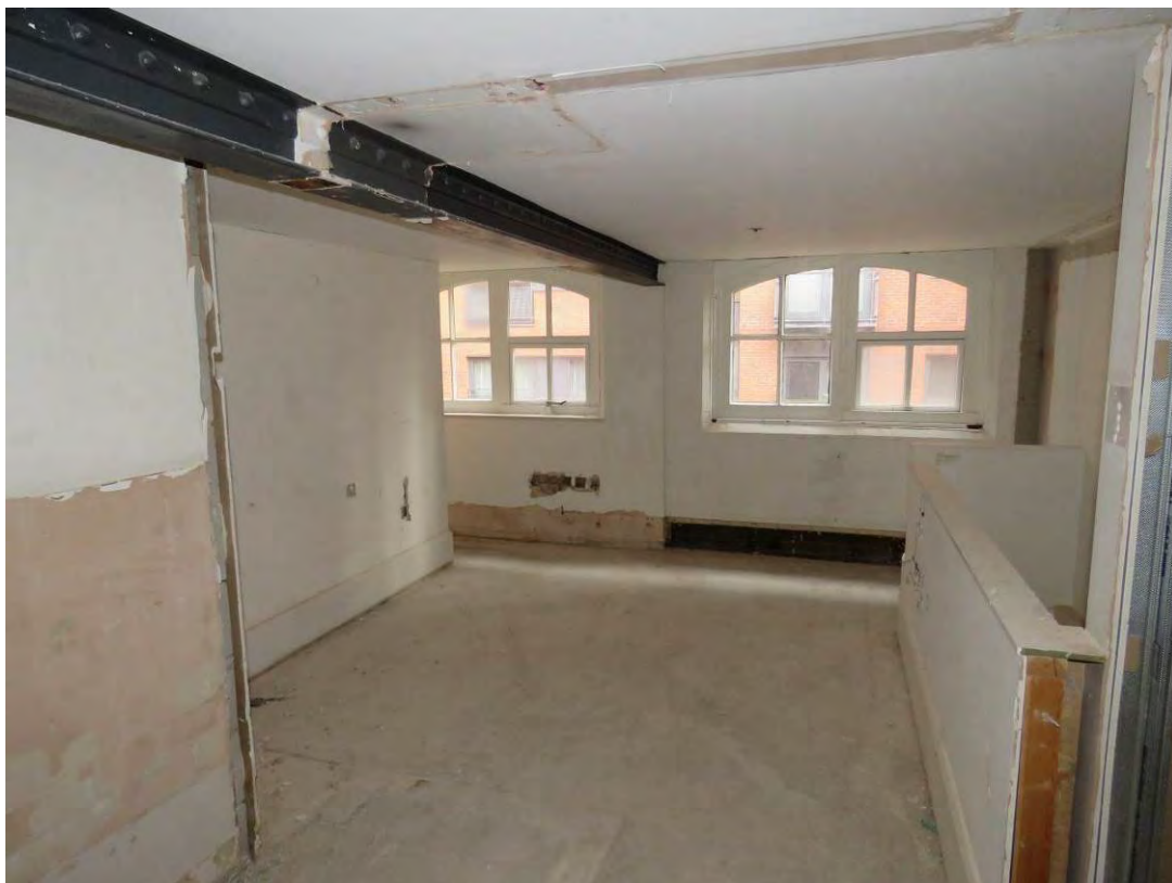
Figure 109: Looking east across FM14 towards the original mezzanine corridor window (left) and original teacher's office window (left).
