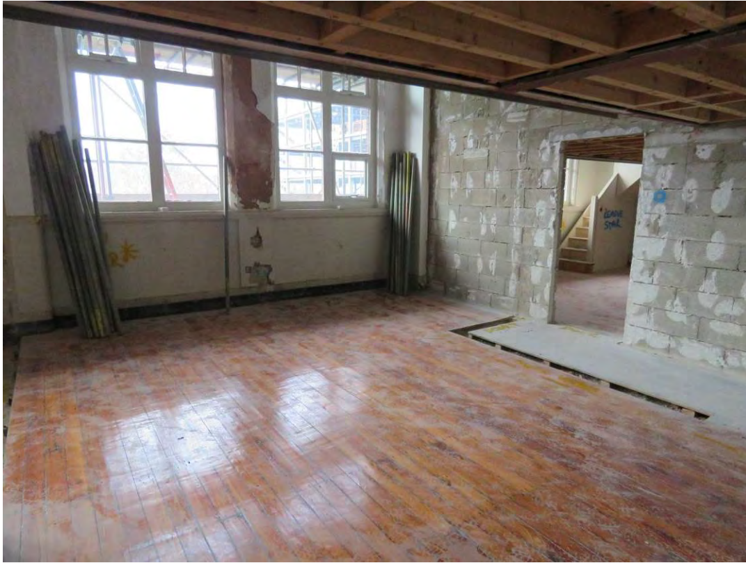
Figure 114: Looking south-west across S4 showing an original example of timber floorboards, which will be covered with new timber floor as part of the consented scheme.
