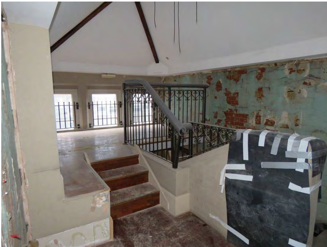
Figure 137: Looking east into the original boys' staircase (T2), showing the modern inserted upper level and steps.
