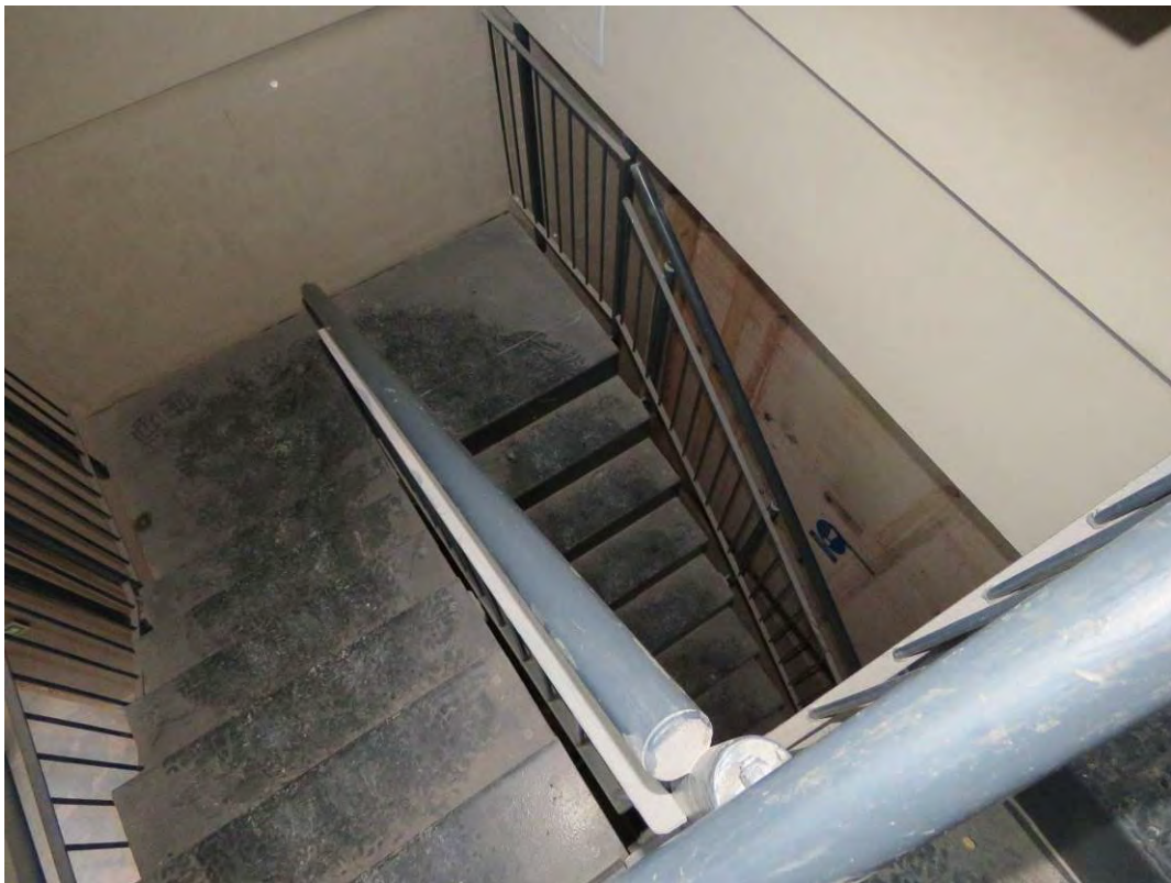
Figure 139: Looking down into the modern 2004 roof access stairs extension (T4) the original girls' staircase.
