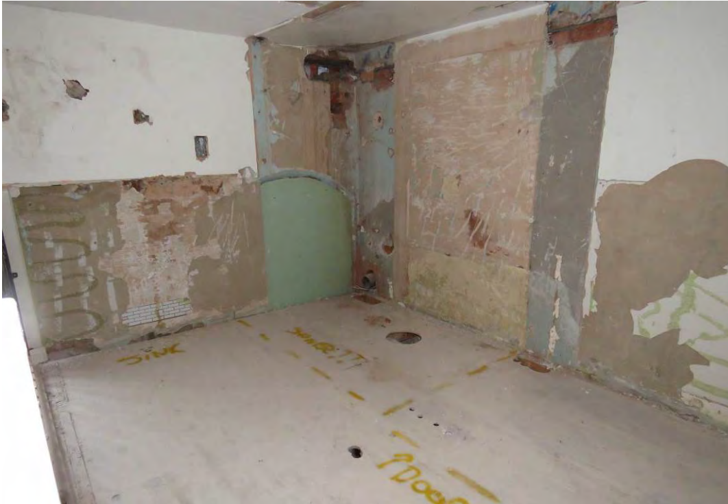
Figure 128: Looking north-east across SM2, which forms the upper part of the original second floor boys' classroom below. The blocked archway forms the upper part of the original classroom entrance door. The arch will be re-covered as part of the consented scheme.
