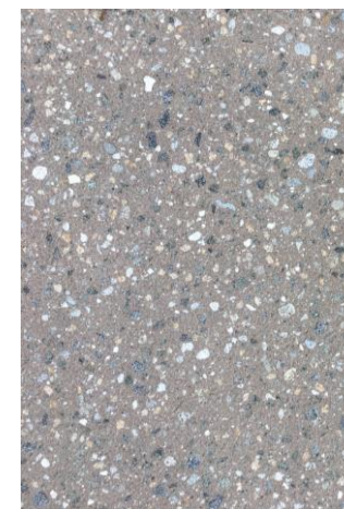
In-Situ Concrete with seeded exposed aggregate
