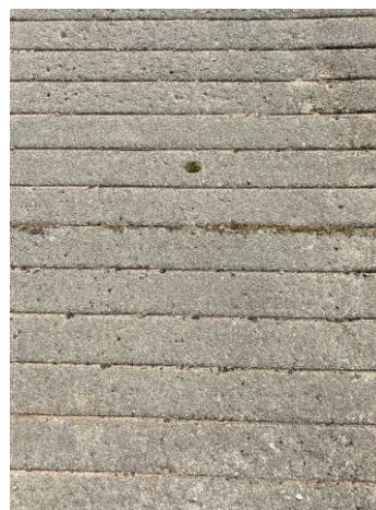
On site example of combed finish
