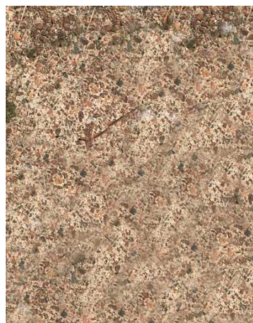
On site inspiration of In-Situ Concrete with seeded exposed aggregate
