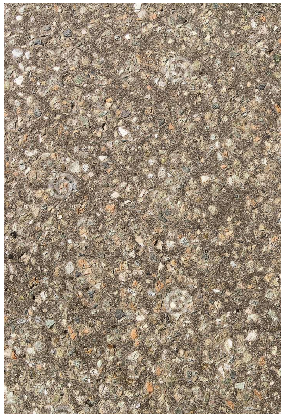
Temporary asphalt with precoated aggregate (detail view)
