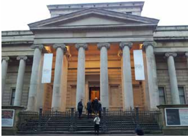
Manchester Art Gallery with banners suspended from the pediment to its portico façade, and ratcheted around the columns
