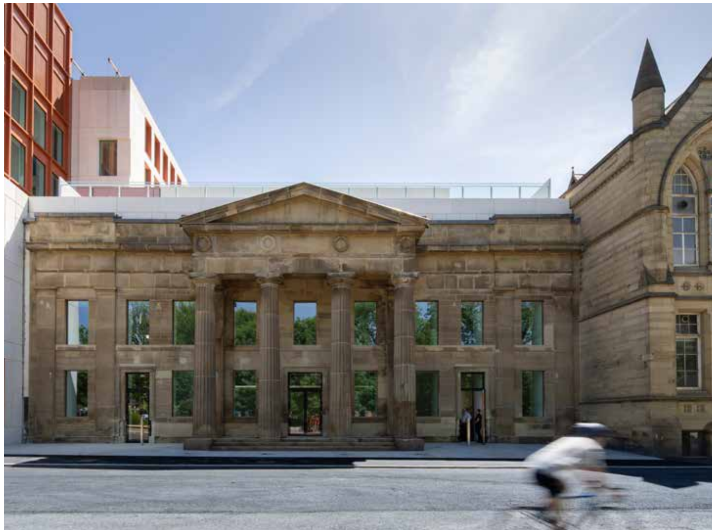
Photo of the Portico façade following its restoration as part of the complete new Arts and Humanities development Building
