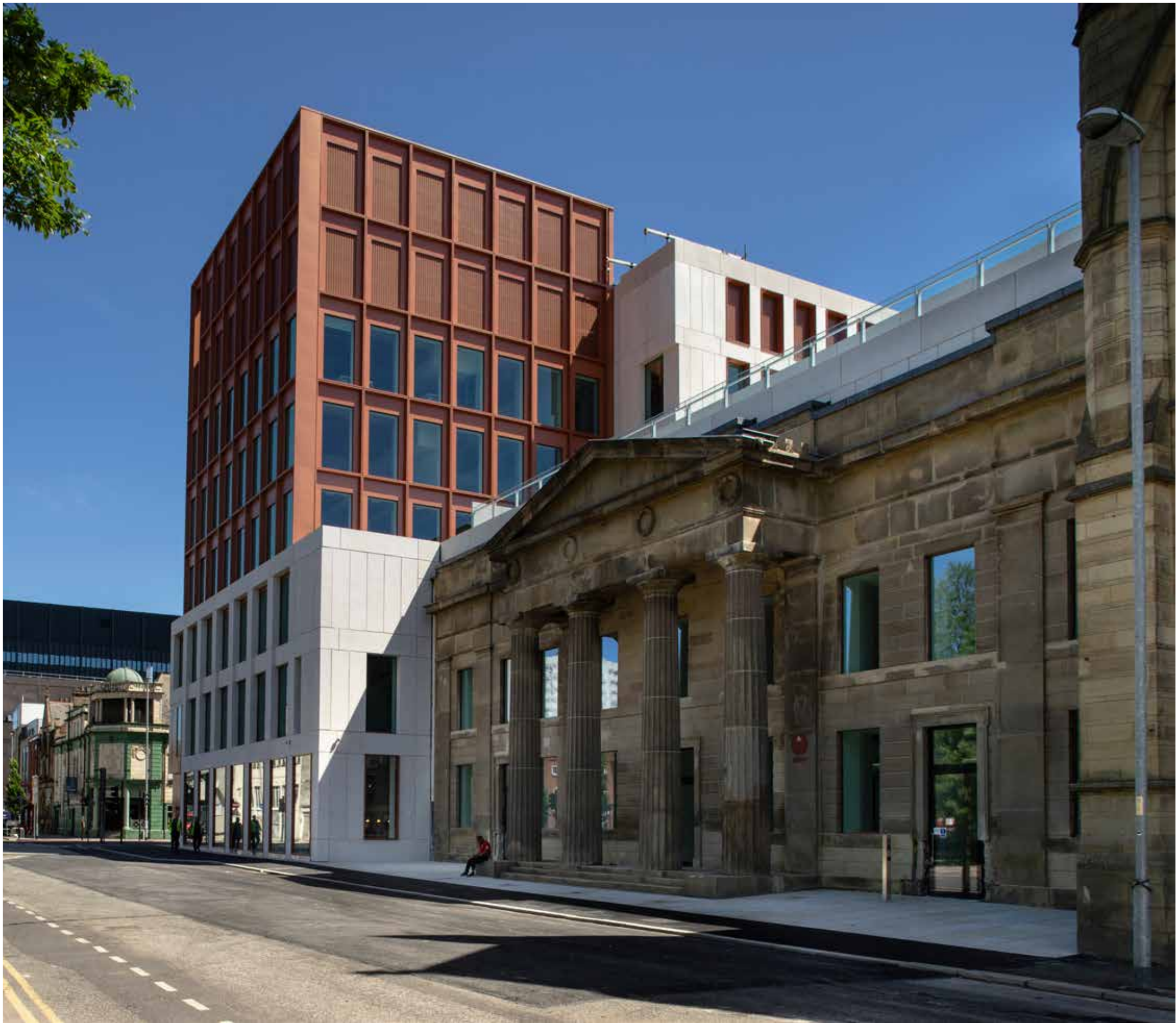
Photo of the restored portico façade frontage to the new Arts & Humanities
