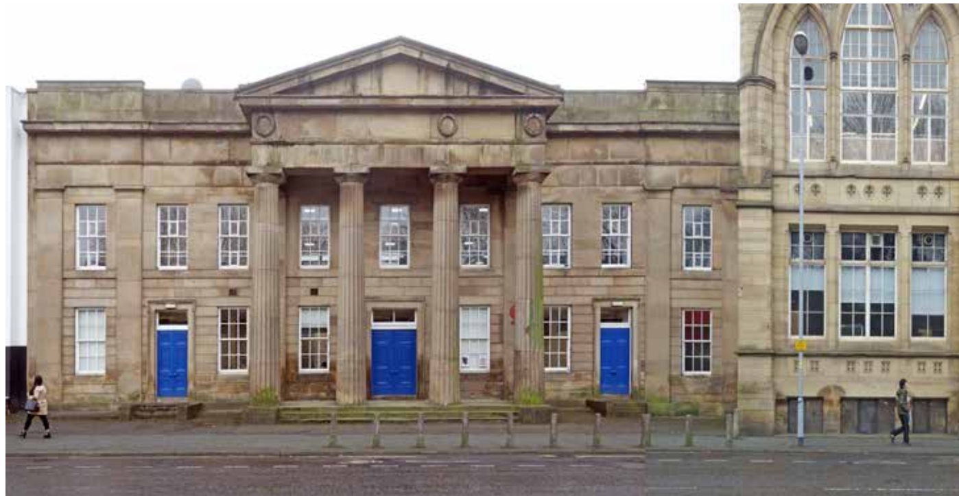
Photo of the Portico façade prior to the demolition of the 1970's Mabel Tylecote building and restoration of the listed building
