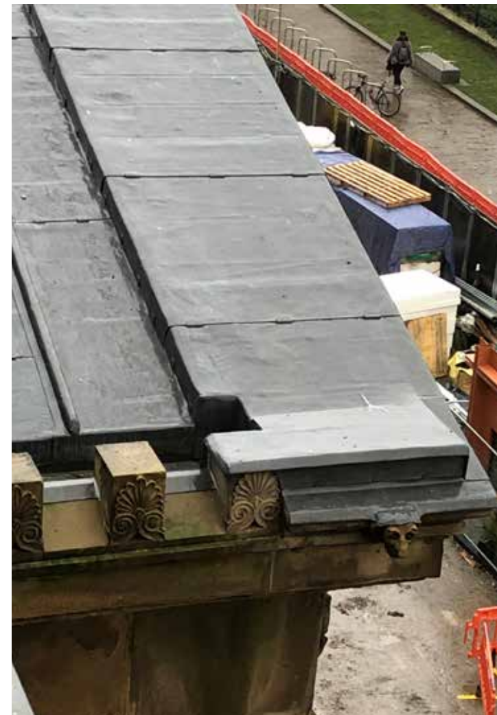
Detail photo of new lead roof and weatherings
