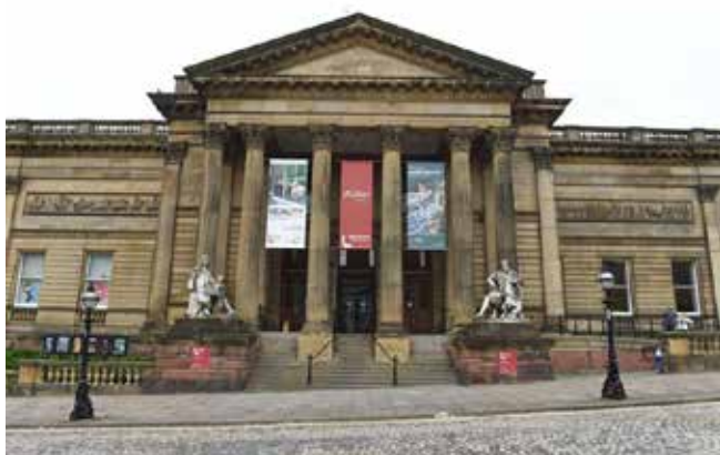
Walker Art Gallery with banners supported from horizontal rails supported in between the columns on its portico façade supported in between the columns on its portico façade
