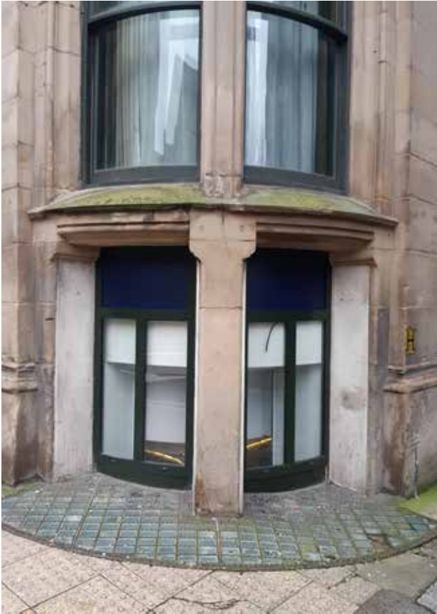
3.18a Basement lightwell infilled with pavement lights
