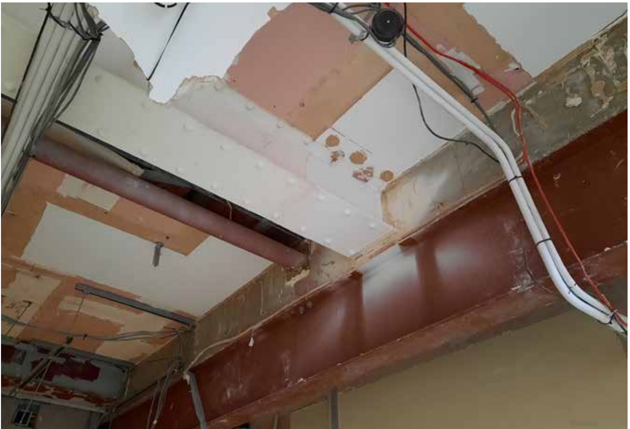
3.29c Opening works at first floor revealing modern beam intersecting original riveted beam
