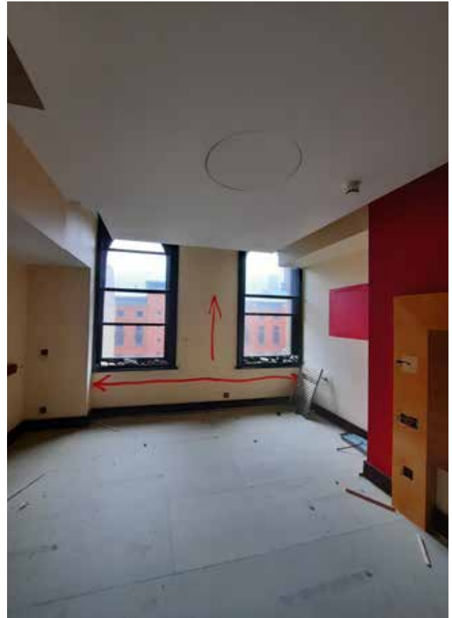
3.27 Typical 3 rd floor room
