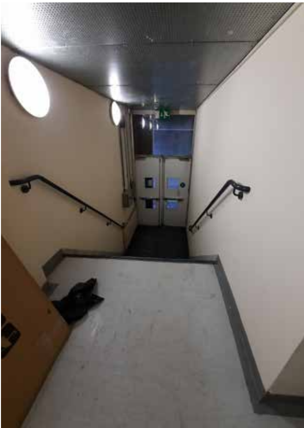
3.22c Rear modern staircase exiting on to Back George Street and serving all floors
