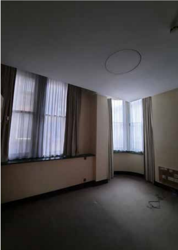
3.25a Ground floor room with lowered ceiling
