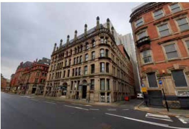
3.2 18-24 Princess Street with group of warehouses lining south side of Princess Street
