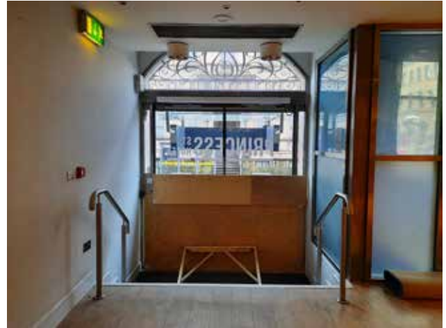
3.23a Modern central entrance
