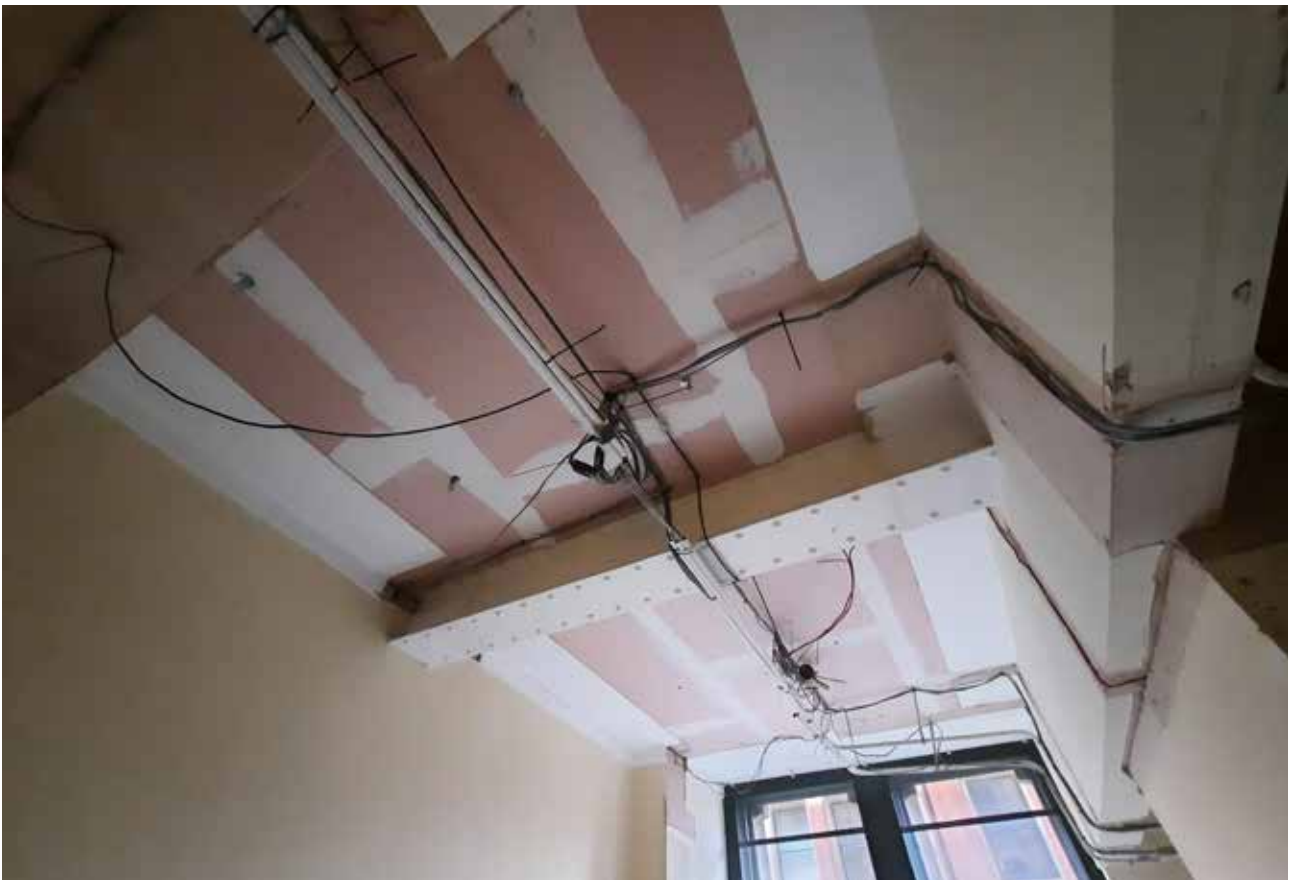
3.30b Opening up works to first floor room revealing original cast iron beam and rivets, modern beam remains encased
