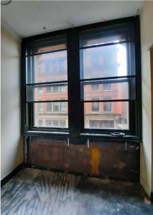
3.30a Opening up works to first floor room revealing original brickwork
