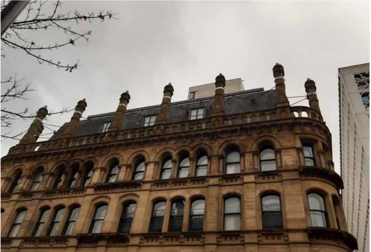
3.21a Two storey mansard and recessed third roof storey behind
