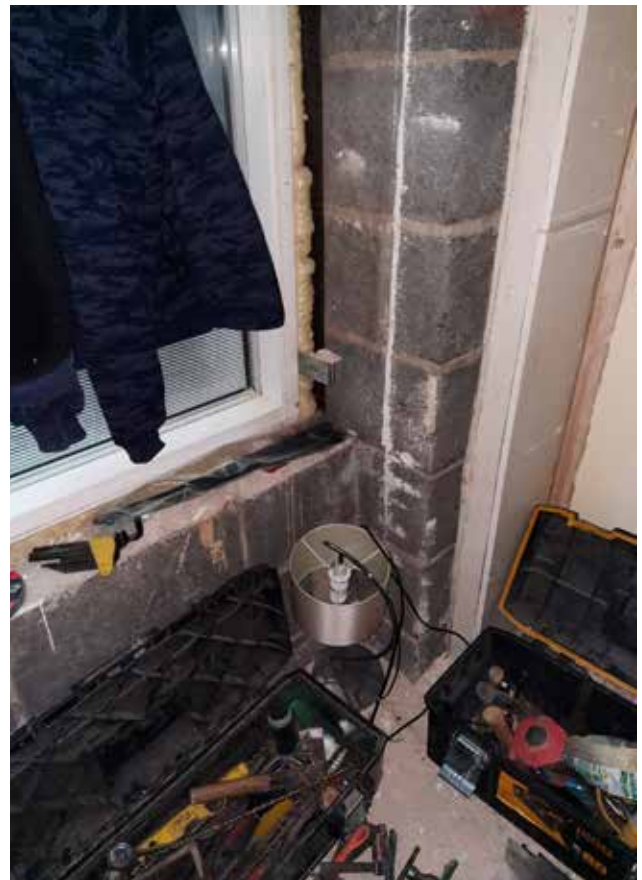
3.32b Opening up works revealing blockwork to modern infill
