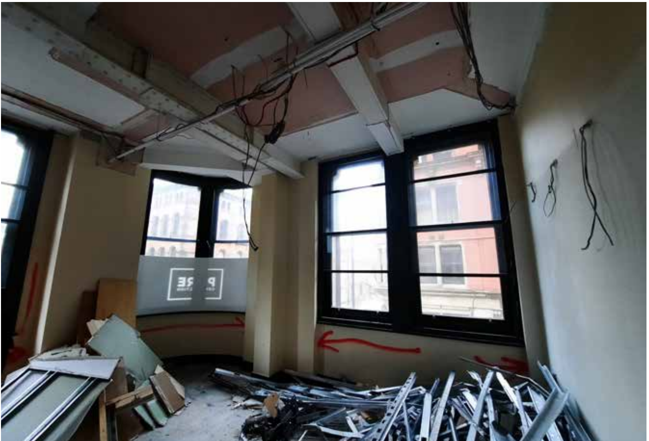
3.31 Opening up works to front first floor room revealing original cast iron beams and rivets
