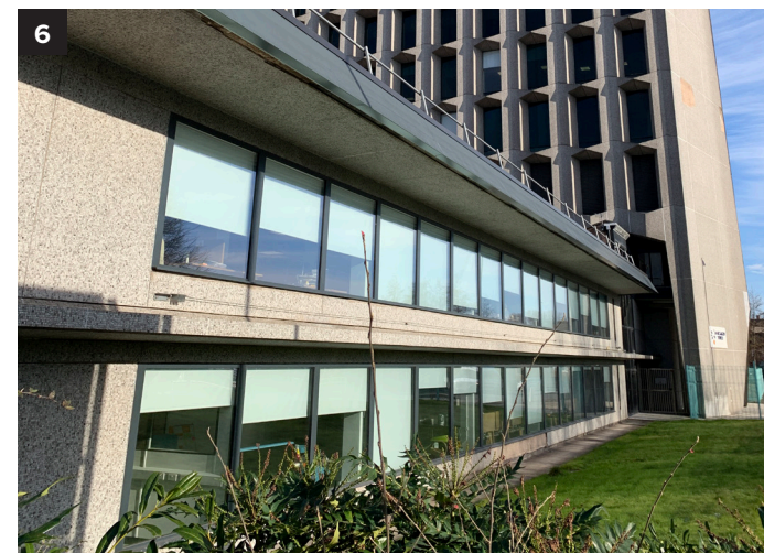
View looking east along Crumps Vale
