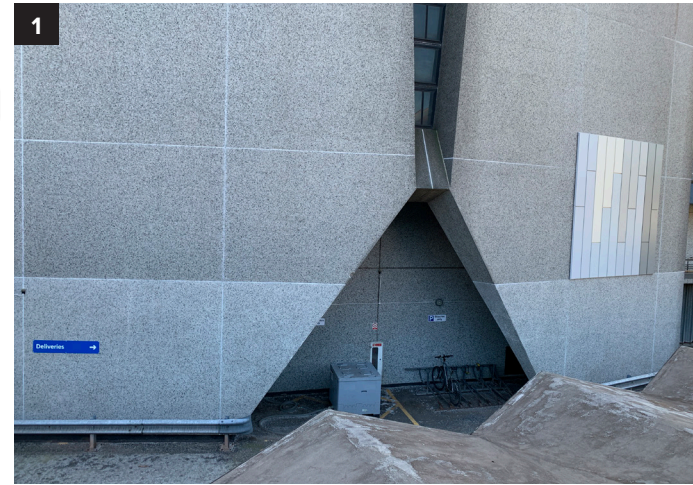
Ground level of Tower on North elevation
