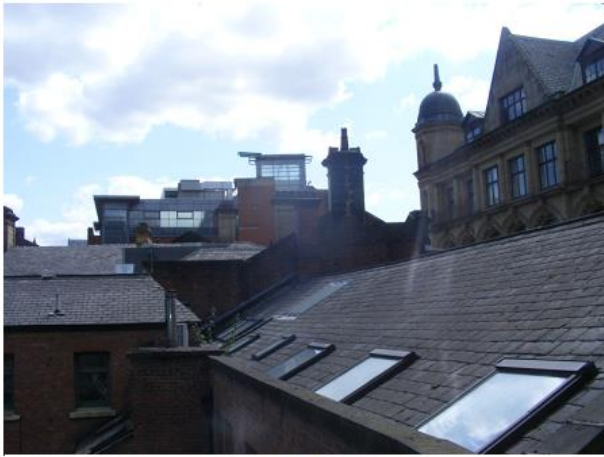
PHOTO 7 Western View Along Roofline
