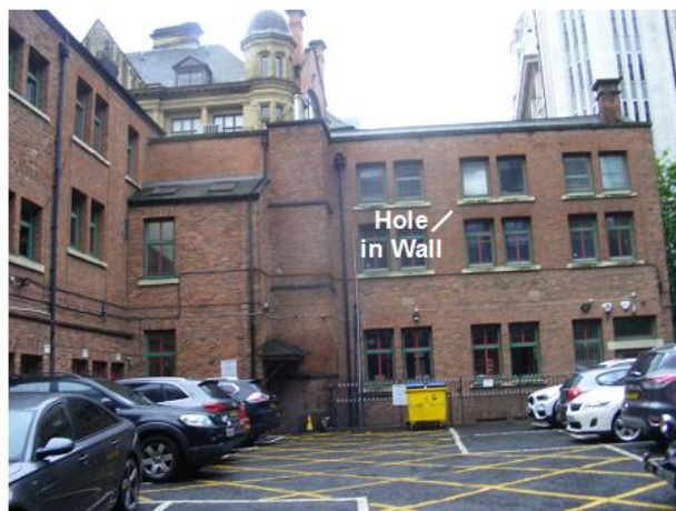
PHOTO 4 Northern Elevation of Main Building
