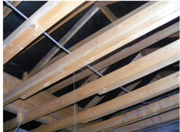
PHOTO 12 Underside of Second Building Roof
