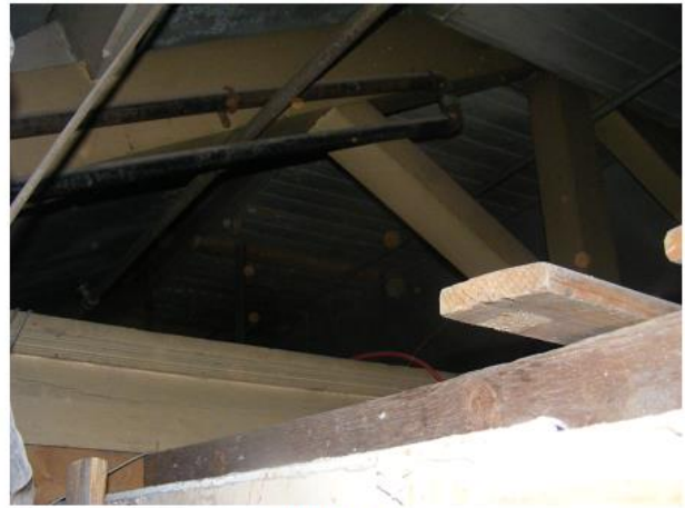
PHOTO 8 Underside of Main Building Roof
