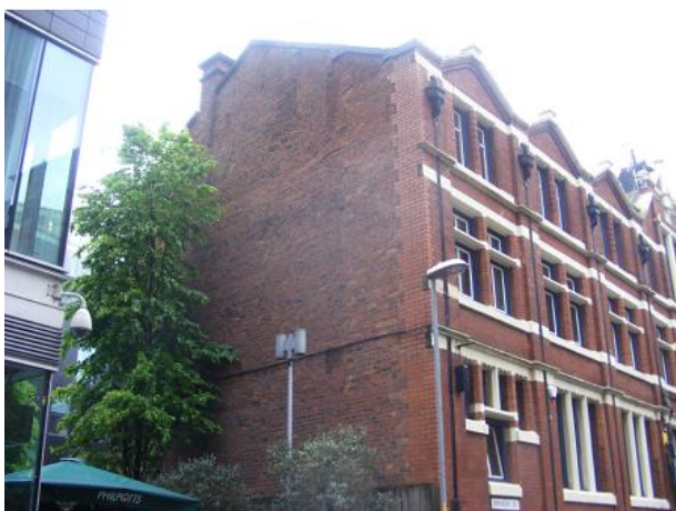
PHOTO 3 Western Elevation of Main Building
