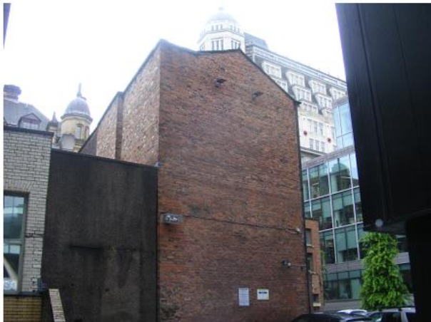
PHOTO 11 Northern Elevation of Second Building
