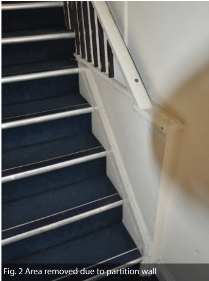
Fig. 3 Handrail, balustrade and stringer
