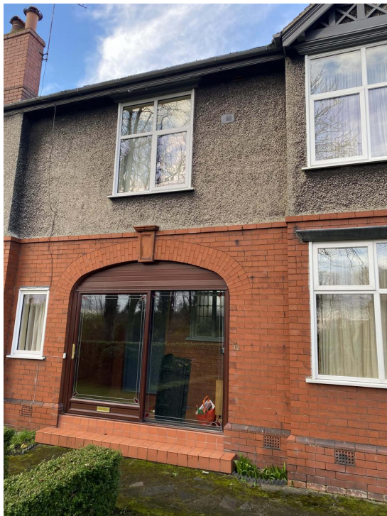
Front porch showing original arch and existing glazed uPVC porch door to be replaced and existing oriel windows to the first floor.
