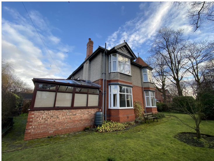
Existing uPVC conservatory to be replaced
