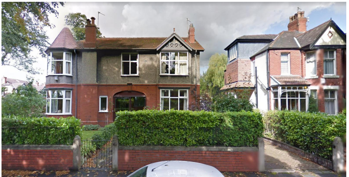
The existing front elevation showing the existing boundary wall, gate posts and gates and driveway.
