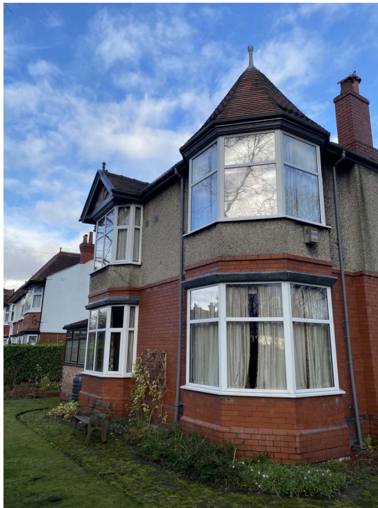
The side elevation showing the turret, bay windows and brick plinth and band detailing
