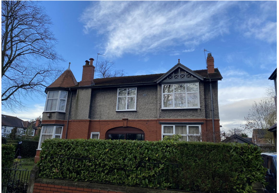
The existing front elevation of the house showing the turret, brick entrance arch, timber detailing and pebbledash render.
