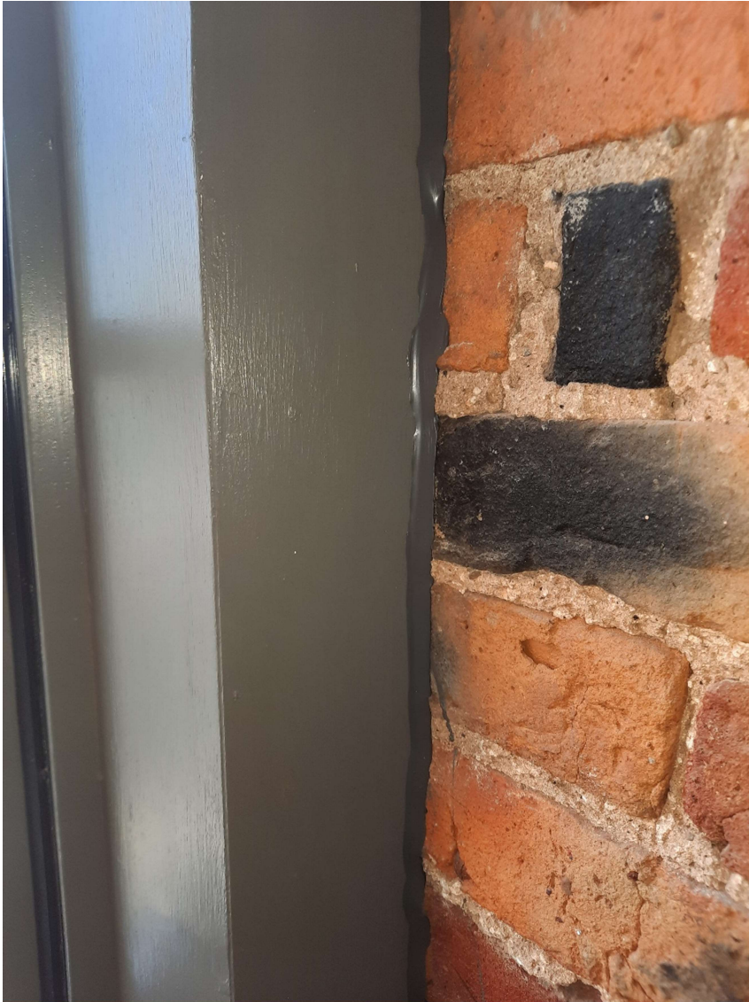
Figure 9 Window reveal painted and sealant applied internal
