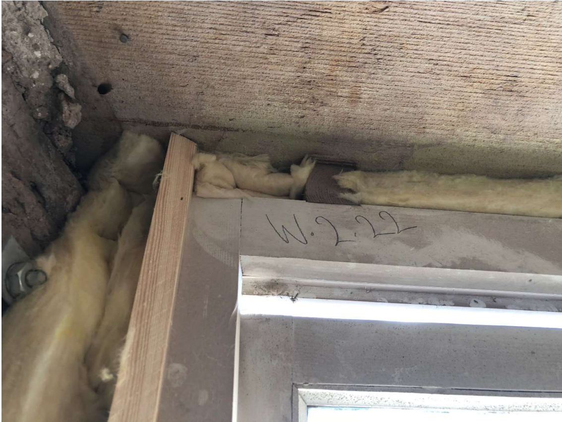
Figure 7 Internal window reveals pre-boarded
