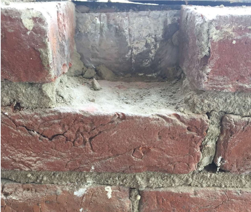
Figure 8 Internal cill repairs
