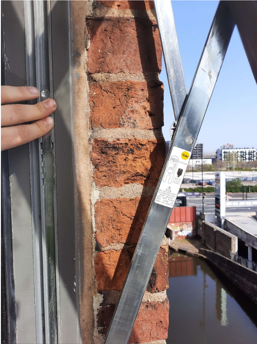
Figure 3 Example of new hinge installed and Burnt Sand Mastic
