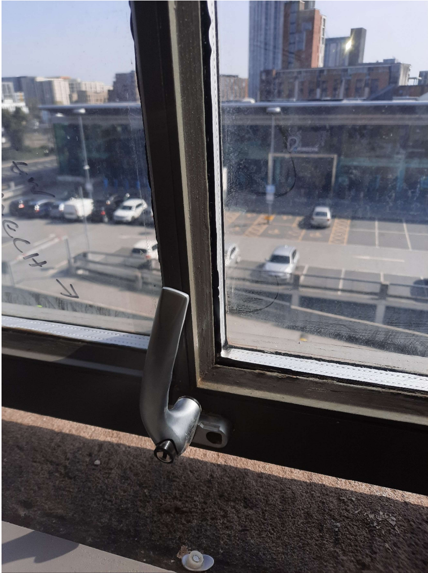
Figure 4 Example of new window handle installed to match existing
