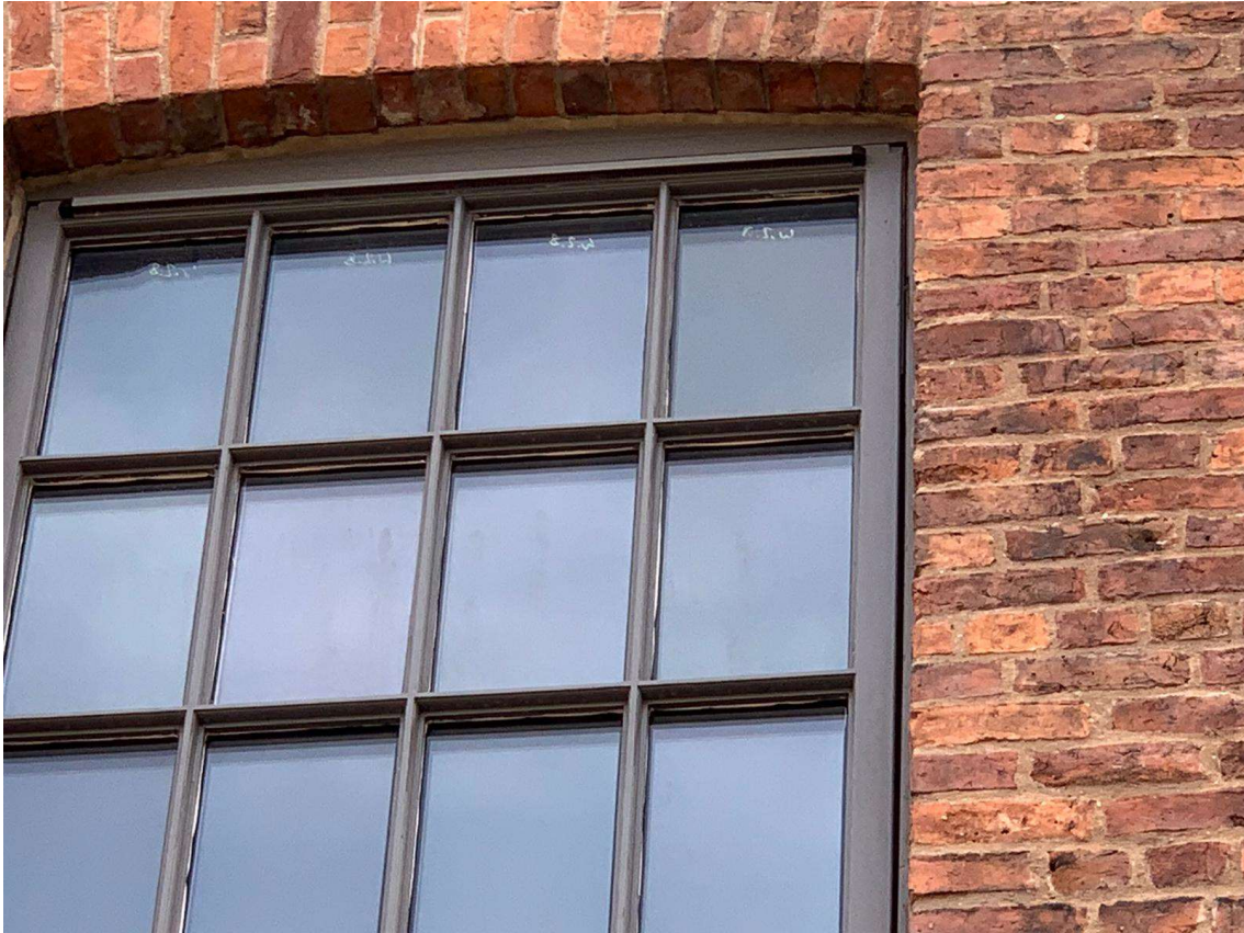
Figure 5 Example of window with trickle vent installed, windows repairs carried out, new glazing and painting.
