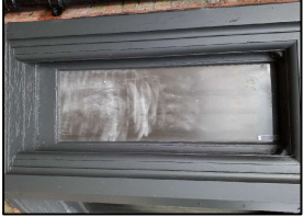
P47b - View of External Bay Window to A037
