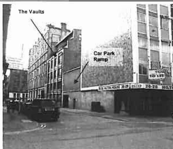
Photo 3: Looking down Tariff Street to car park ramp and 'The Vaults' apartments
