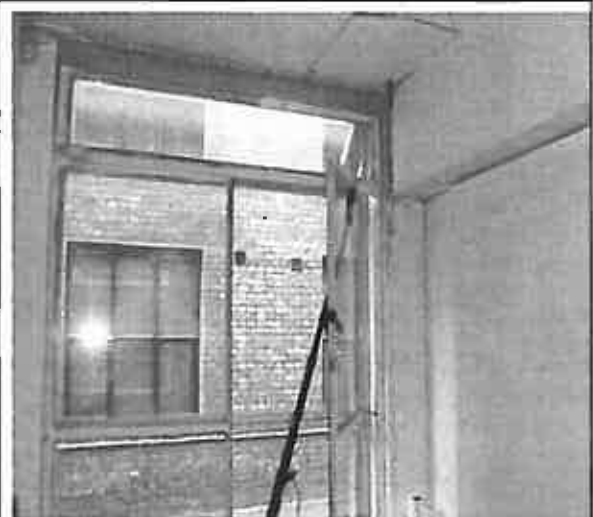
Photo 4: Looking from Hilton House ground floor west façade window across to The Vaults apartments.
