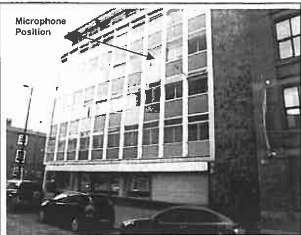
Photo 2: Looking to Port Street façade of Hilton House, showing noise monitoring position
