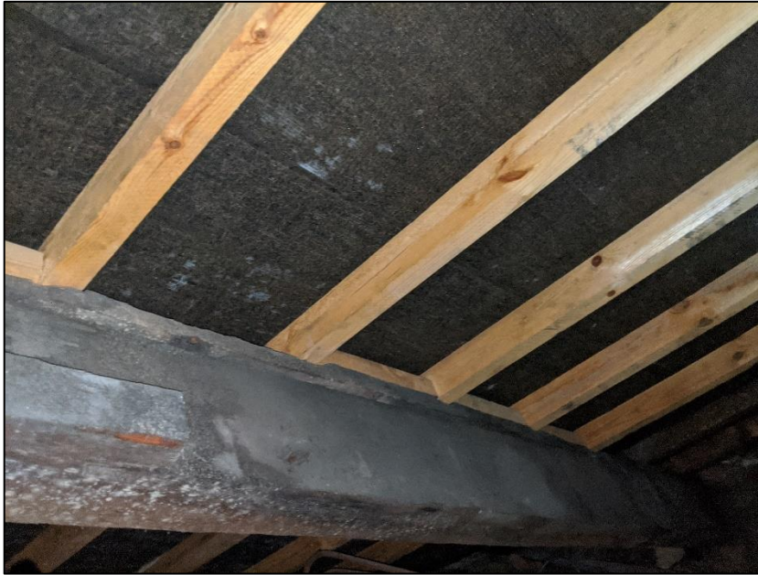
Photograph 6 showing the small, shallow roof void above the extension
