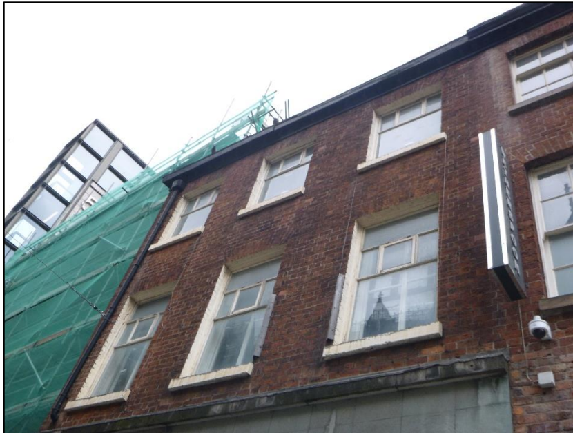
Photograph 1 showing the front elevation of the property
