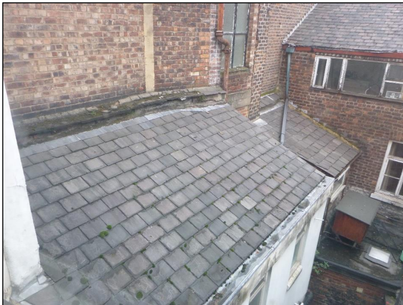
Photograph 3 showing the roof of the rear extension
