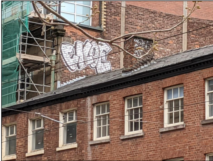
Photograph 2 showing the roof of the property
