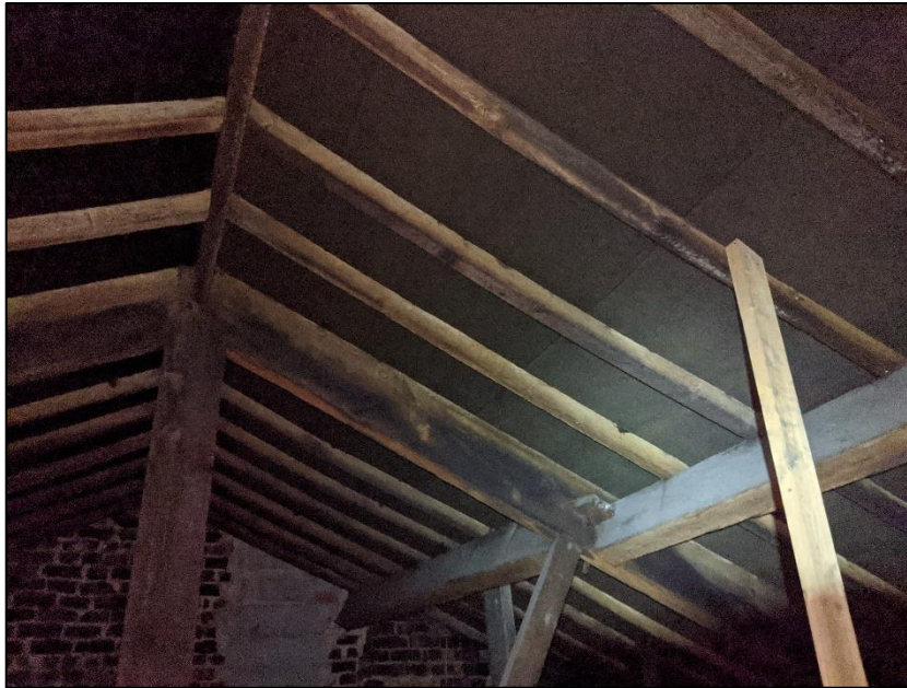
Photograph 4 showing the roof structure of the upper floor
