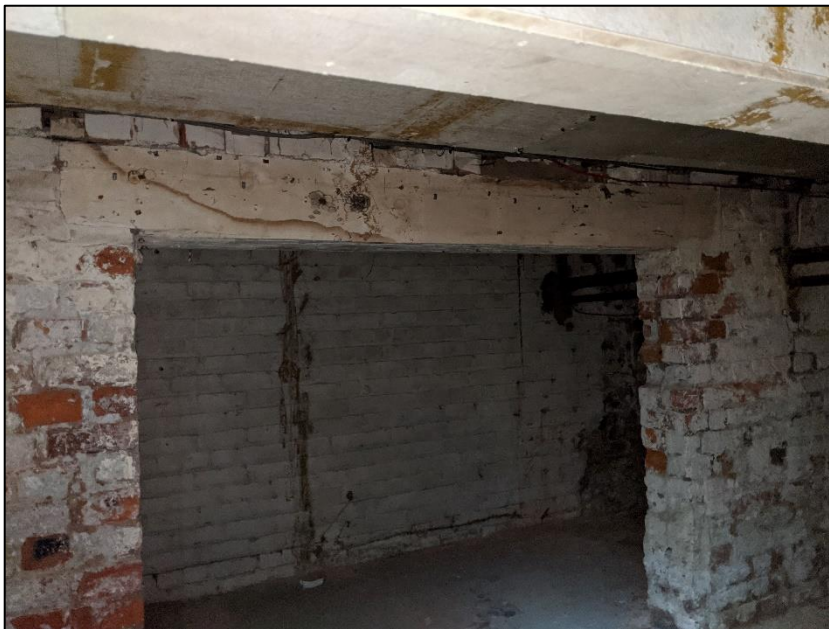
Photograph 7 showing the cellar space
