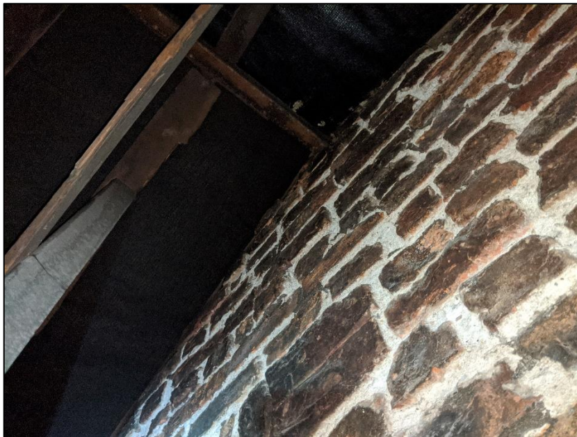
Photograph 5 showing the internal brickwork
