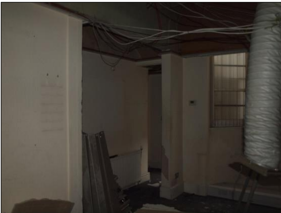
Plate 23: Northern end of ground floor showing passage to northwest extension
