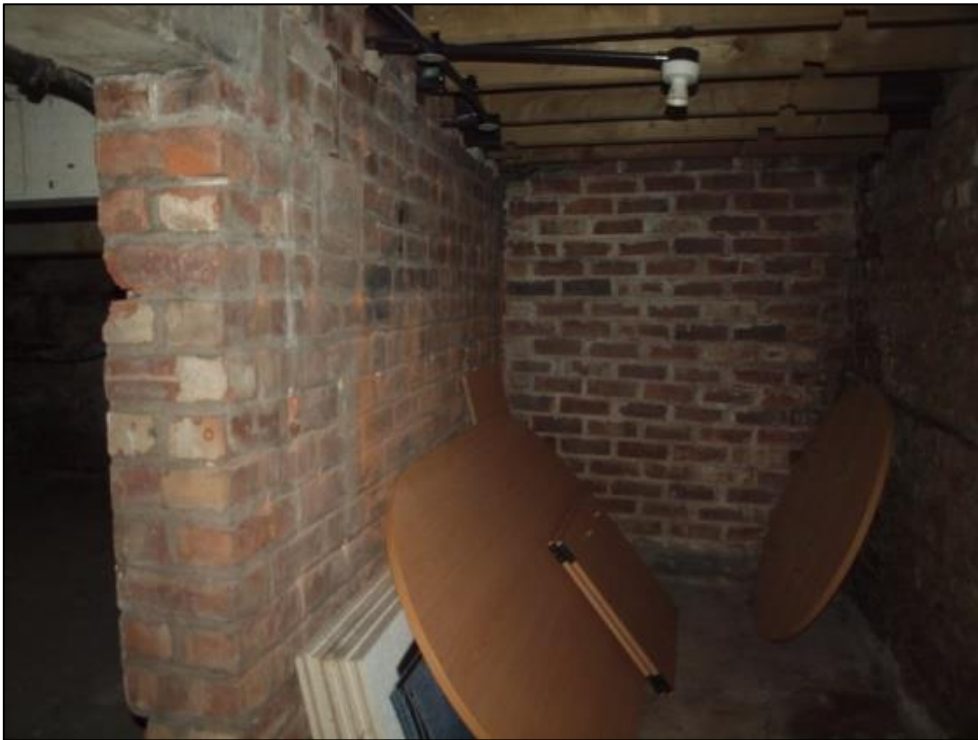
Plate 76: Southern end of basement showing inserted walls
