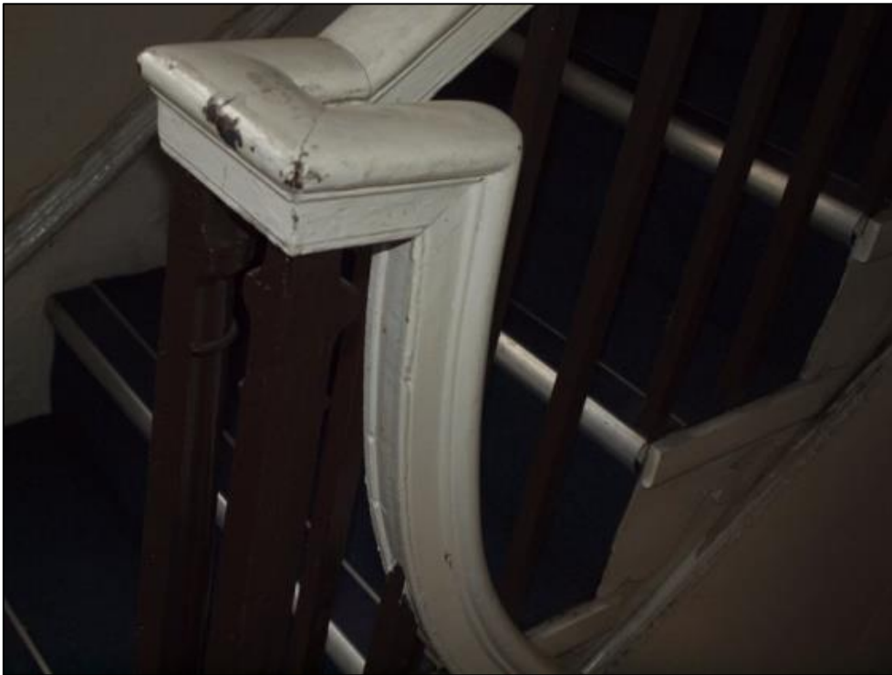
Plate 48: Detail of handrail
