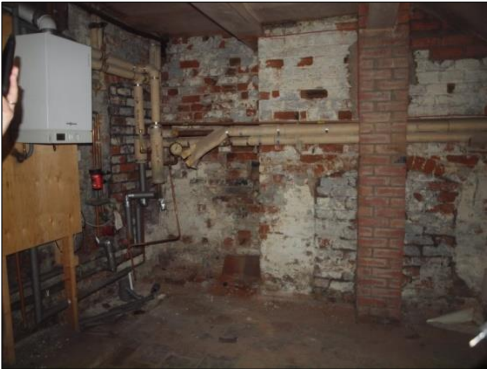
Plate 80: Eastern room of basement showing blocked fireplace
