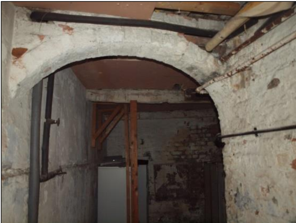
Plate 73: Brick arched entrance to northern room of basement
