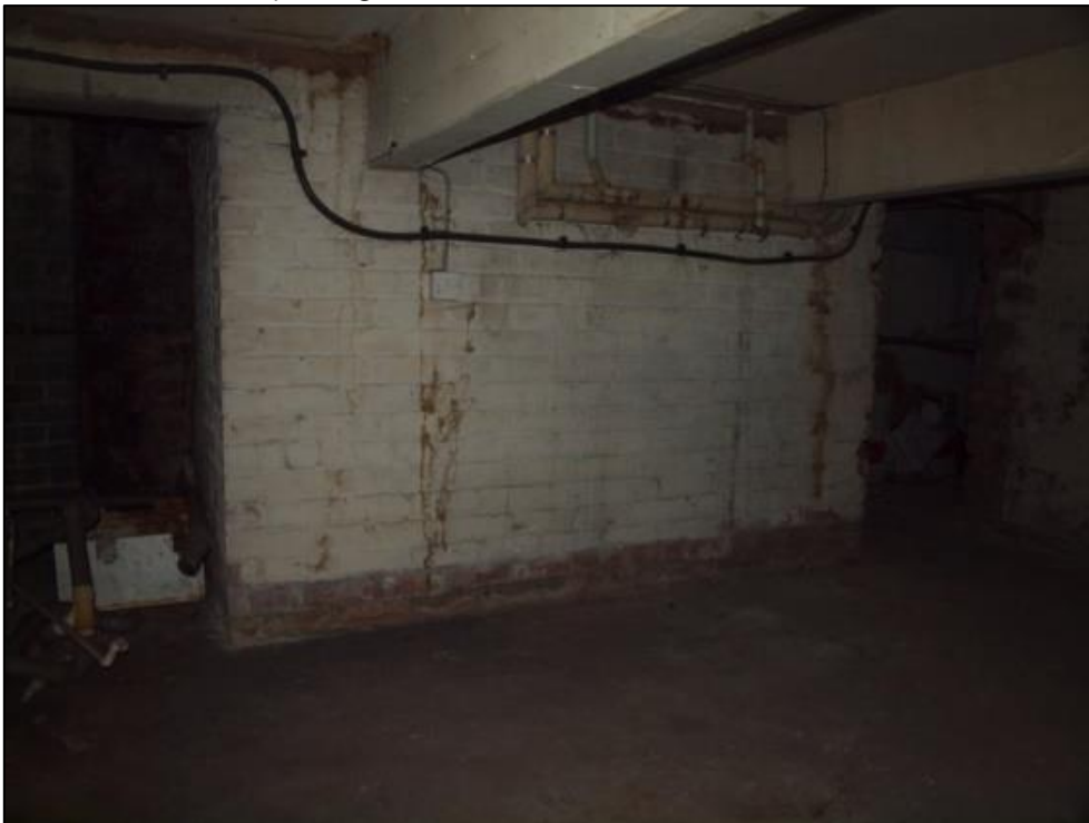
Plate 79: Southern room of basement
