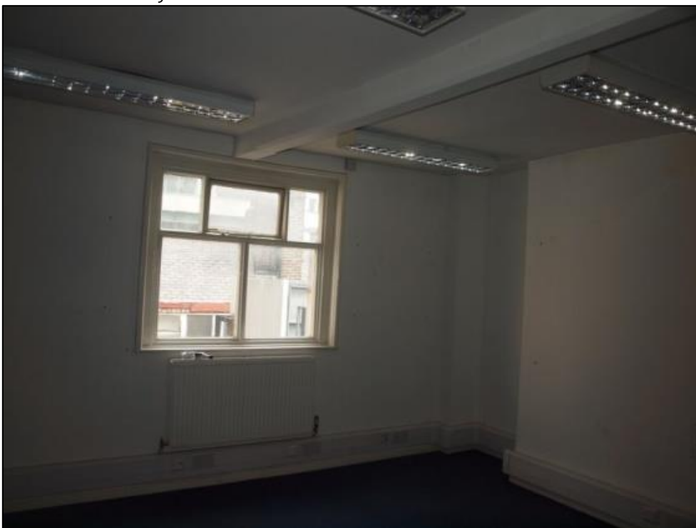
Plate 57: North room showing window
