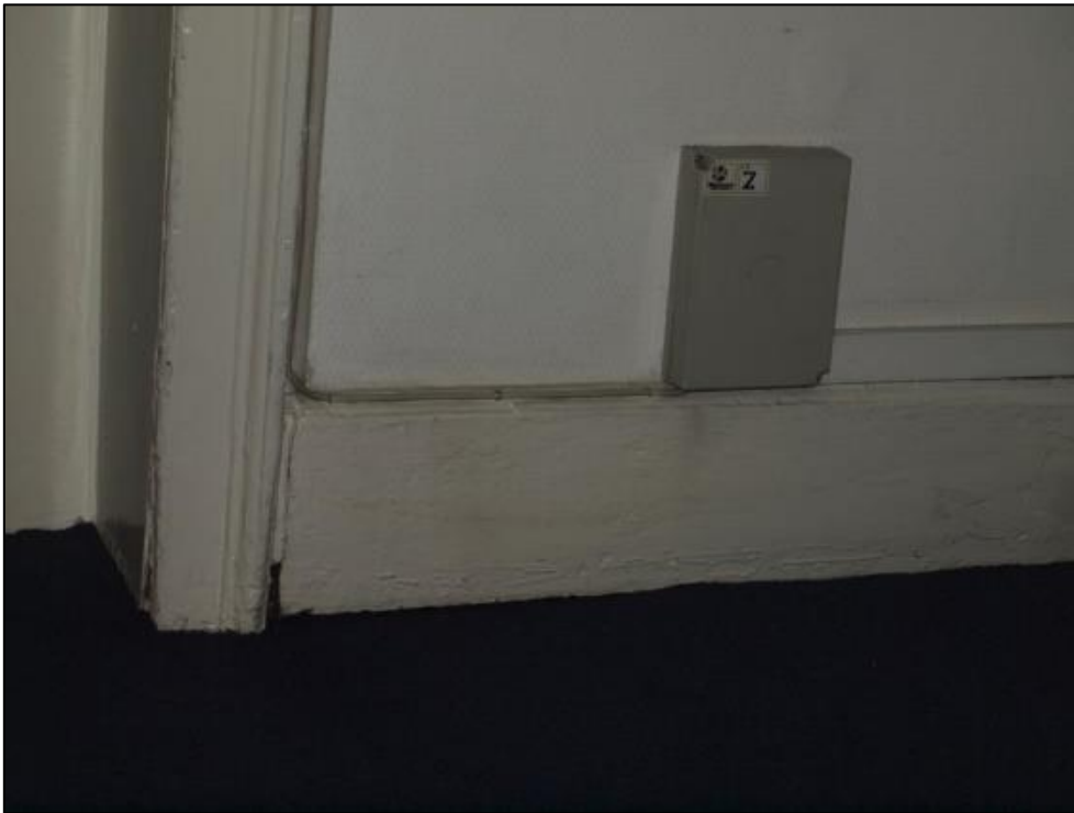
Plate 60: Skirting to west of doorway to south room
