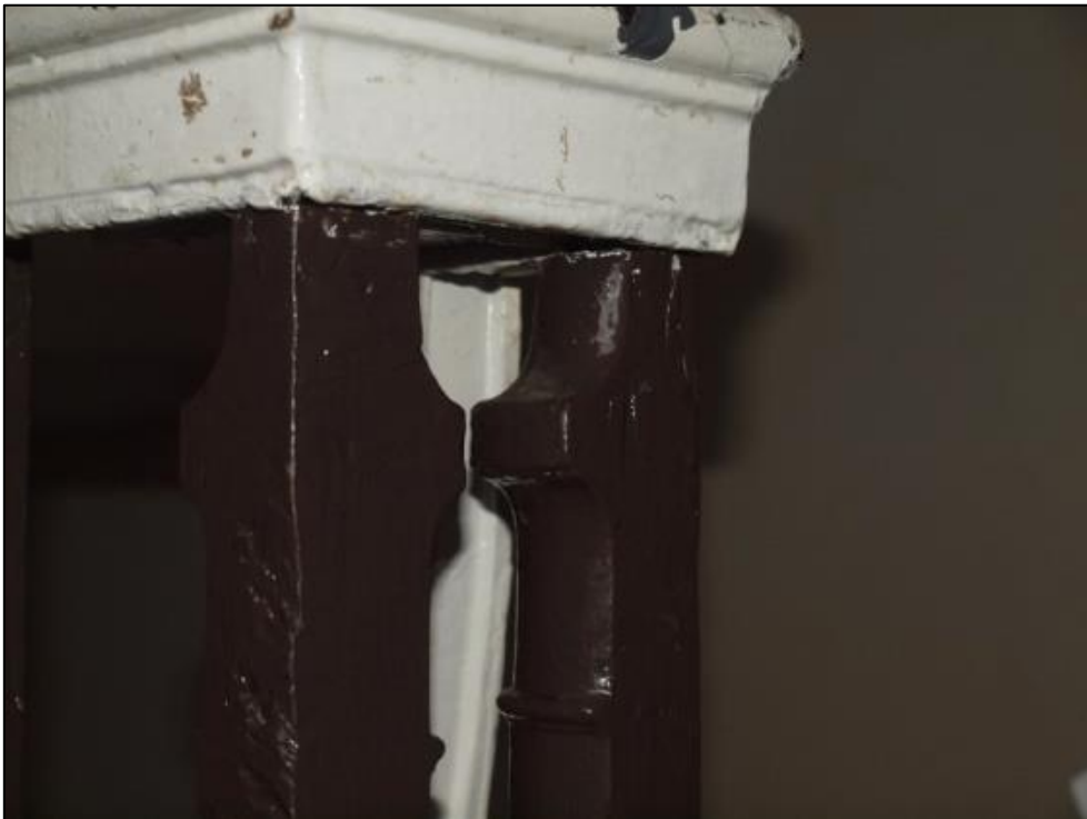
Plate 49: Detail of reused balusters
