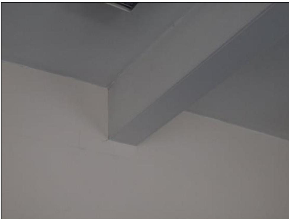
Plate 71: Modern timber beam in south room
