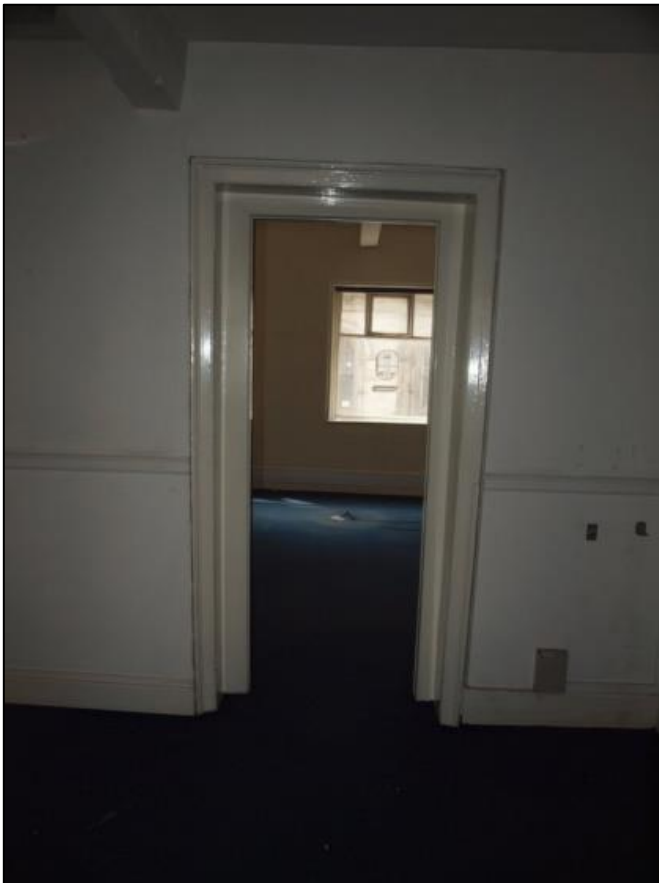
Plate 61: Moulded timber surround of doorway to south room
