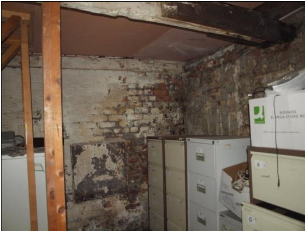
Plate 74: Northern room of basement
