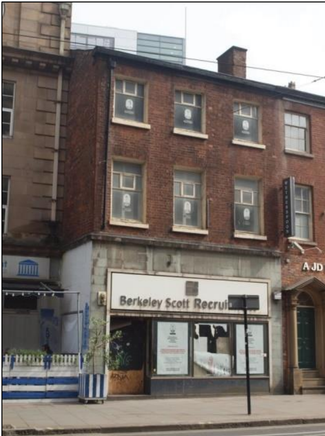
Plate 3: Detail of 65 Princess Street
