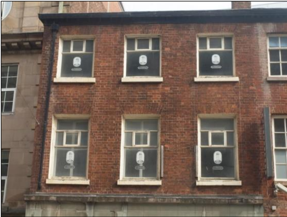
Plate 5: First and second floor windows
