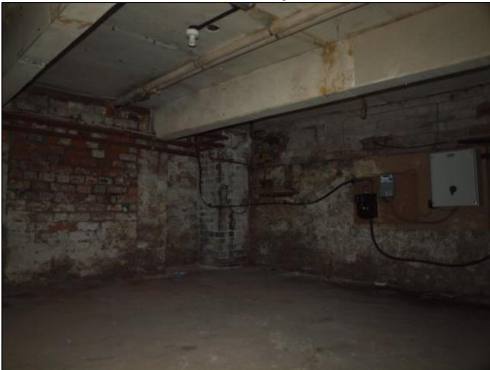
Plate 77: Southern room of basement showing low ceiling and modern timber beams
