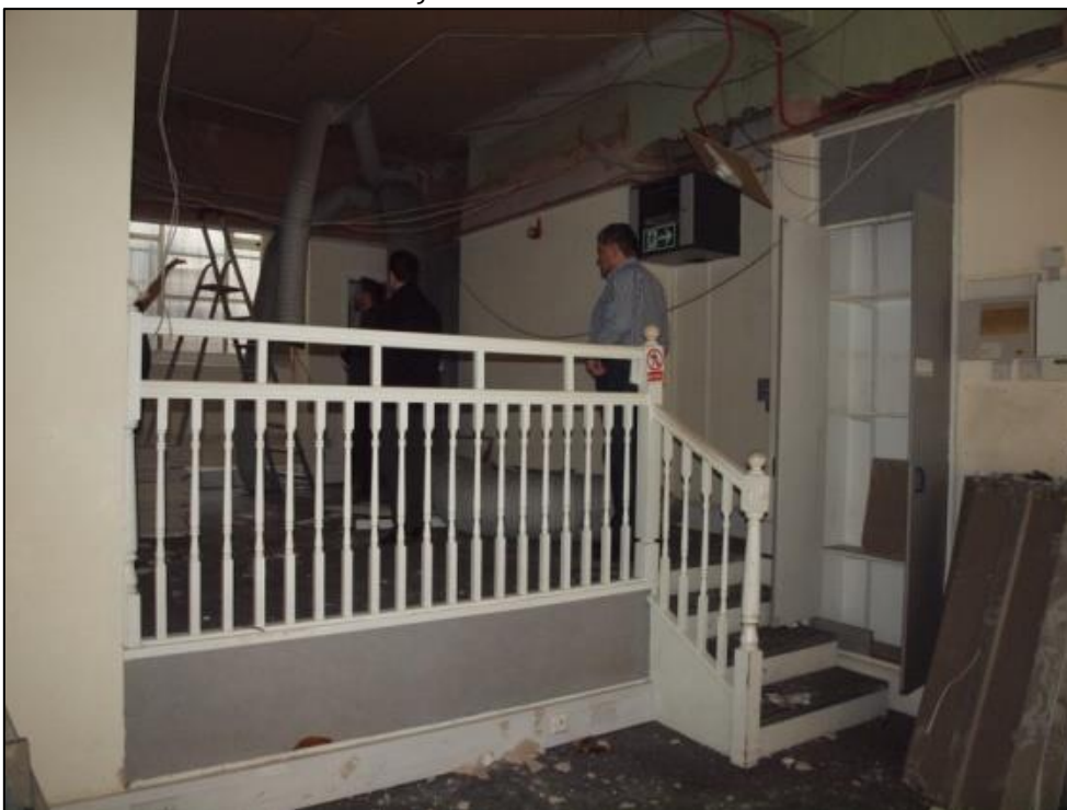
Plate 15: Southern end of ground floor showing raised area to north
