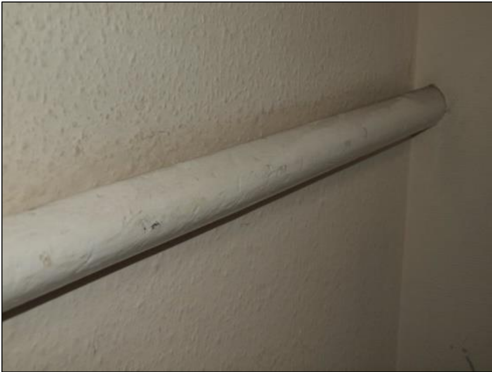
Plate 28: Simple timber handrail of staircase
