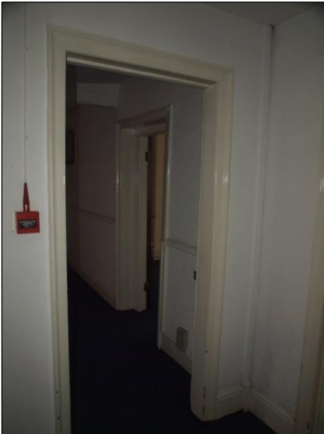
Plate 55: Doorway to north room
