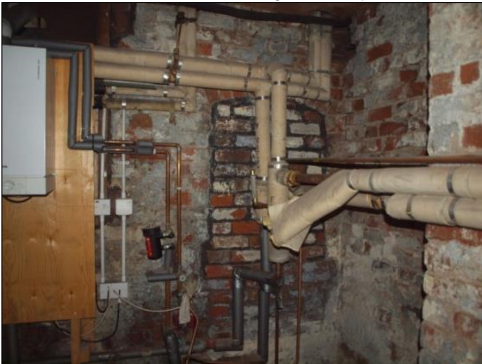
Plate 81: Eastern room of basement showing blocked opening
