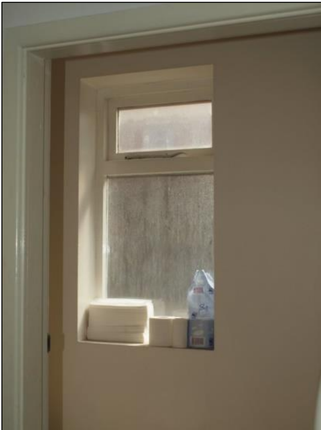
Plate 33: Detail of modern casement window to toilet
