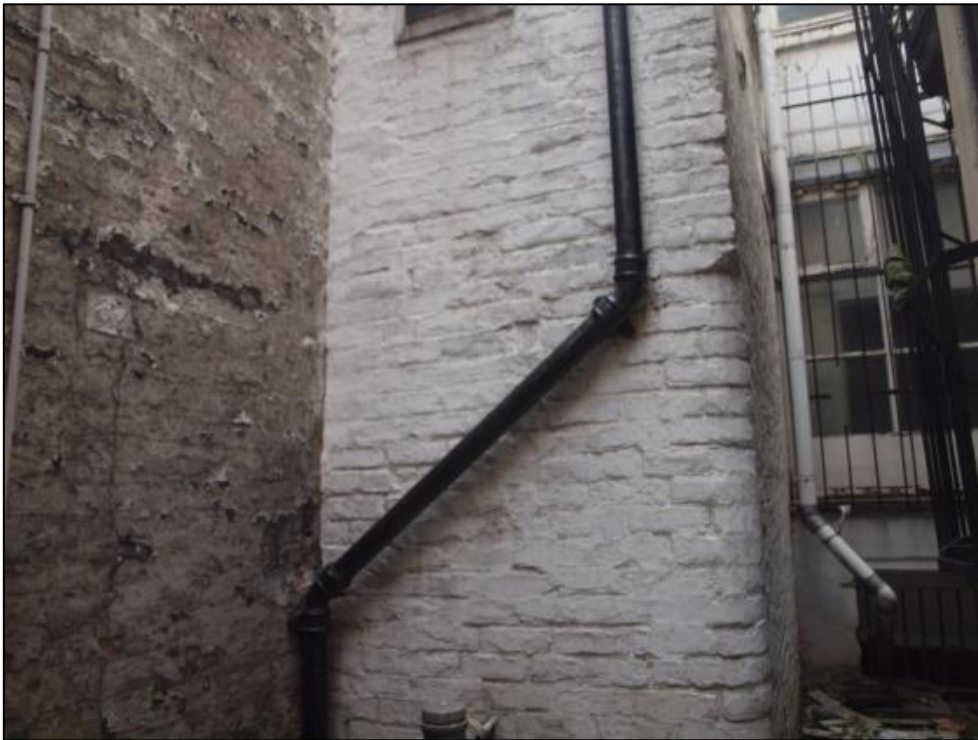
Plate 12: Whitewashed brick of northeast extension showing bull-nosed brick corner
