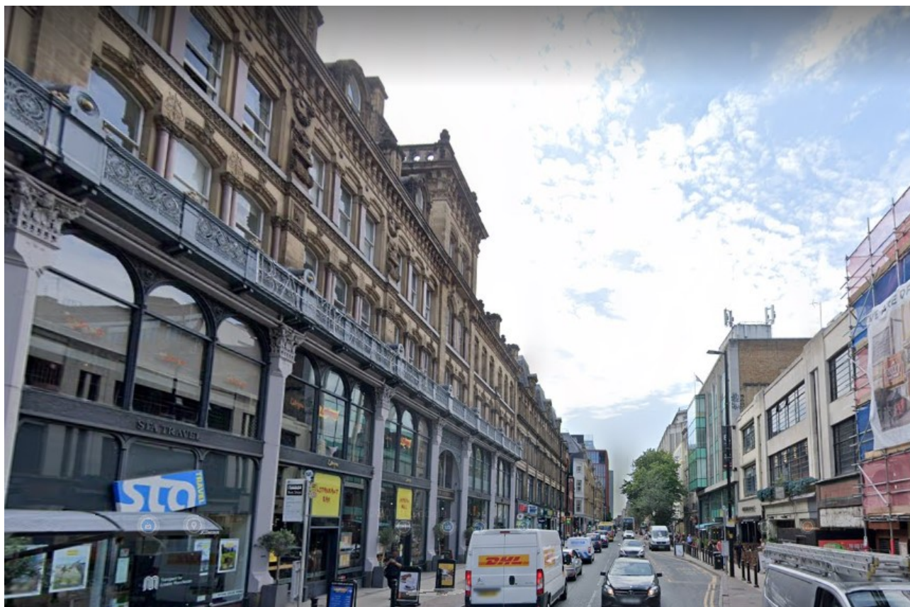
Figure 11: Image of Barton Arcade (left) demonstrating co-visibility with the application site (Source: Google Streetview)
