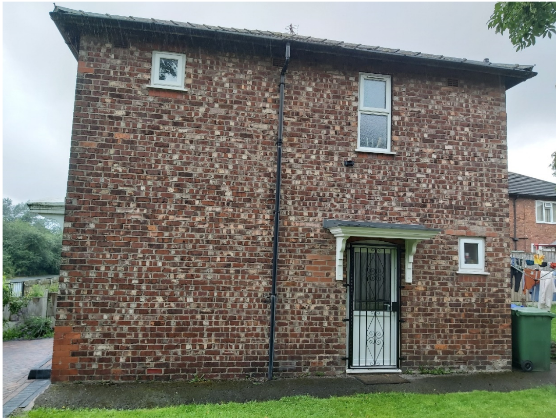
PHOTO: EXISTING SIDE VIEW
