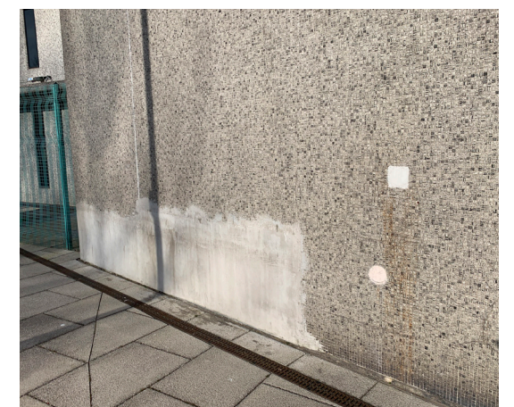
Replacement cladding panels to area of delamination
