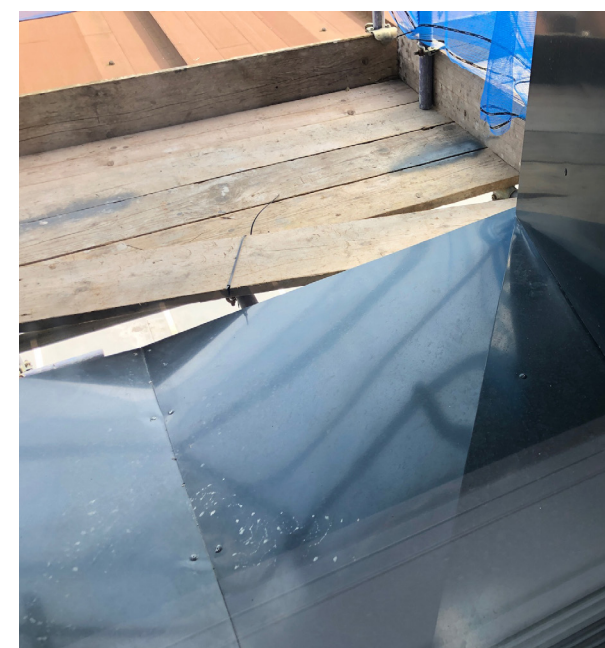
Overcladding in sheet metal (test) on site to 1 window: not a long term solution or cost effective sepcification / installaion method for the entire building
