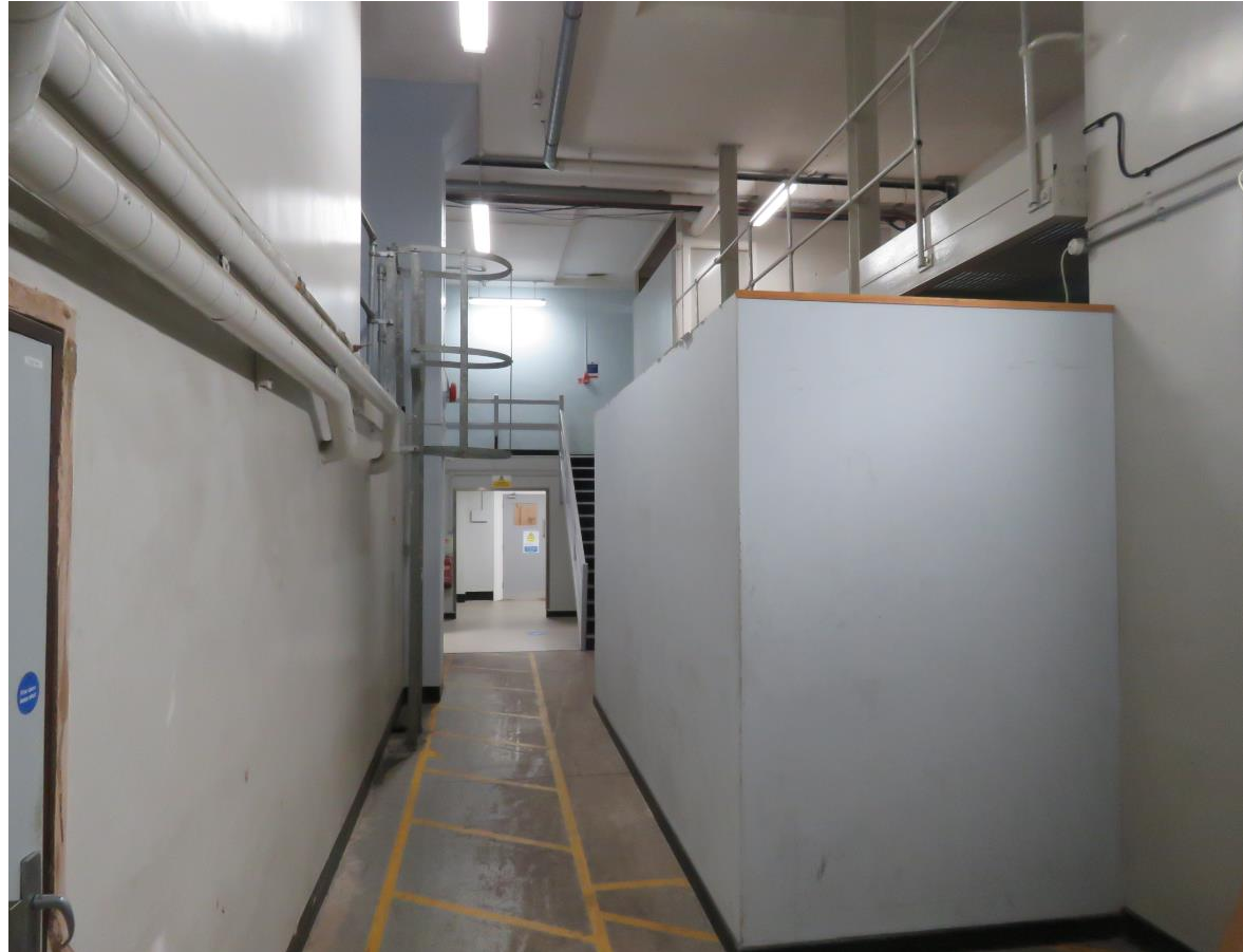
00-38 Looking north along the service corridor showing the mezzanine entrance to the car-park and building manager's office.
