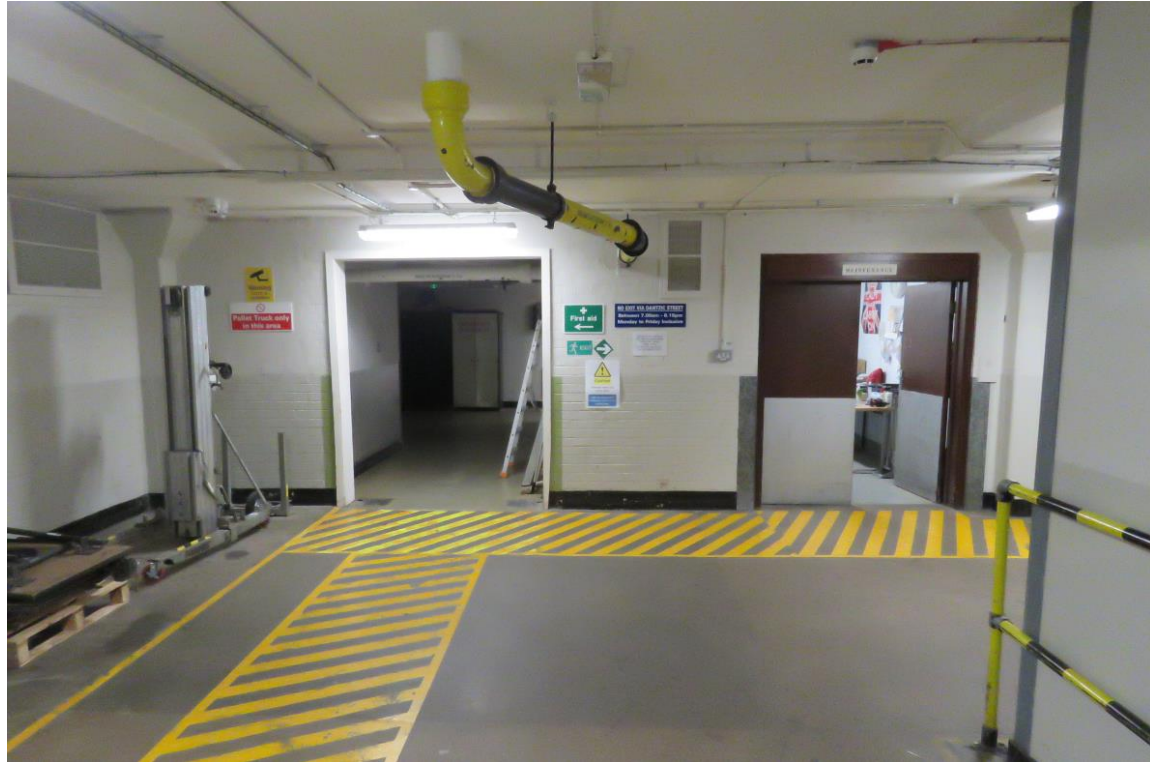
00-22 Looking south into the service area.
