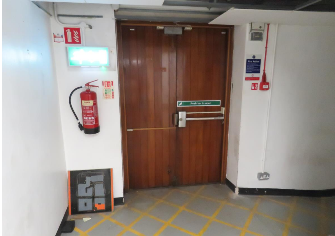
00-26 Looking south toward an emergency exit.
