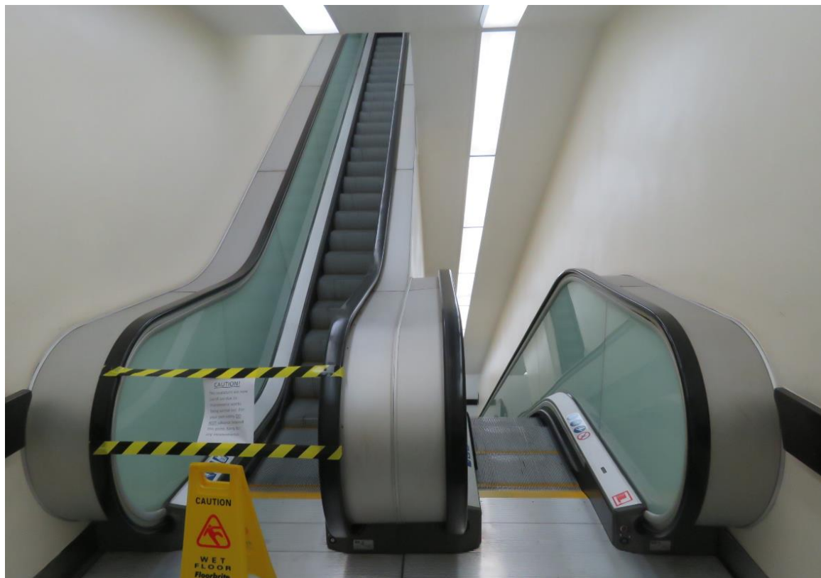
00-35 . View of the escalators. Looking north.
