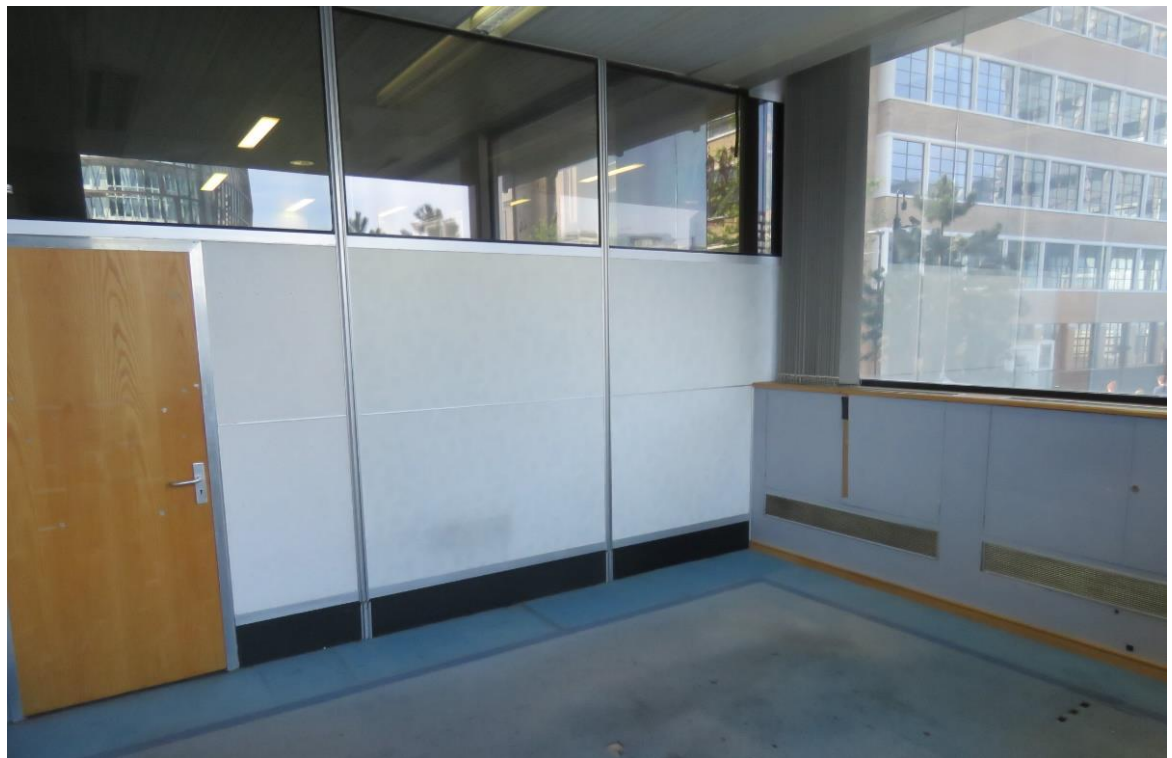
00-07 Looking south-east within the original corner office, showing the high-level Weathermaster.
