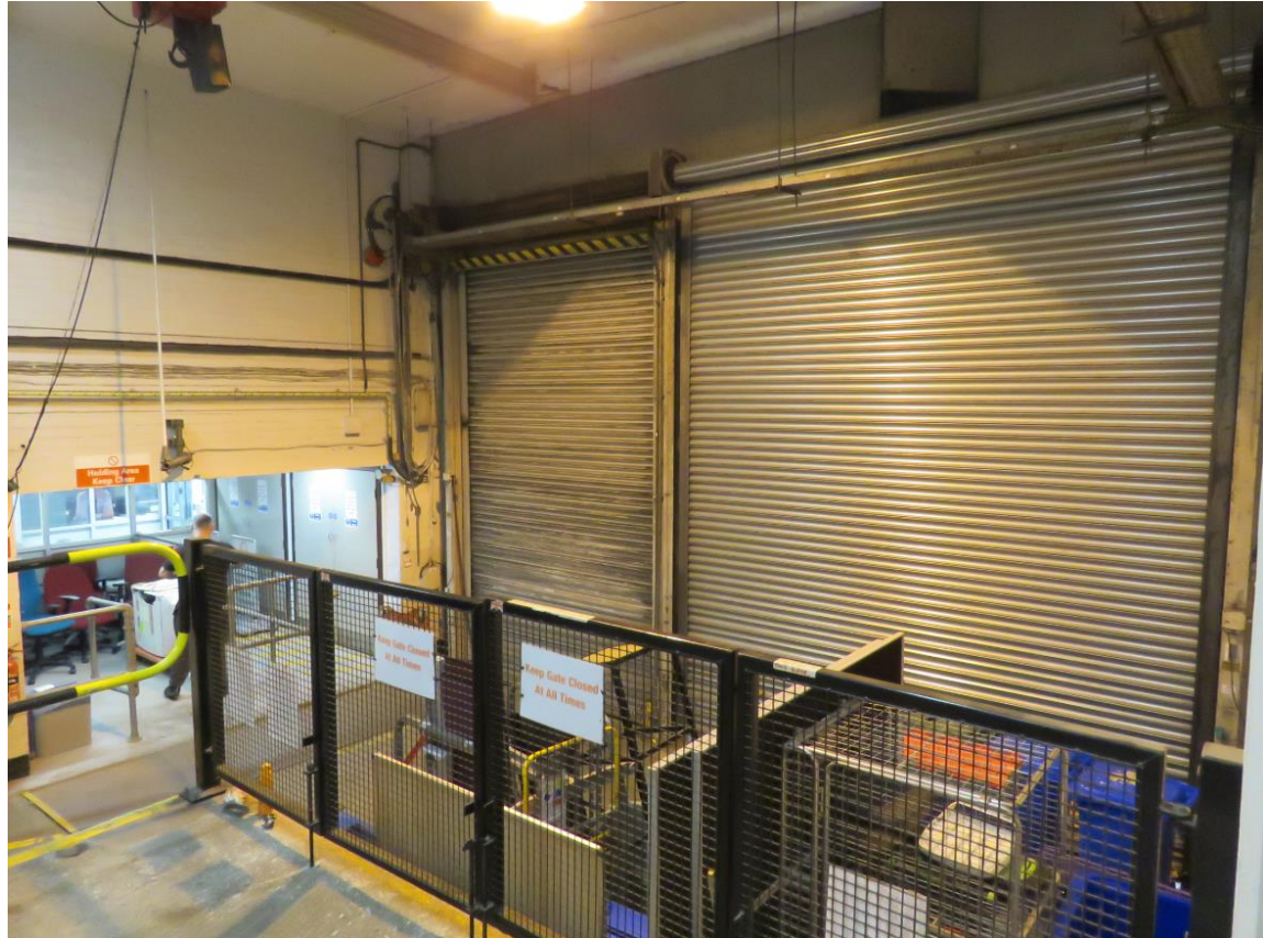
00-18 Looking south-west towards the Dantzig vehicle entrance.
