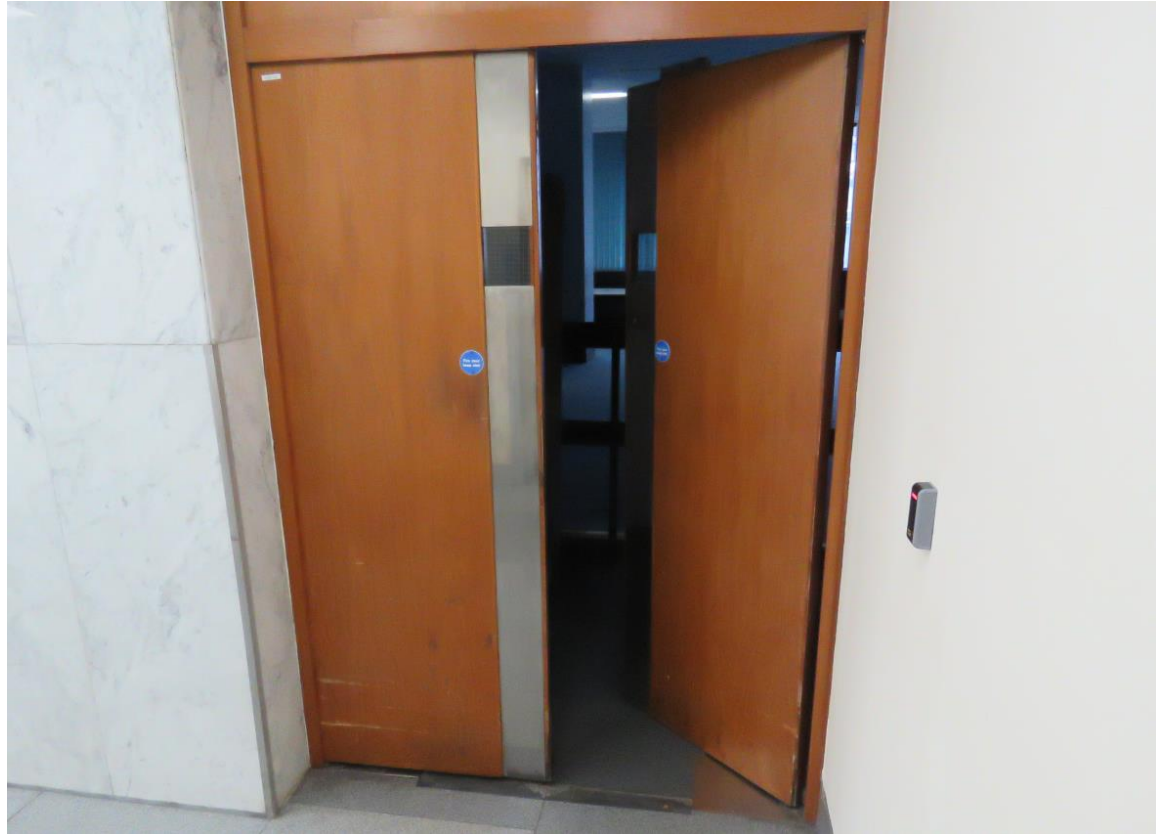
00-34 Entrance to the former branch office.
