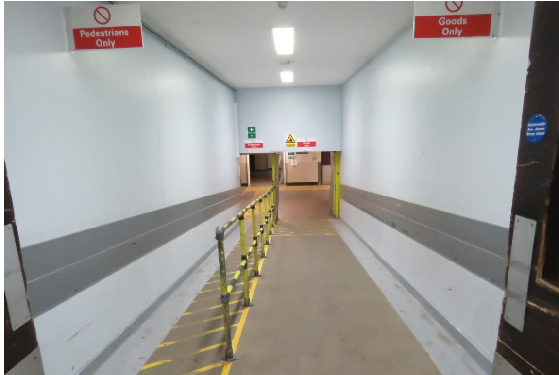
00-20 Looking south along the service corridor. Note the change in level.
