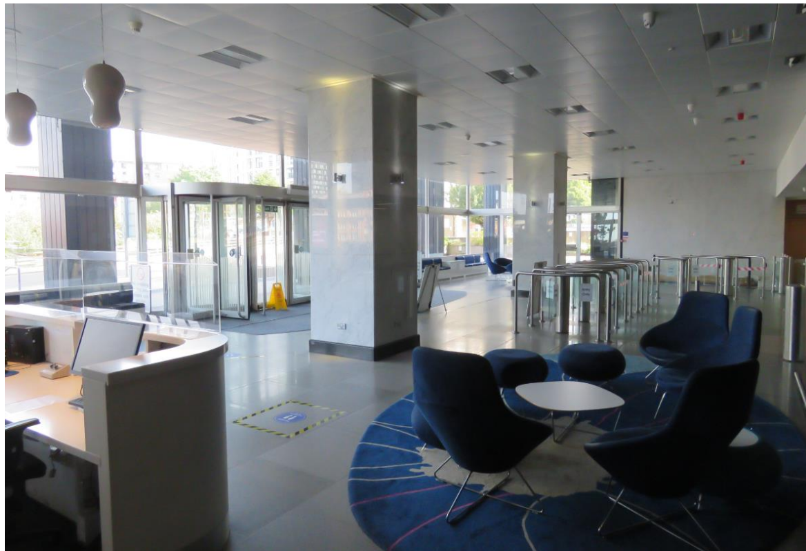
00-05 Looking north-east from the entrance to the post room showing the replacement ceiling.
