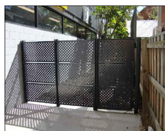
Perforated steel panel fencing 2.1m height, with 1.2m clear opening width lockable single gate to match. Galvanised steel with powder coated finish.
