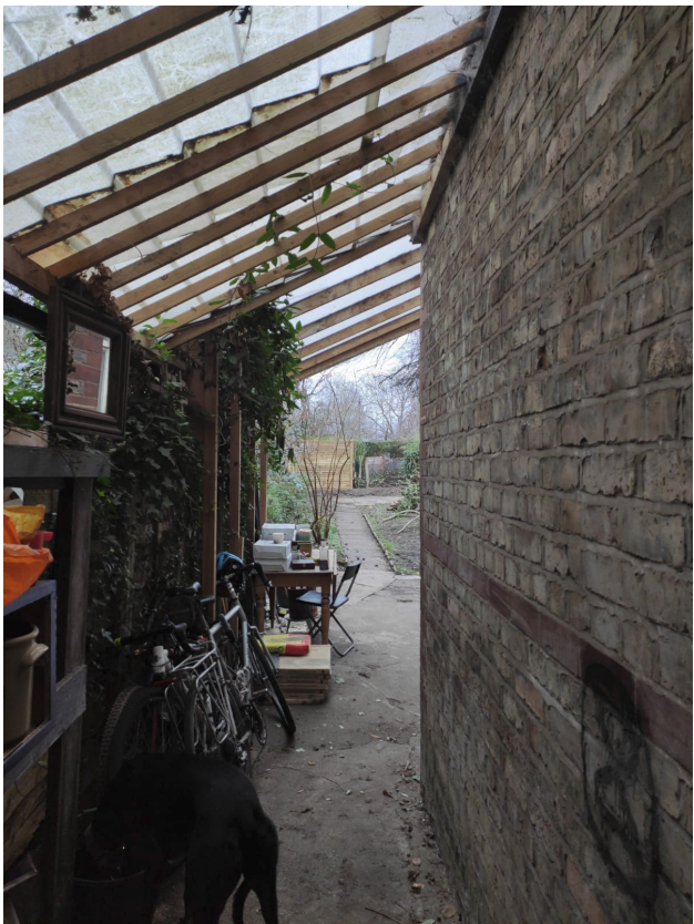
Fig 0.8 - View down side to the rear garden
