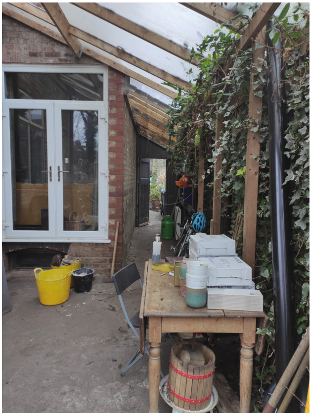
Fig 0.9 - View down side to front garden
