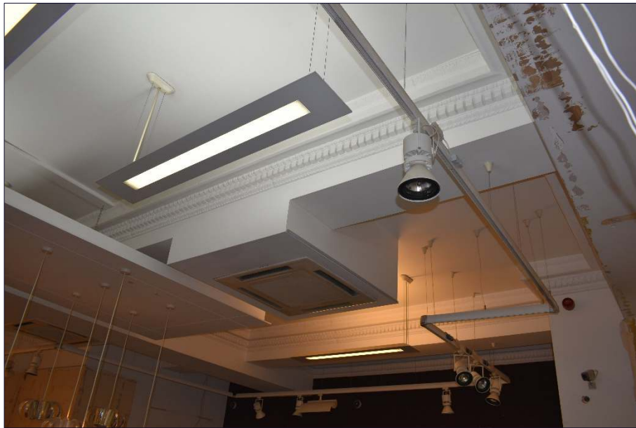
Plate 10: Ceiling detail of Unit 16-18, Royal Exchange Arcade
