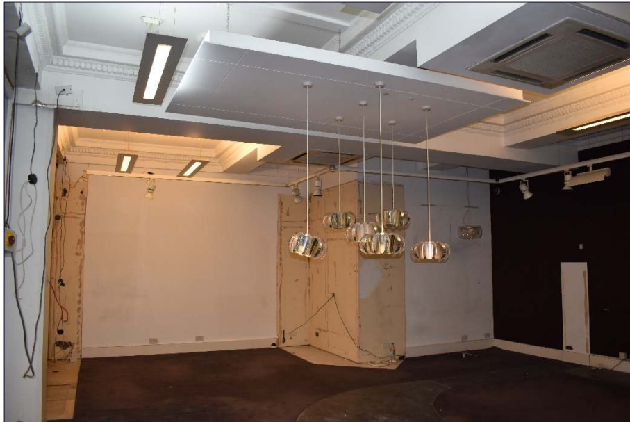
Plate 9: East wall of unit 16-18 Royal Exchange Arcade
