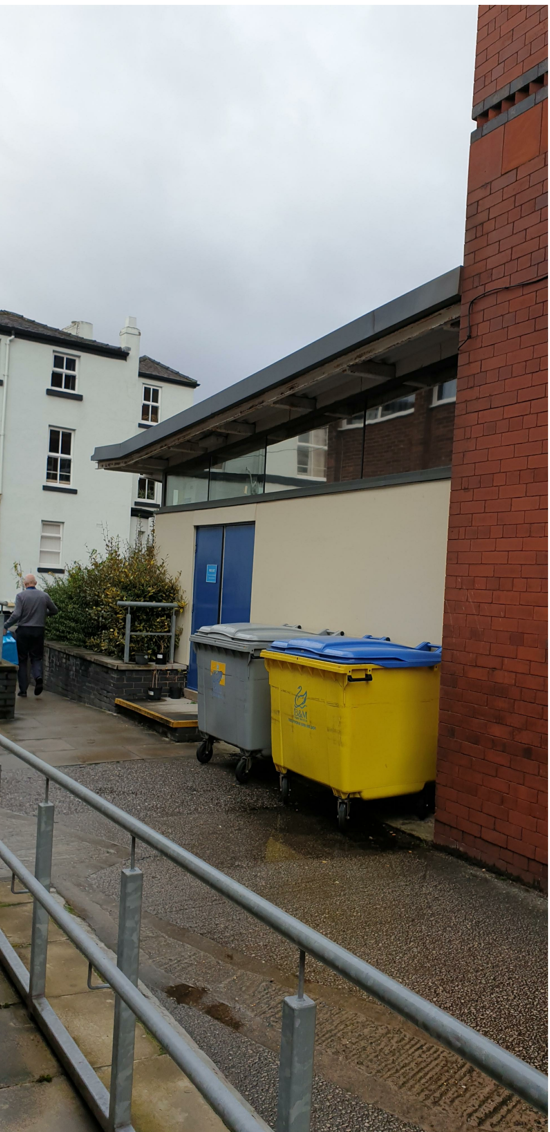
Image of existing south facing elevation;
