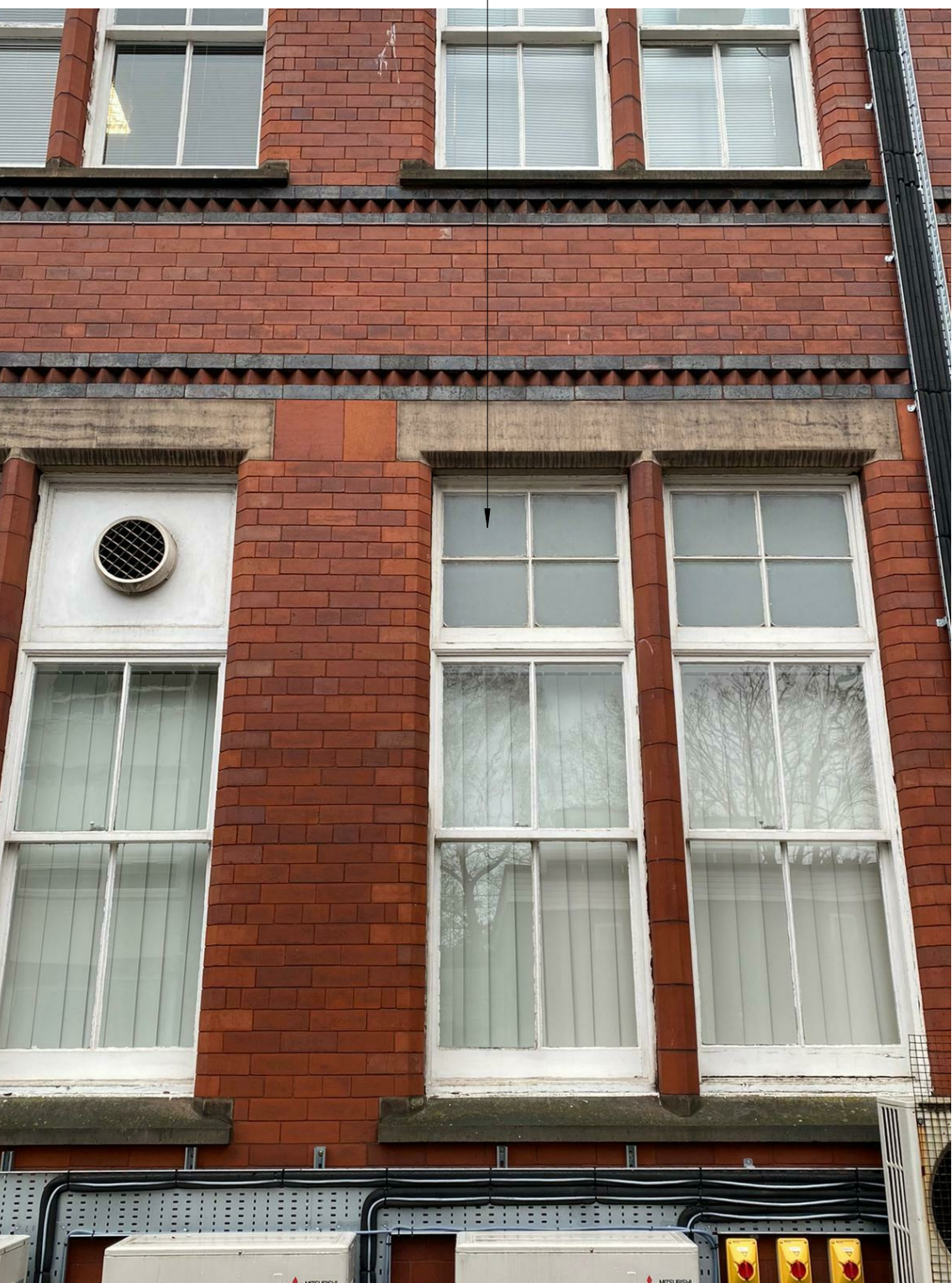
Image of existing south facing elevation, focussing on chamfered brick detail & stone lintel to be retained
