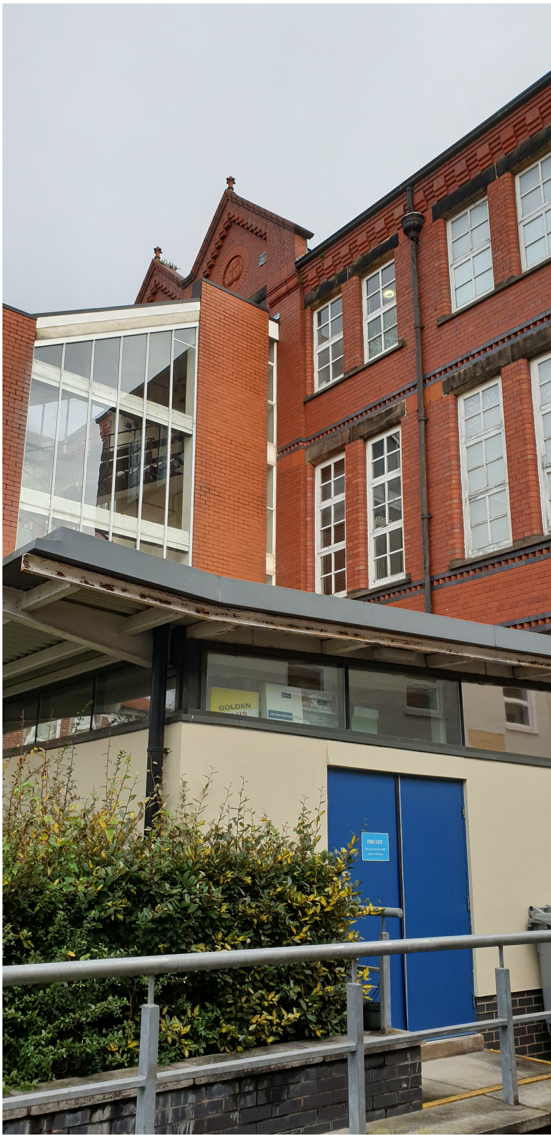
Image of existing south facing elevation
