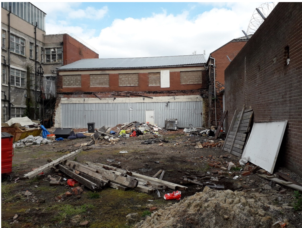
Figure 3 View of the site, looking north
