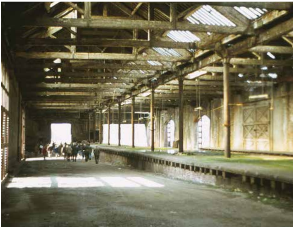
The Power Hall in 1978 prior to restoration
