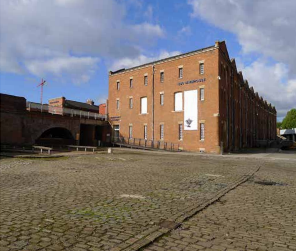
2. Exterior view of the 1830 Warehouse, looking West
