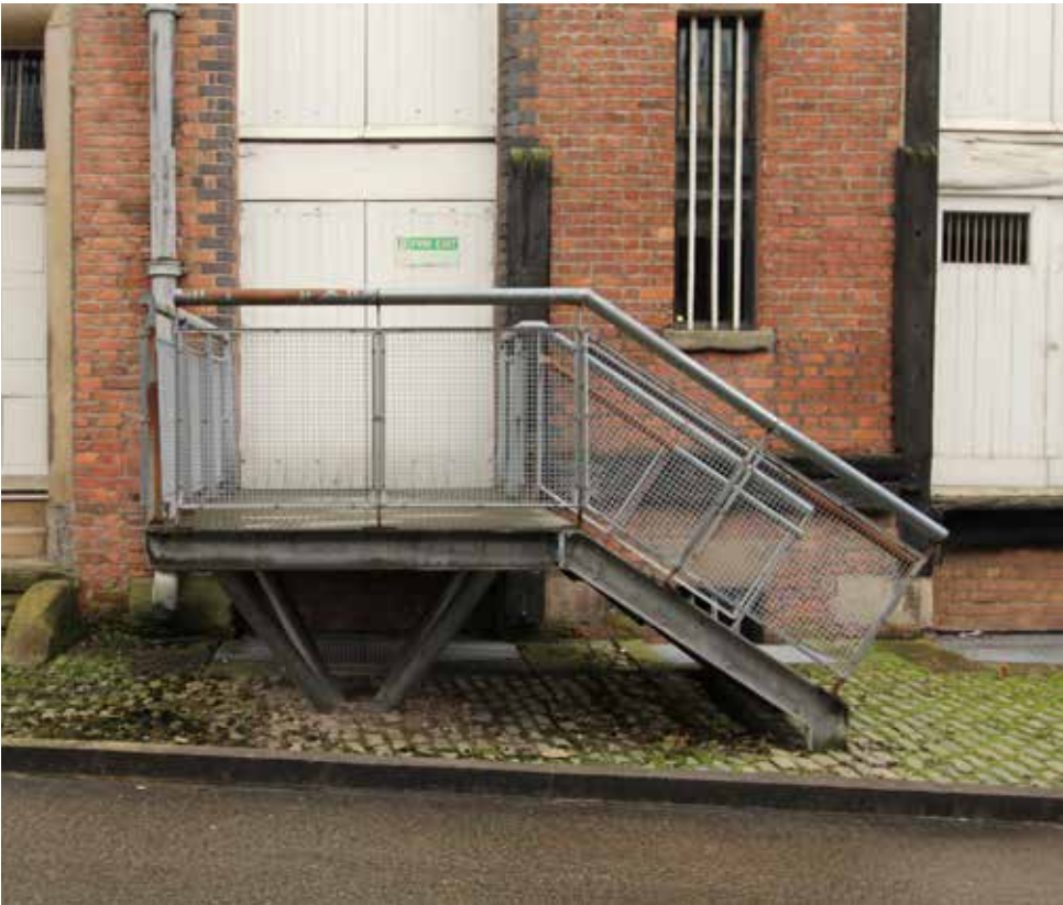
4. Exterior detail view of the 1830 Warehouse Bay 2
