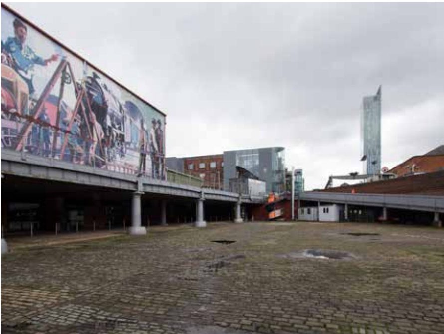
View of the ramp connection Lower and Upper Yard
