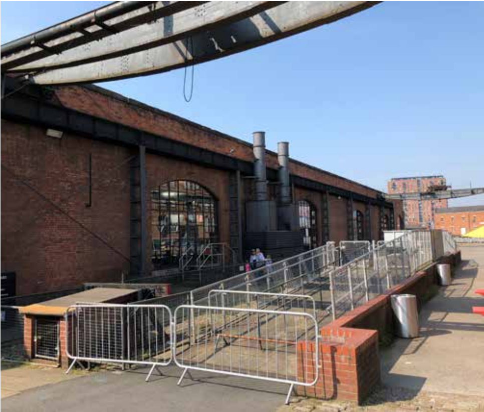
2. Exterior view of the Power Hall at the East end, looking towards the platform
