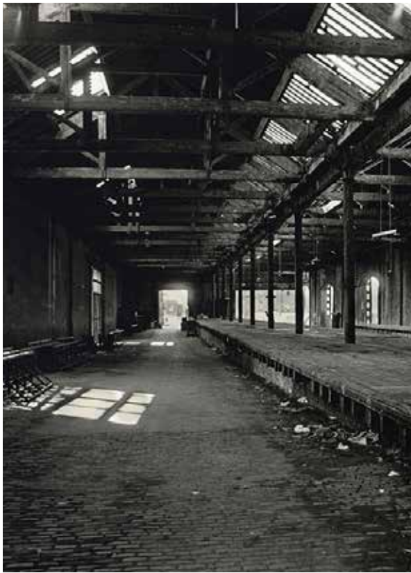
The Power Hall prior to restoration
