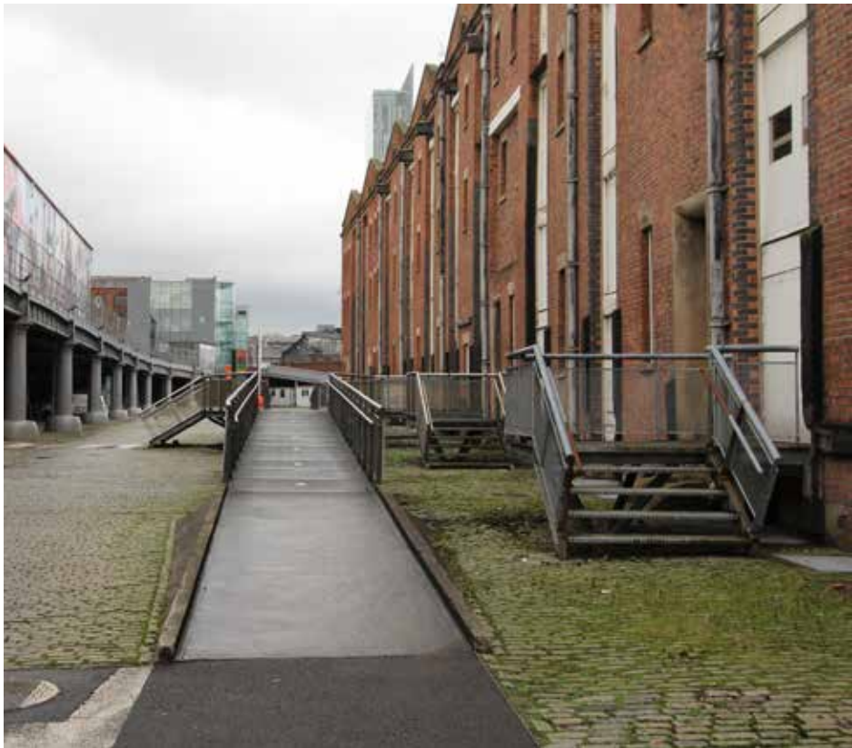
3. Exterior view of the 1830 Warehouse at the West end, looking East
