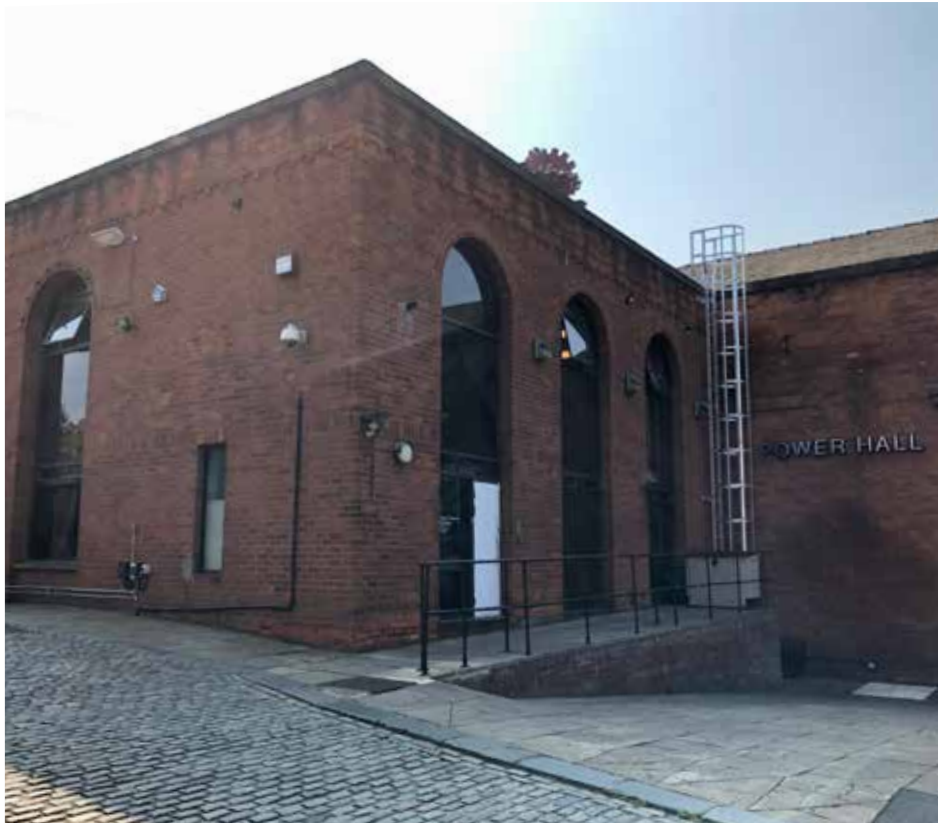
1. Exterior view of the Power Hall at the Eastern end, next to the entrance
