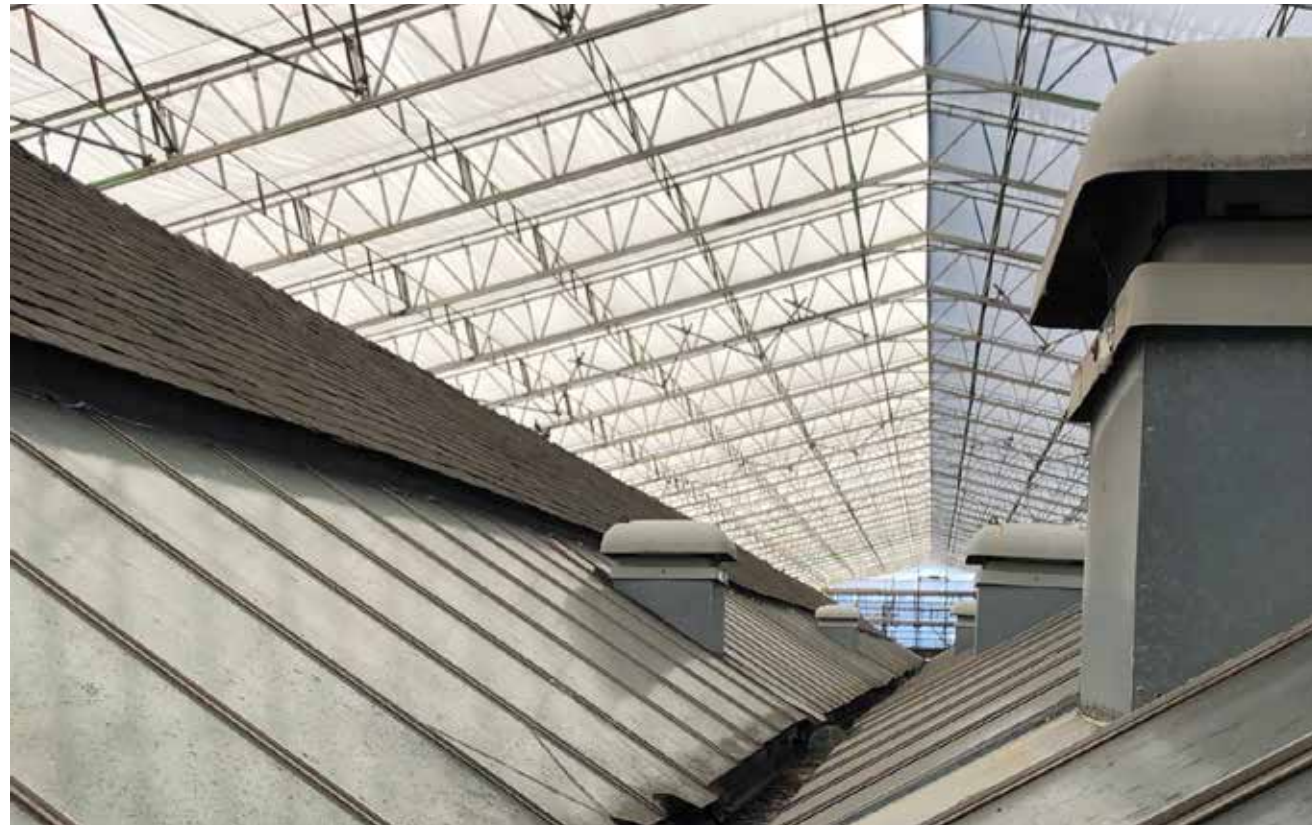
View of the central valley roof and scaffold enclosure
