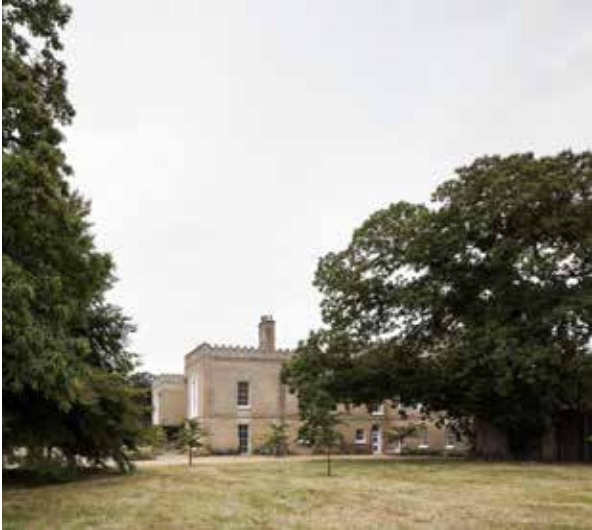
Refurbishment of a Grade I listed artist's house, Norfolk
