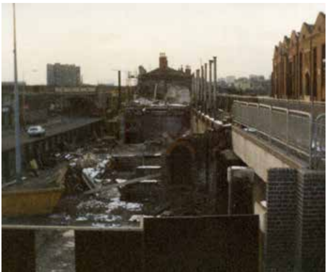
Photograph of the Station being rebuilt 1986
