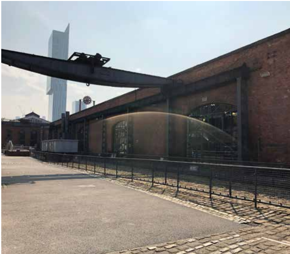
3. Exterior view of the Power Hall at the West end, looking East
