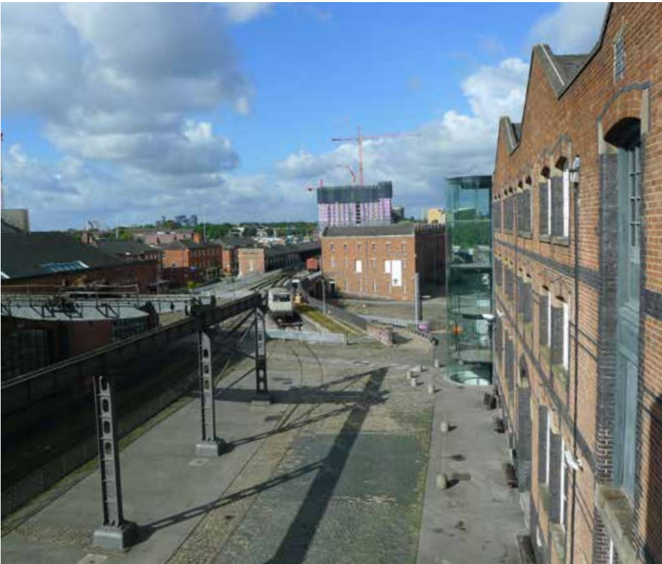
4. View of the Upper Yard looking West, towards the lower yard
