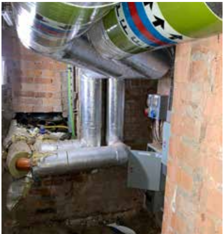
1 Existing pipework entering 1830 Warehouse
