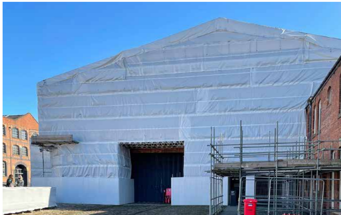
View of the Power Hall exterior with scaffold enclosure
