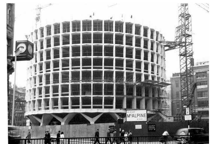
Space House during construction
