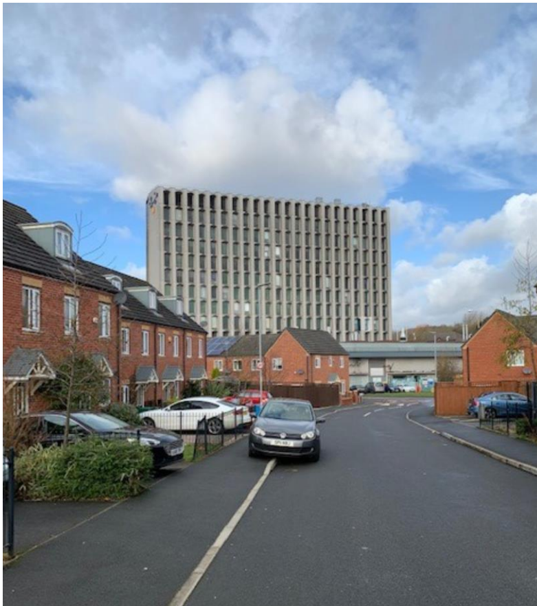
Figure 3.1 Hexagon Tower from Bottomley Side
