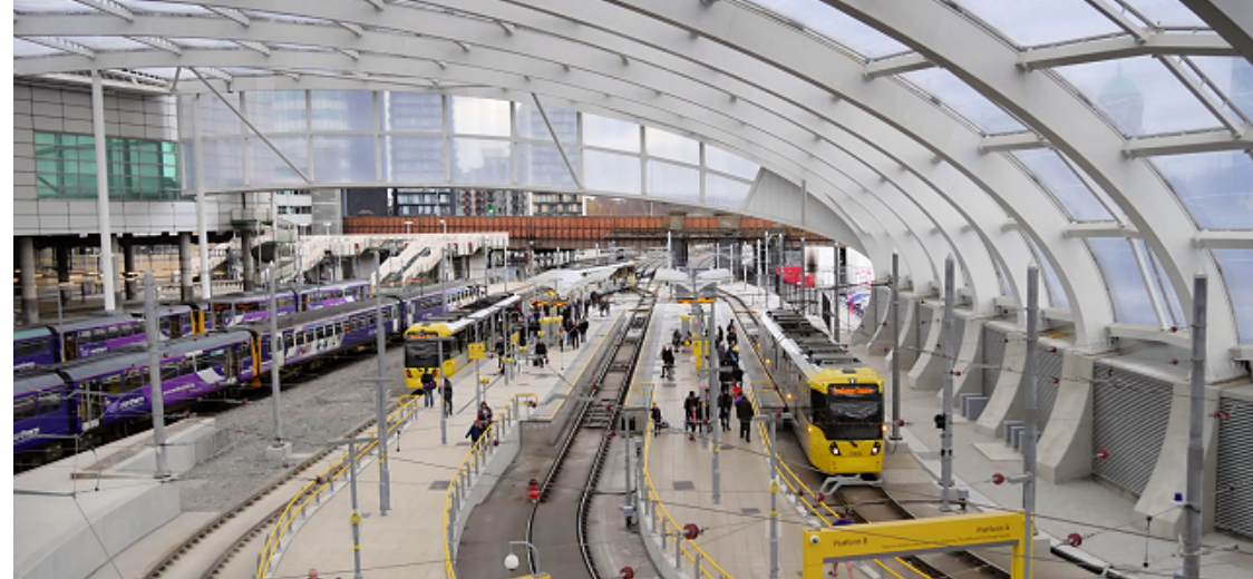
Victoria Station - Trains
