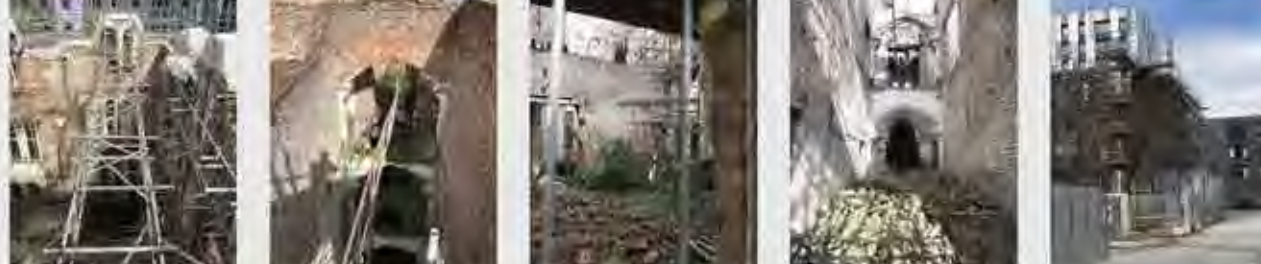
Photograph showing building condition.
