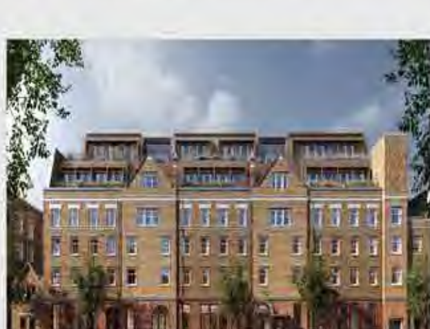
Photograph showing building condition.
