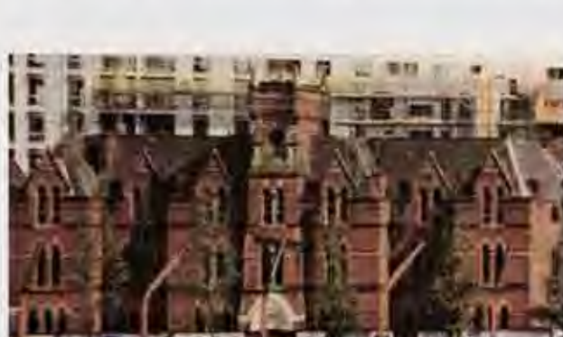
Photograph showing building prior to demolition work.
