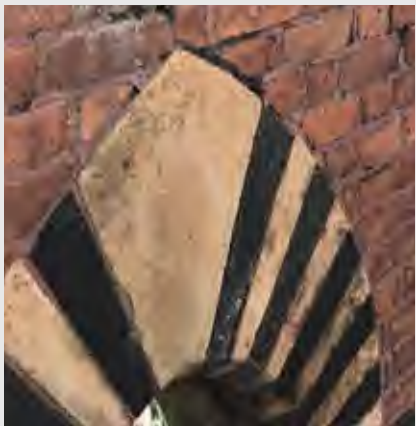
Arched Lintels to match existing
