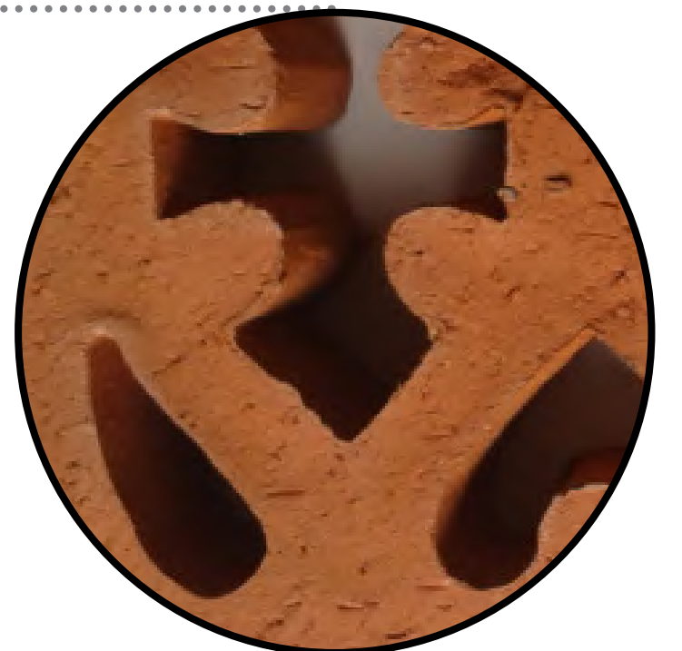
Terracotta air vents shape and colour to match frieze
