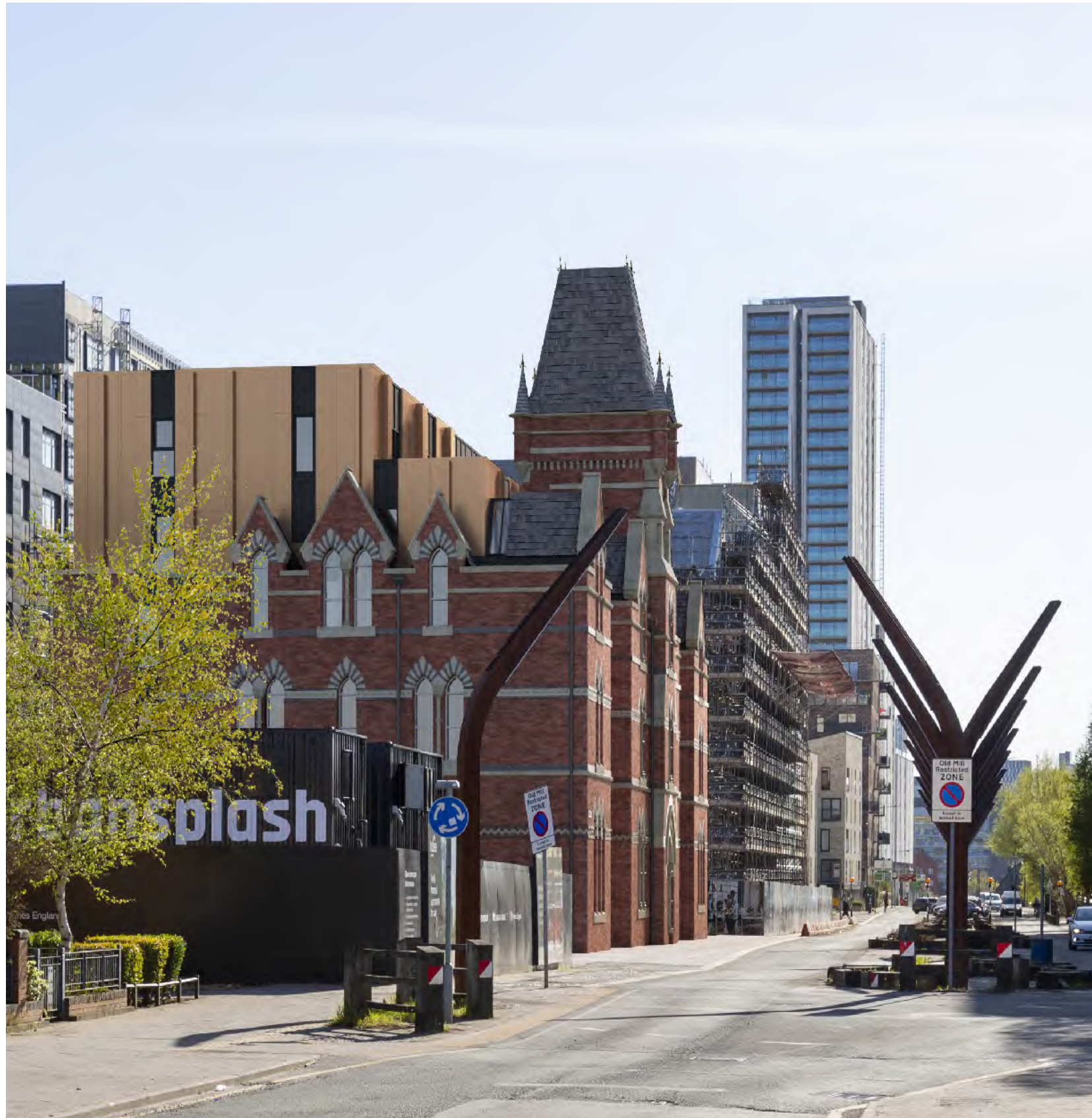
View looking at North East Elevation from Old Mill Street
