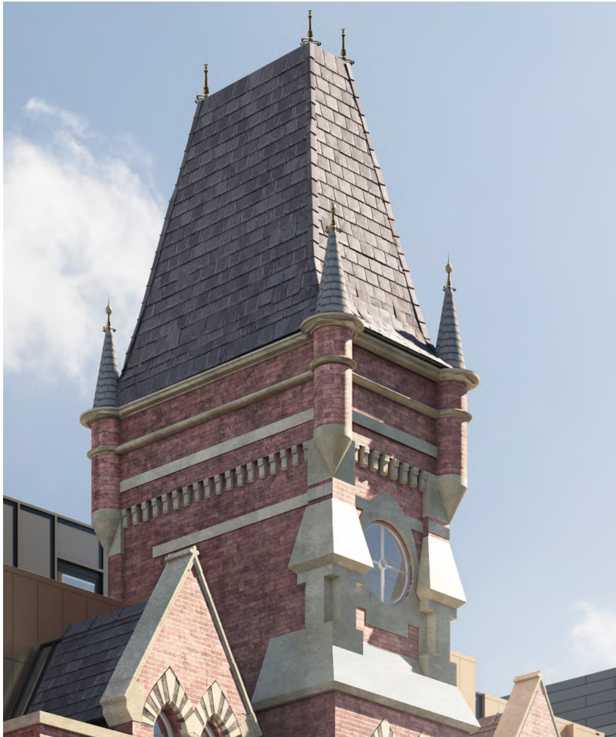
Front View-brick & detailing to be replaced / matched
