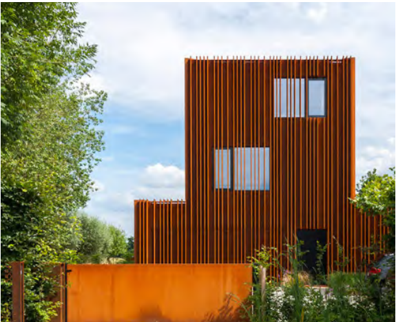
The Corten House, Konitech, Belgium
