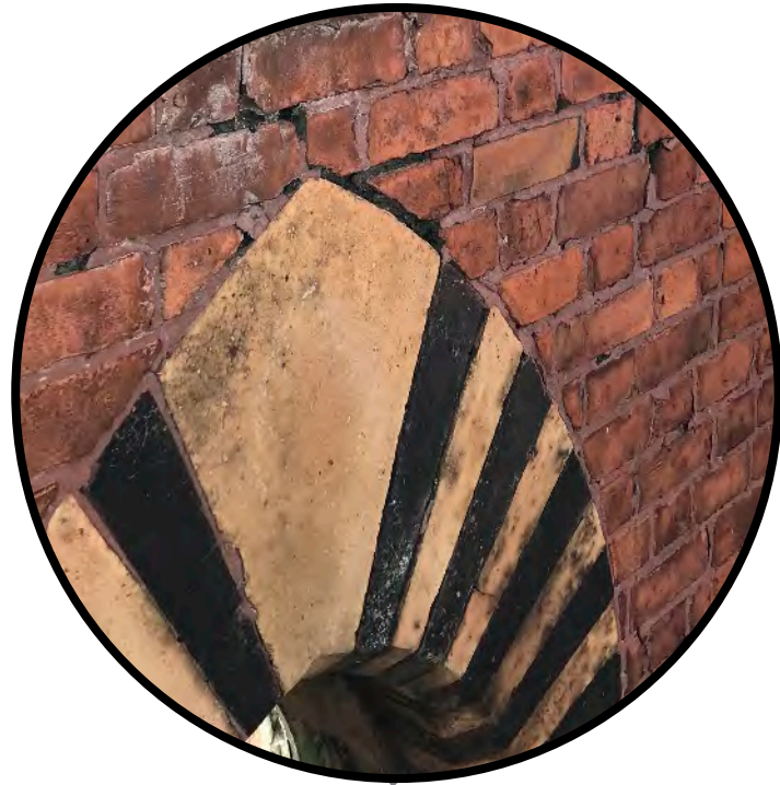
Arched Lintels to match existing
