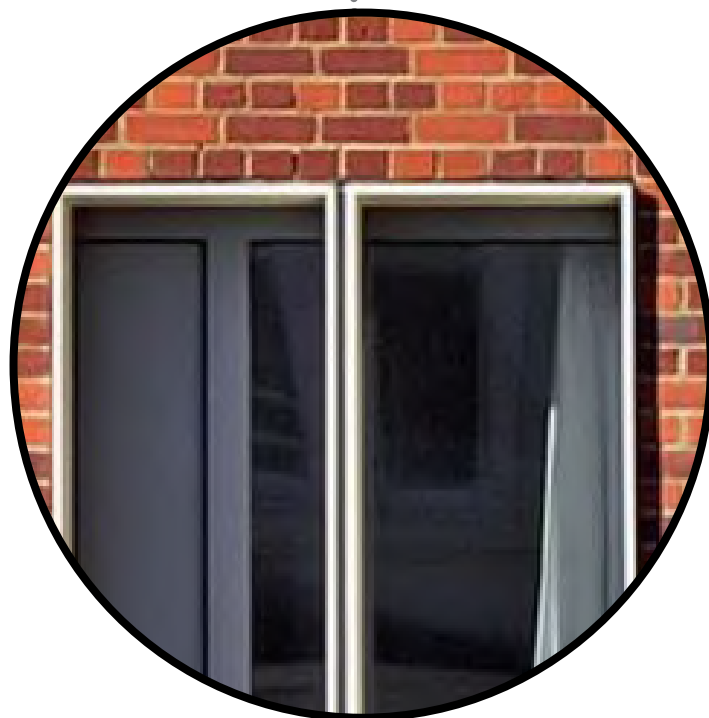
Powder coated aluminium window frame
