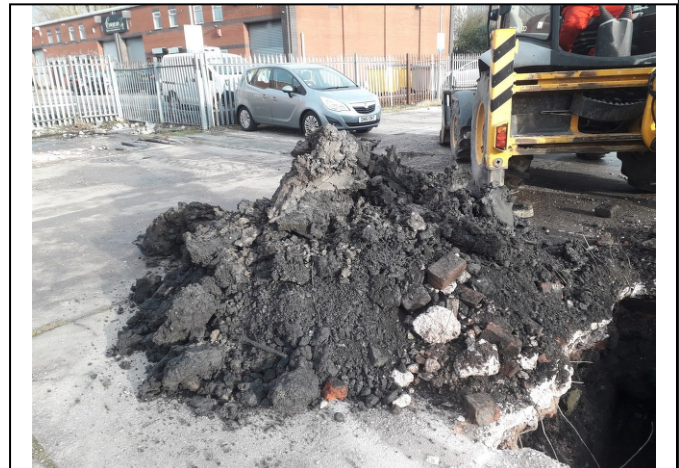
Trial Pit 109 Spoil
