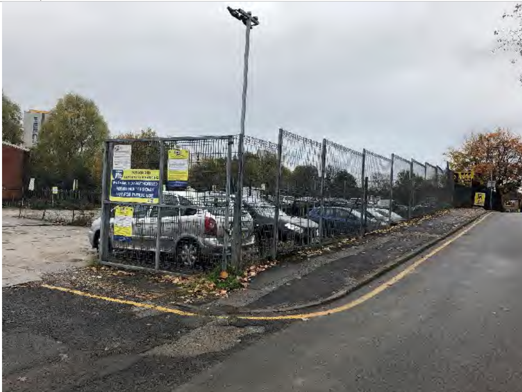
PLATE 2 VIEW TOWARDS SOUTH EAST CORNER (LEVEL CHANGE OVER BRIDGE STRUCTURE)
