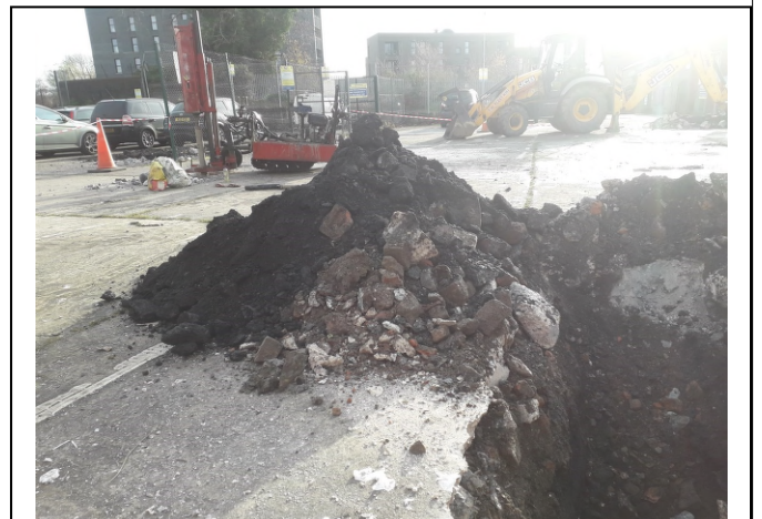
Trial Pit 110 Spoil
