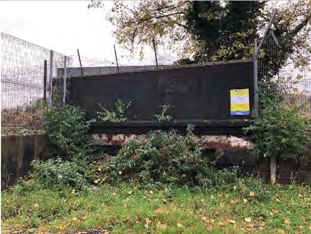
PLATE 5 BRIDGE STRUCTURE UNDER JERSEY STREET
