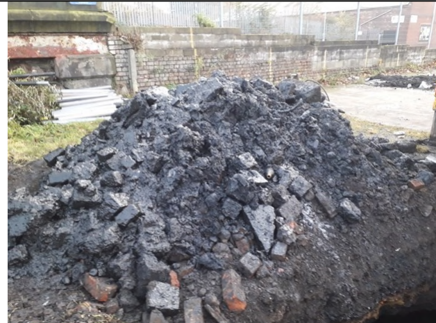
Trial Trench 103 B Spoil
