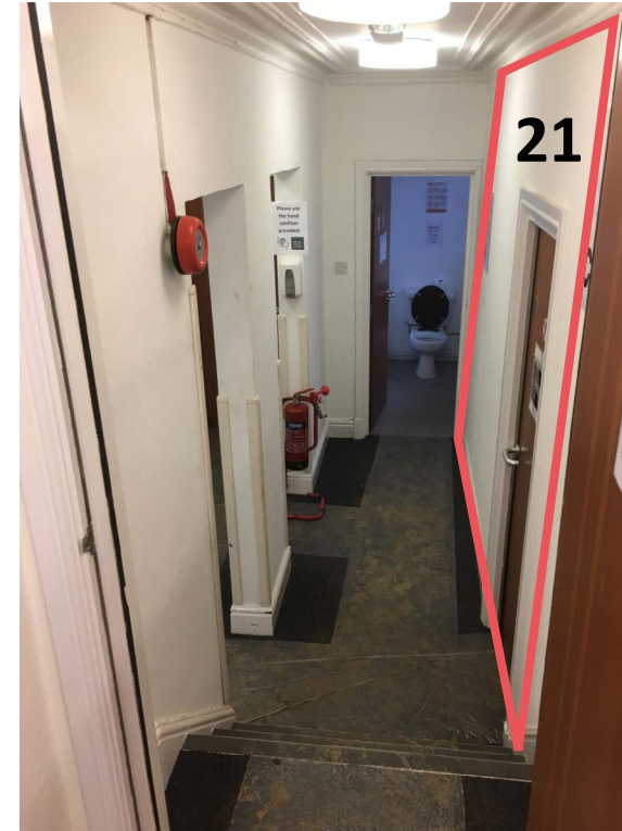
Views from first floor - hallway
