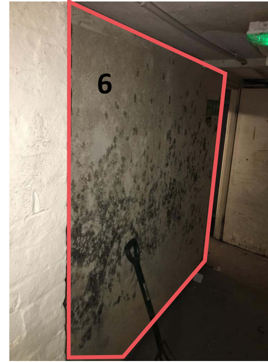
Staircase brick wall- View numbers 6
