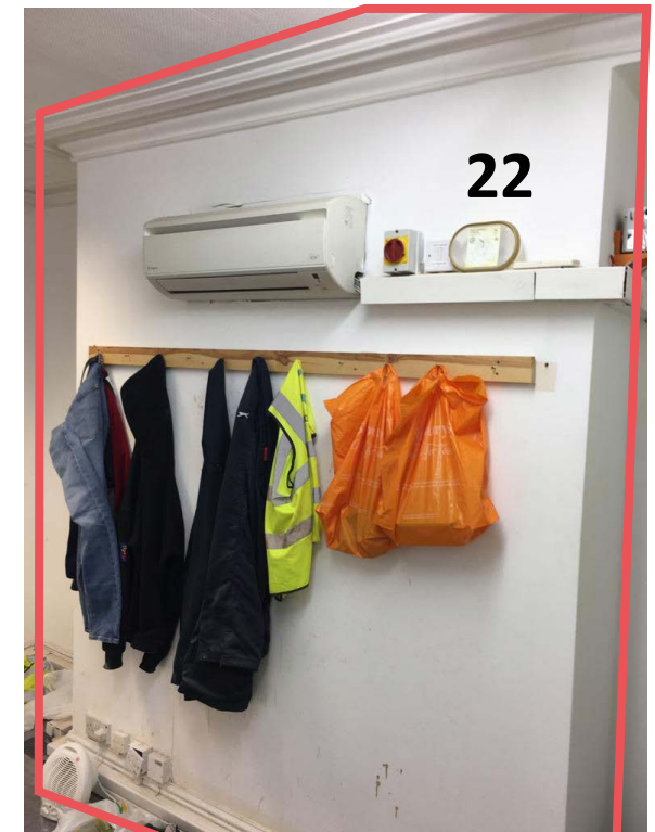
Views from first floor - Chimney breast to be demolished to enlarge bedroom
