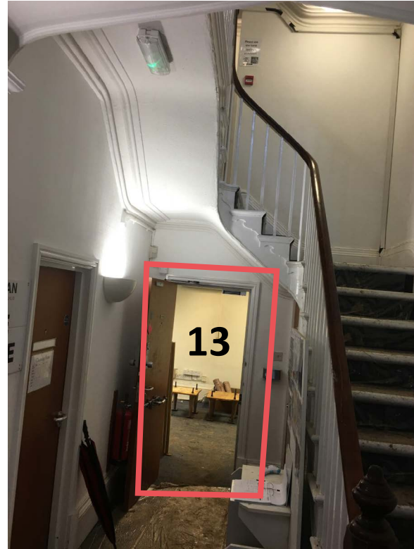
Door to be blocked - View 13
