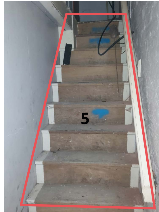
Staircase to be dismantled View numbers 5
