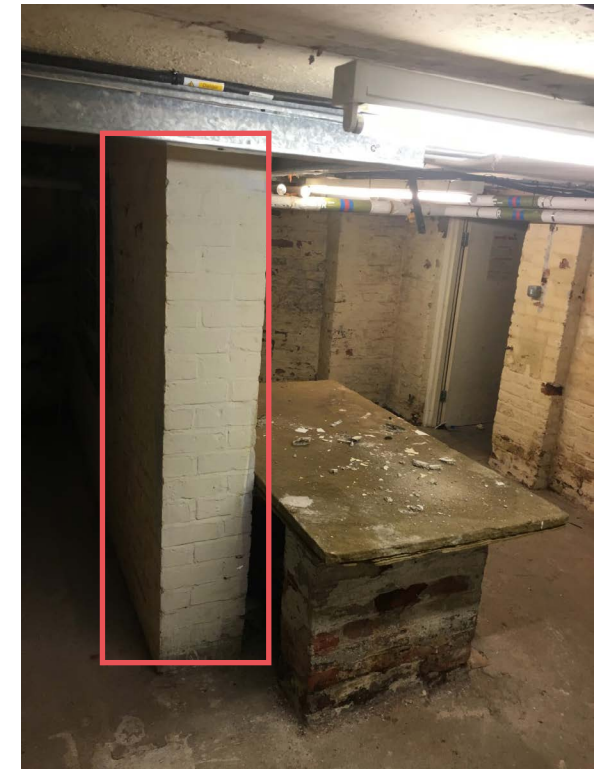
Views from room 2 - Stone worktop to be removed and kept in a safe area.
