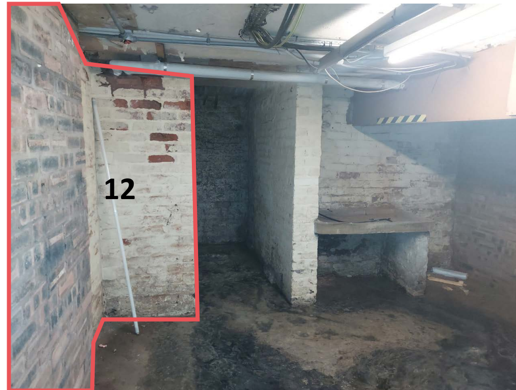
View 12 - Brick wall to be demolished - Stoned sink to be retained
