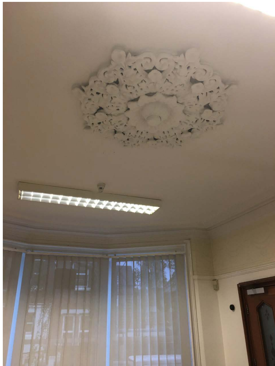
Views from room 5- ceiling rose
