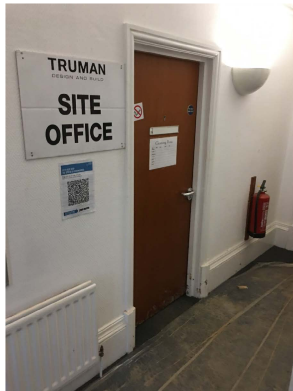
Views from ground floor lobby - Doorway, skirting and architrave to be retained
