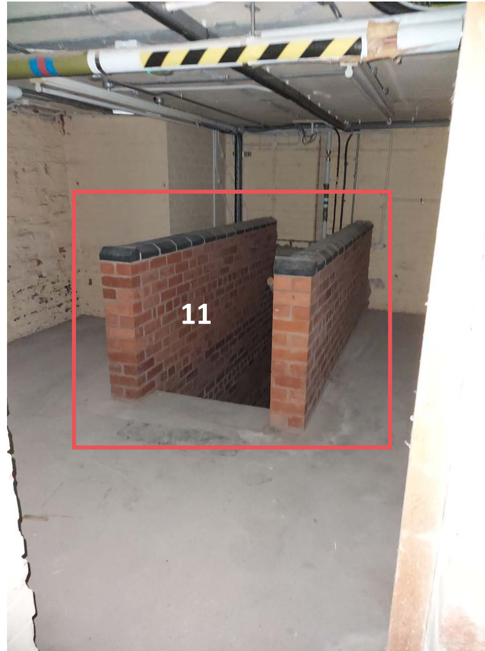
Staircase to be sealed - View 11
