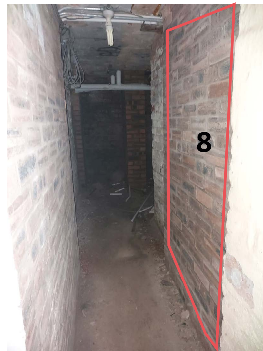
Corridor wall to be demolished, View numbers 8
