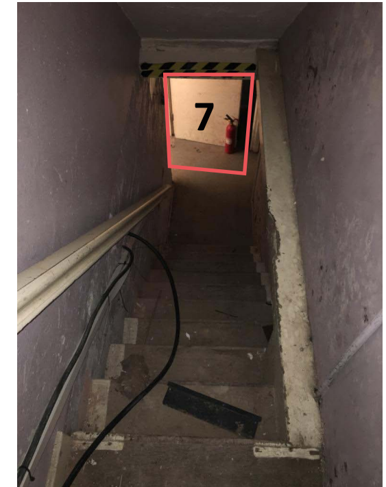
brick wall to be demolished- View numbers 7
