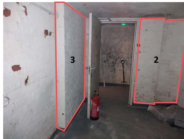
Walls to be demolished - View numbers 2 and 3
