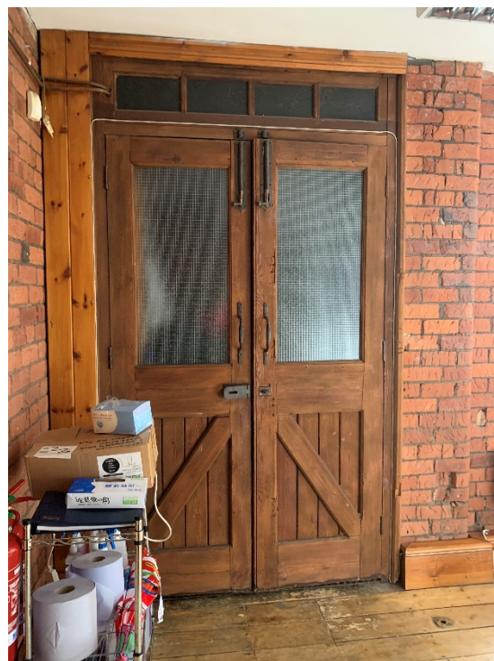
Figure 13: The original hoist doors to the south-east corner.
