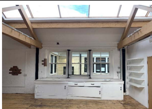
Figure 15: Looking north towards the internal atrium illustrating modern cupboards below the window.
