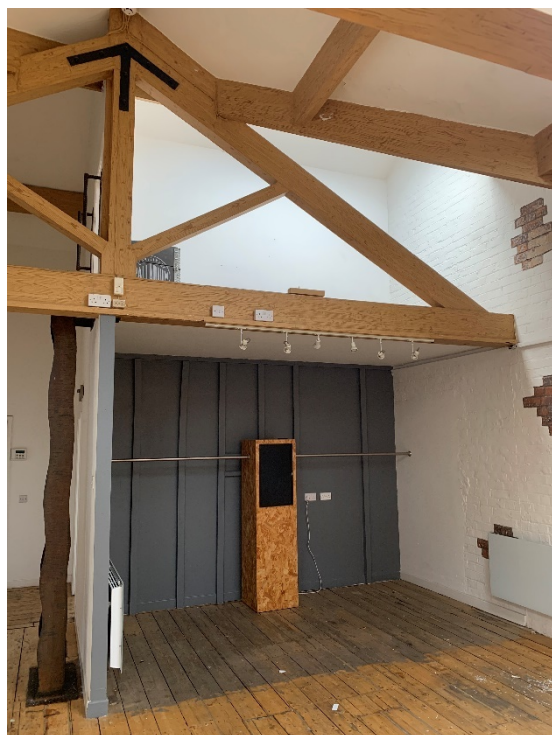
Figure 17: Beneath the modern mezzanine illustrating the underside of the modern mezzanine.
