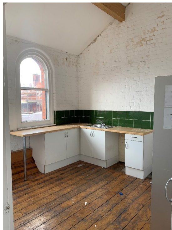
Figure 18: The modern kitchen fit-out to the north-west corner of the unit.
