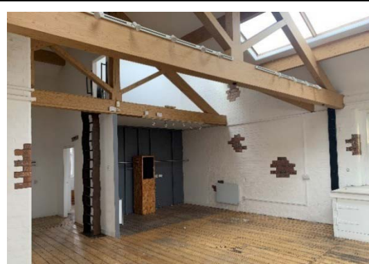
Figure 16: Looking west towards the modern mezzanine illustrating the exposed original roof structure..
