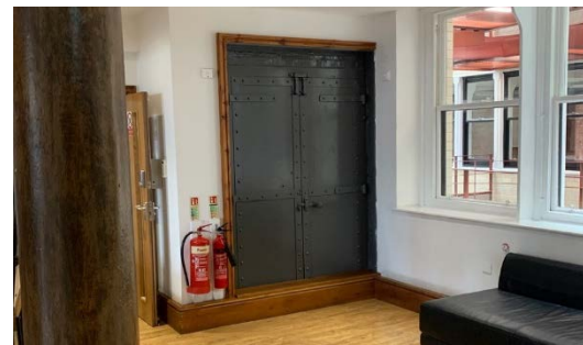
Figure 8: The original metal hoist doors to the south-west corner of the western unit.
