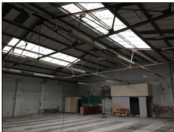
Plate 6 Interior of building
